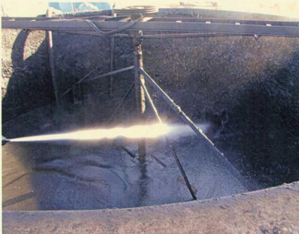
*No. 14 – Using the hot oil truck to jet fluid in the fiberglass tank.*
