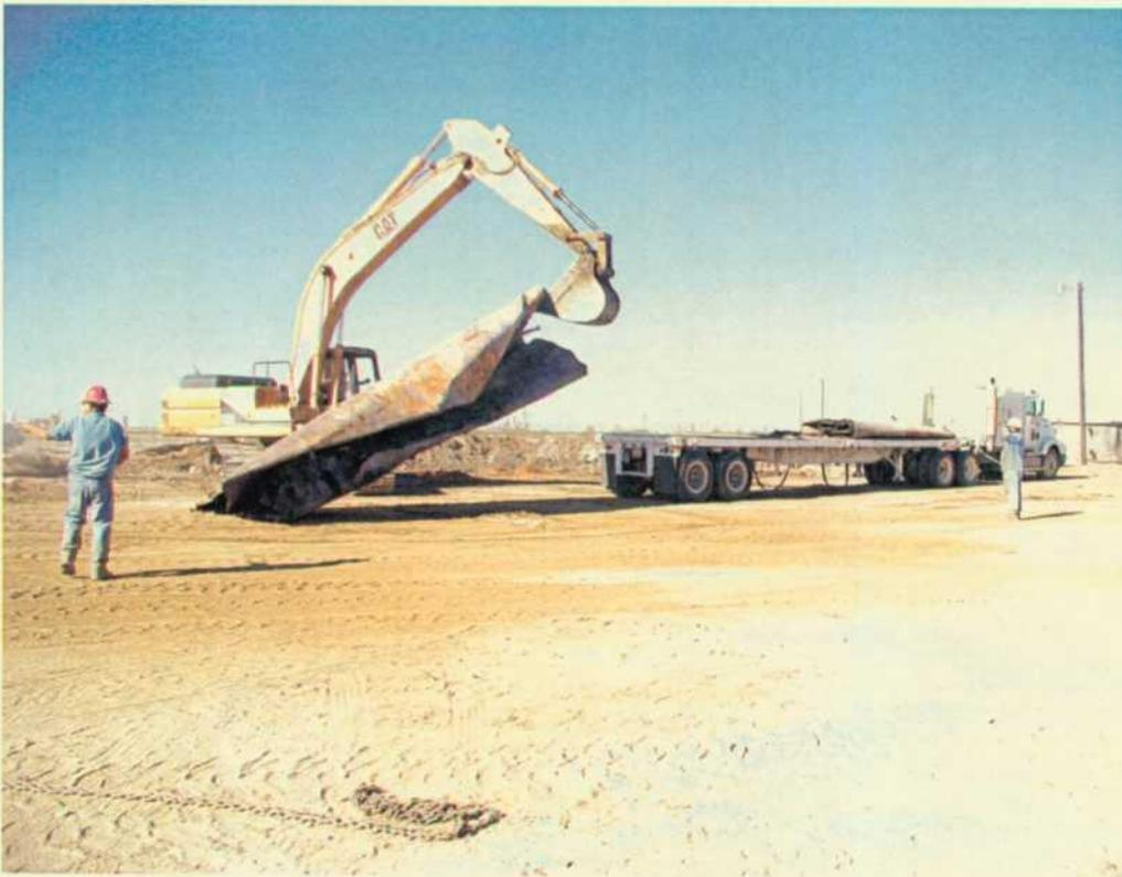
*No. 28 – Loading the smashed tank # 3 on flatbed trailer.*
