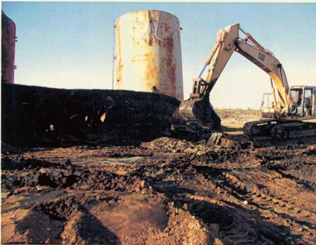
*No. 26 – Using track hoe to remove walls of 3000 bbl tank.*
