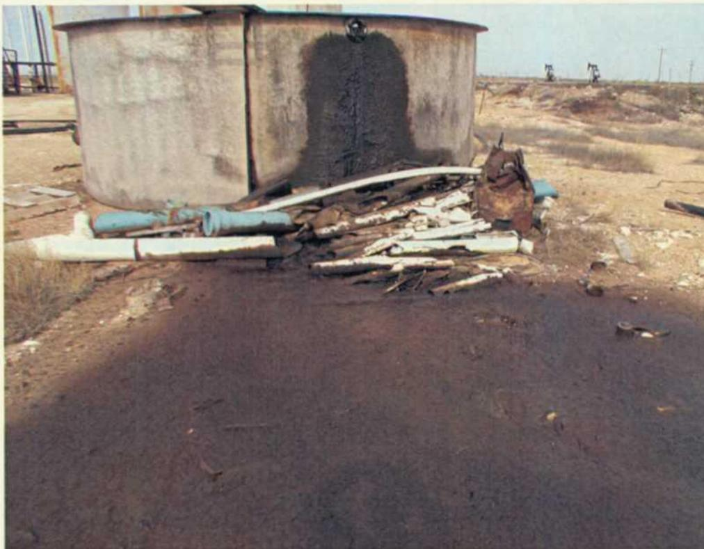
*No. 6 – Heavily stained soil at tank #6 and pvc piping.*
