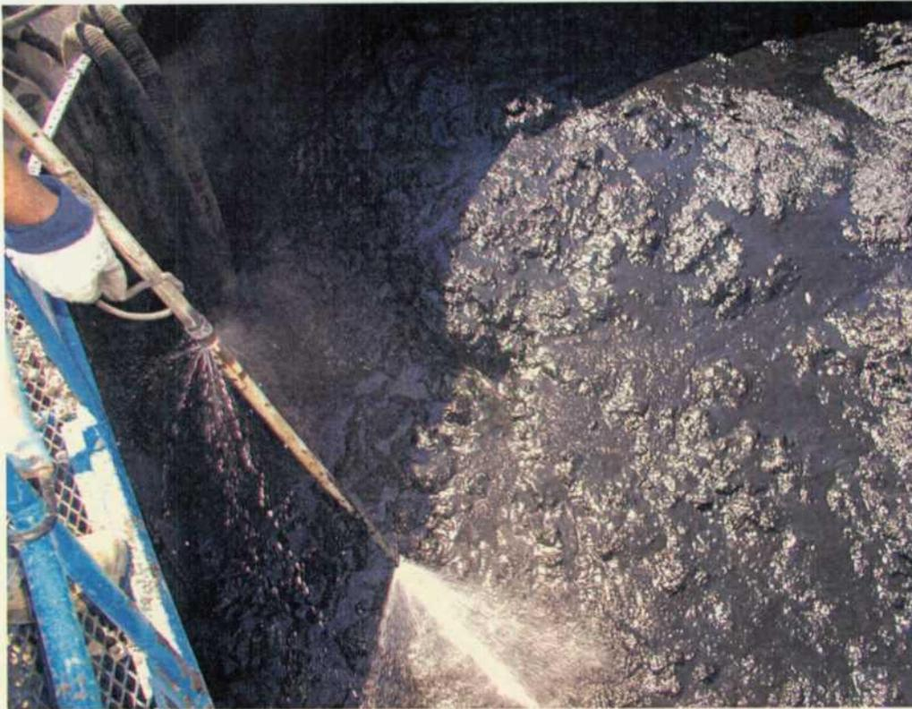
*No. 19 – Jetting and removal of fluid from 3000 bbl tank.*
