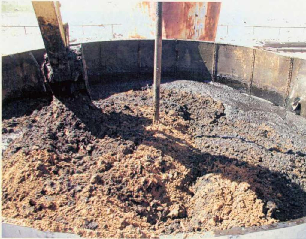
*No. 25 – Mixing of the thick fluid with sand.*
