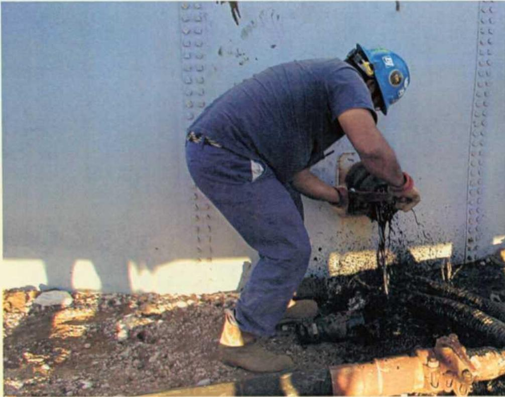
*No. 15 – Removing trash including a bird from the valve of the 3000 bbl tank.*
