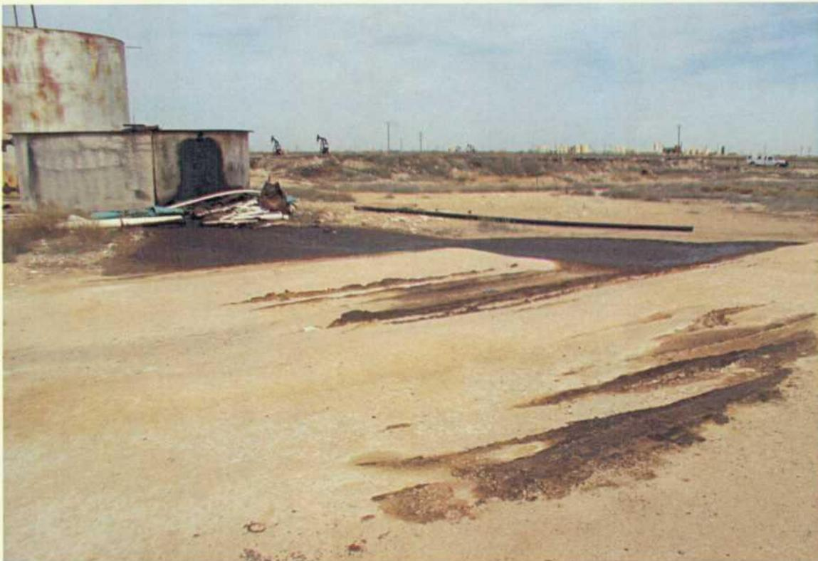
*No. 8 – 200 barrel tank with product that has overflowed on to the surrounding ground surface.*
