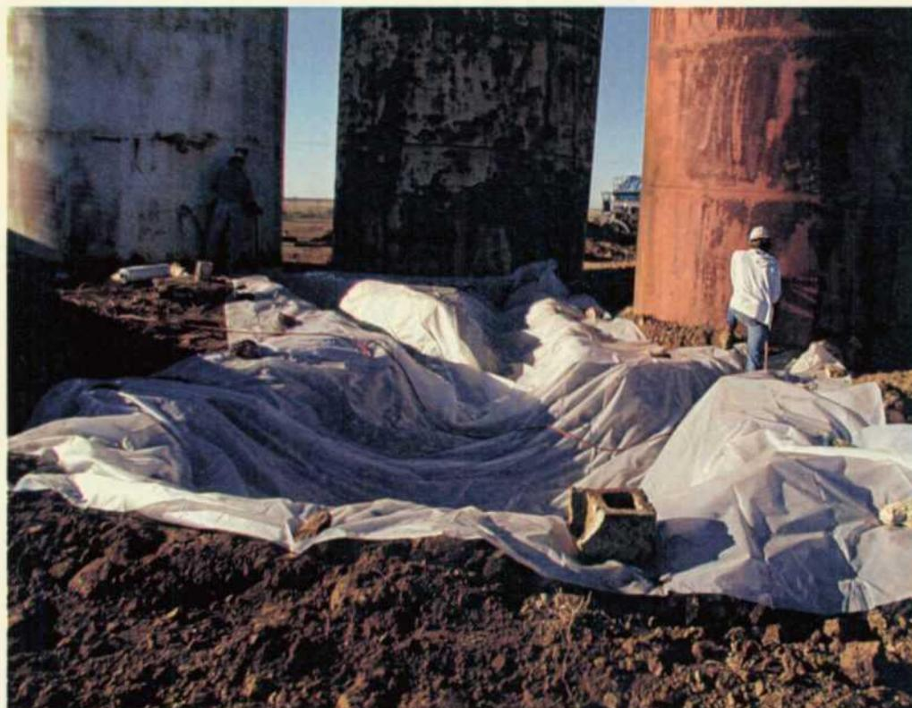
*No. 18 – The pit and plastic used for drained fluid from welded tanks.*
