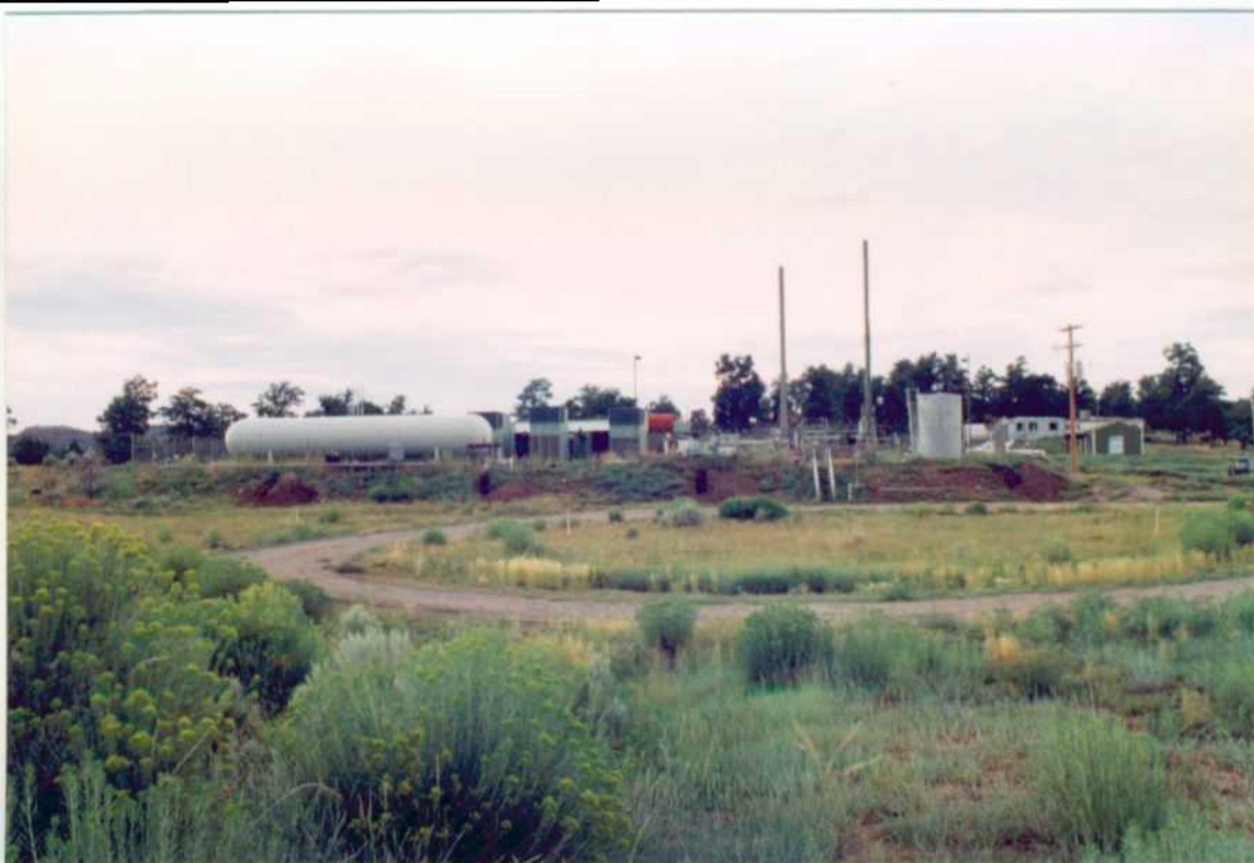
Gavilan Natural Gas Processing Plant
