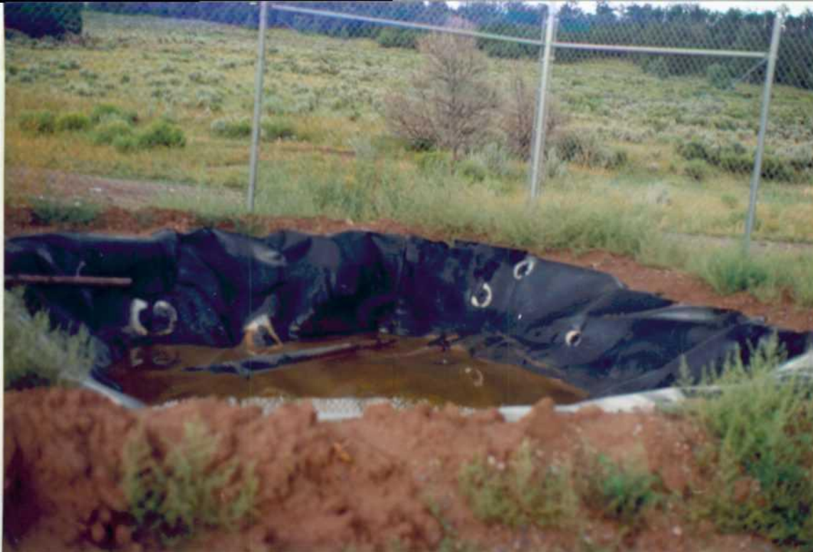
Lined Pit Located at Southeast Corner
