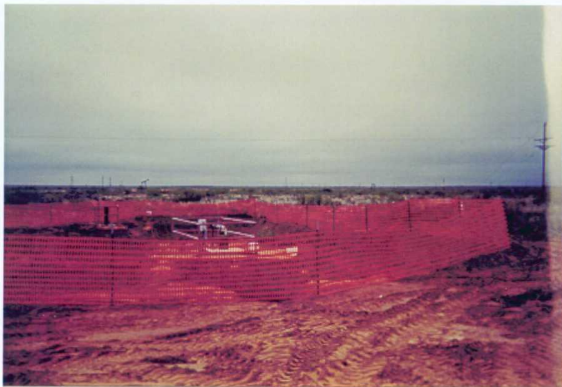
Photo No 4: Affected Area following completion of excavation activities and prior to backfilling/site restoration activities. View looking North.
