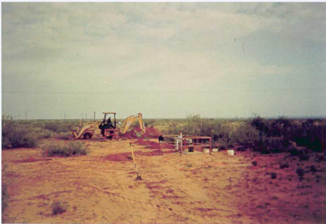
Photo No 1: Affected Area prior to excavation during underground utility location. View looking North.
