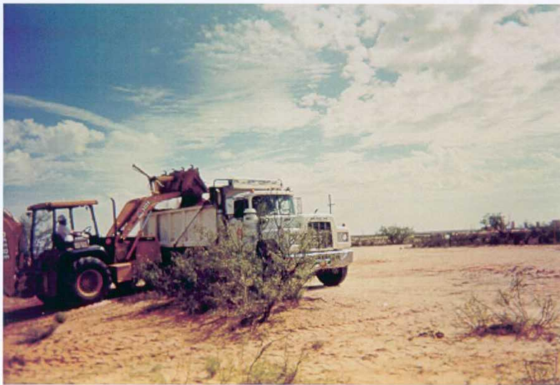
Photo No 3: Impacted soil loading operations. View looking Southeast.
