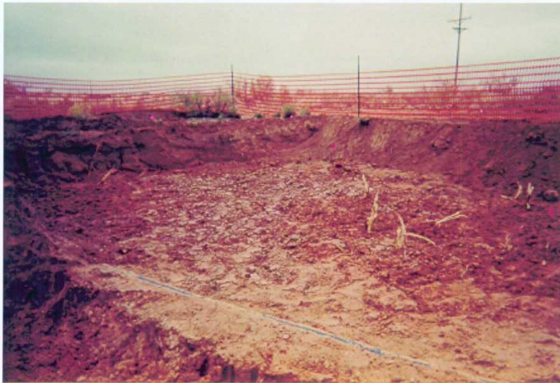
Photo No 2: Northeast portion of the Affected Area following excavation. Note RW-2 discharge line exposed in foreground. View looking Northeast.
