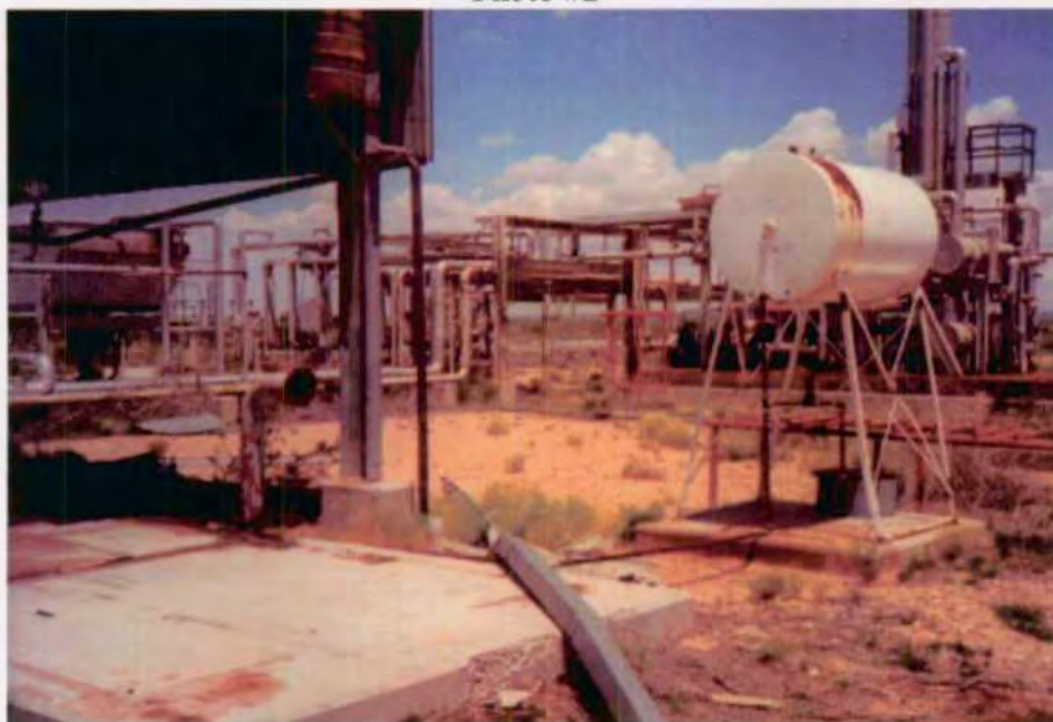
GW-141 CROSSTEX ENERGY SERVICES LOVING GAS PLANT Saddle tank without secondary containment or label
