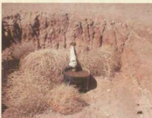
Wastewater pond leak detection system. System is plugged with evaporate solids.
