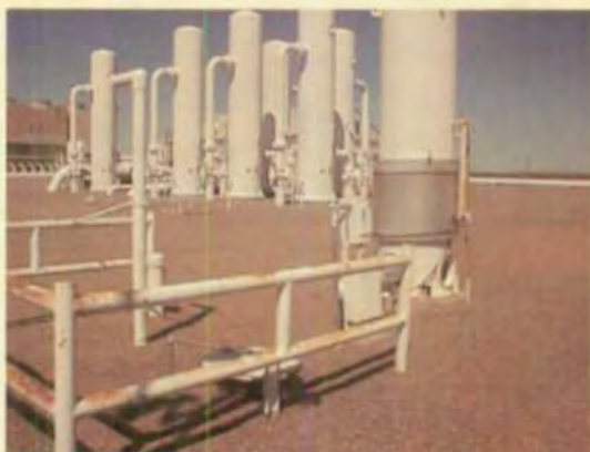
B plant inlet scrubbers and below-grade sump with leak detector.
