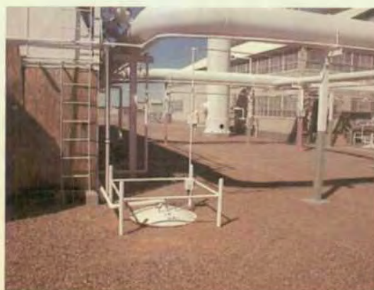
Auxiliary jacket cooling water below-grade sump. No secondary containment.
