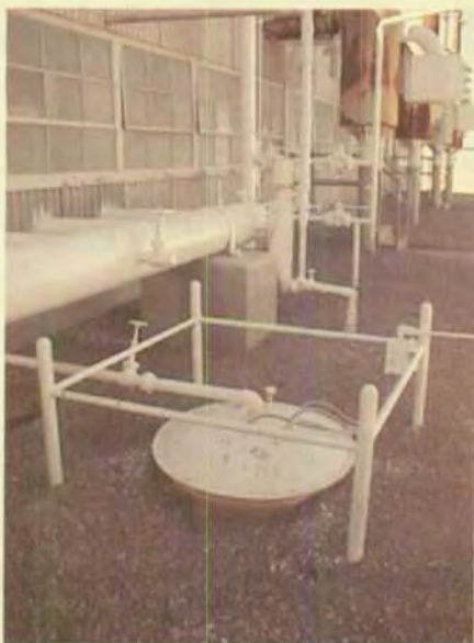
A plant below-grade sump-NO containment.
