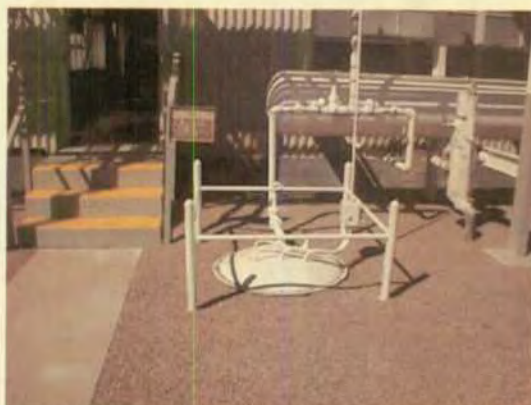
Auxiliary building oil cooling water below-grade sump. No secondary containment.
