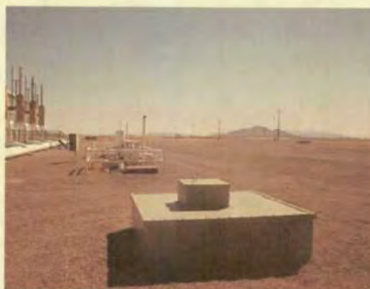
Plant waste water underground valve testing box.
