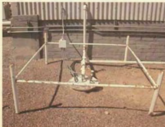
Used oil below-grade sump-no containment.
