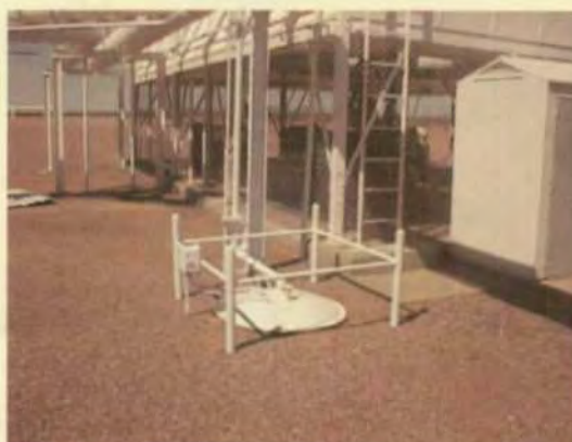
Fin-fan coolers and below-grade water jacket tank-No secondary containment. Located northwest of cooling towers.
