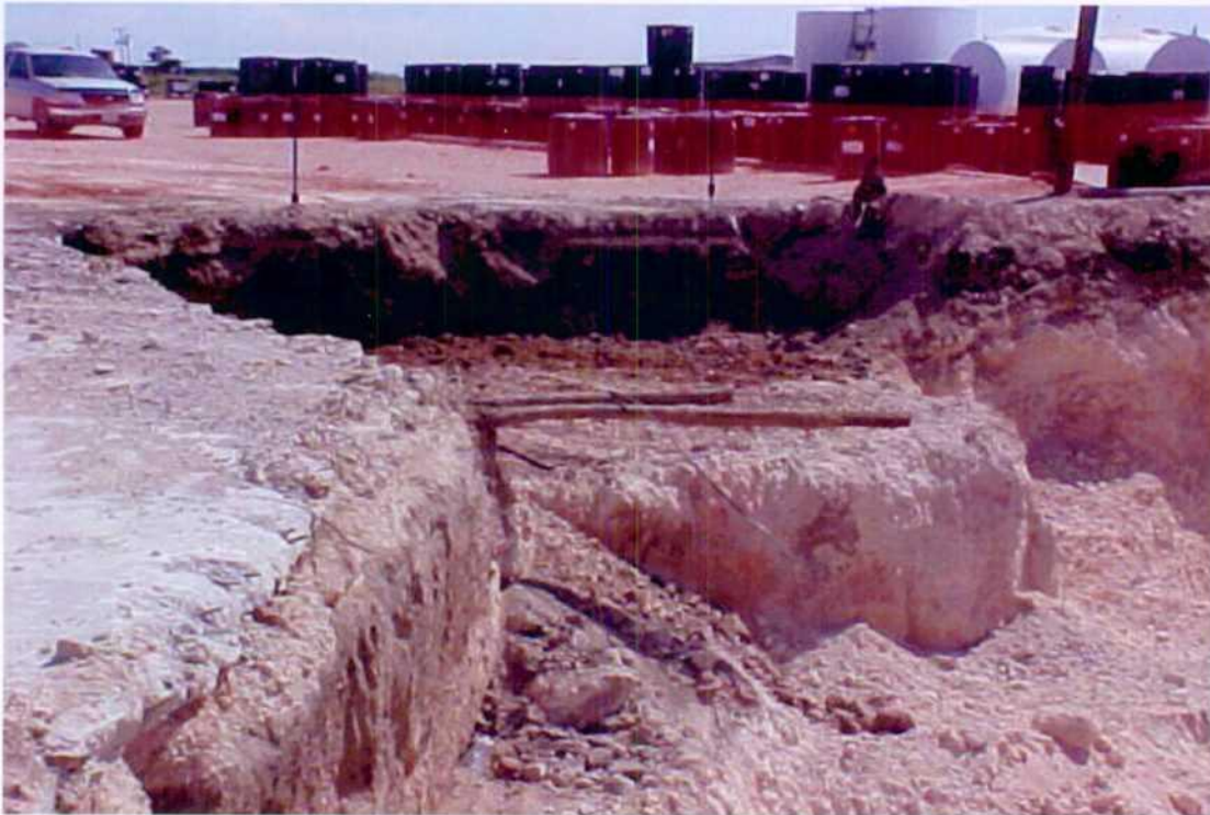
View south-southwest. Metal pipes (drain system) from warehouse exposed (8-10-02).
