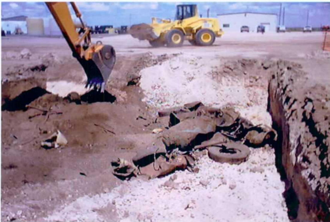
View east. Debris removed from Area 3 "Trenched Area" (7-22-02).
