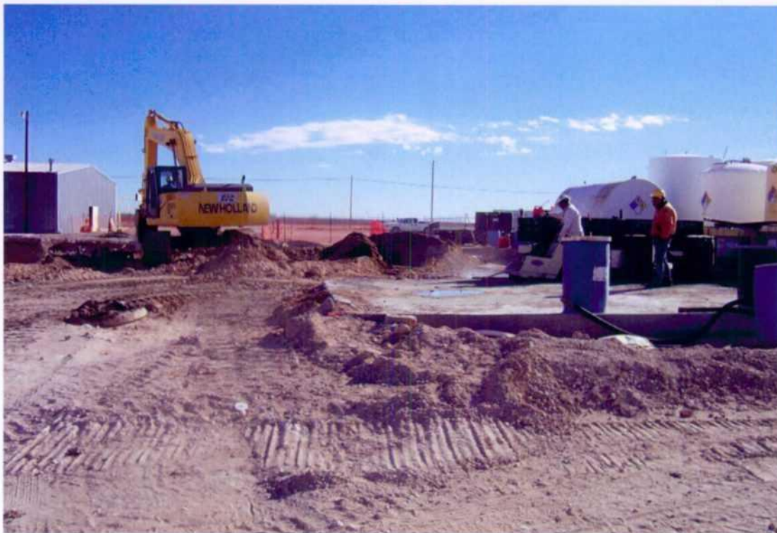
View east. Removal of concrete pad over Area 2 (1-21-03).
