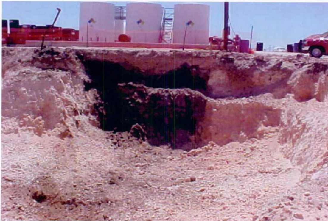
View south. Area 2 west pit sidewall, prior to being excavated out (8-10-02).
