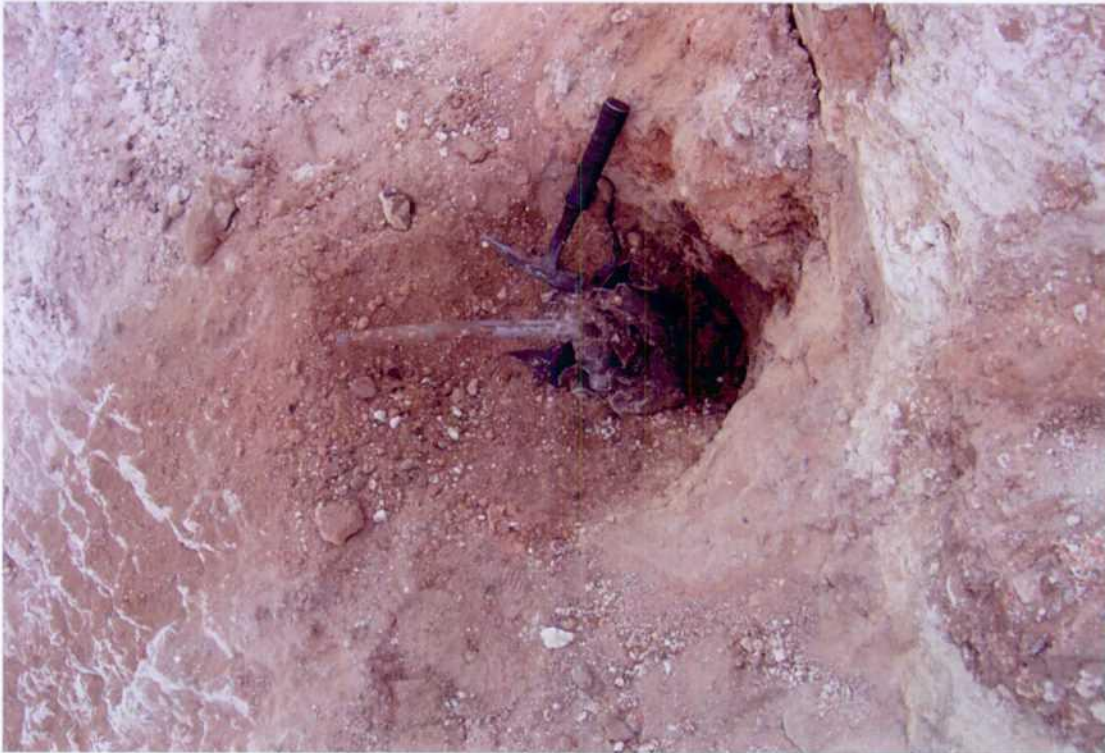
Looking down at "discovered" well casing embedded in south sidewall Area 2 (2-25-03).
