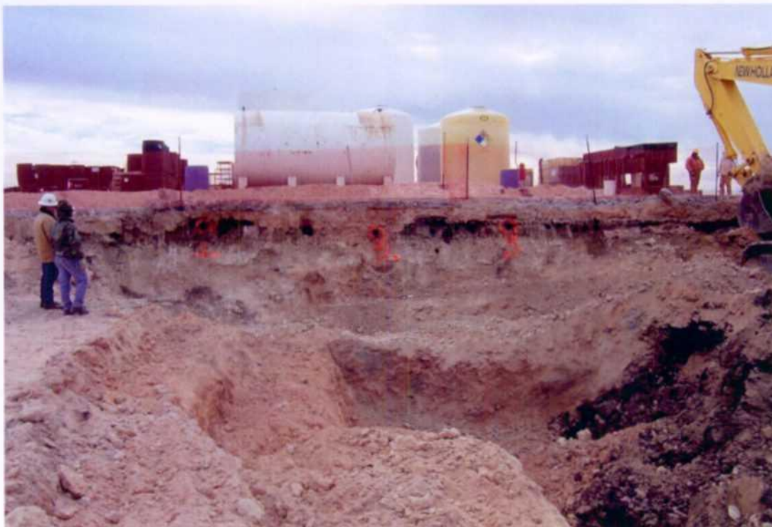
View south. "Final" southwall of Area 2 below remaining bulk chemical containment area (1-28-03).
