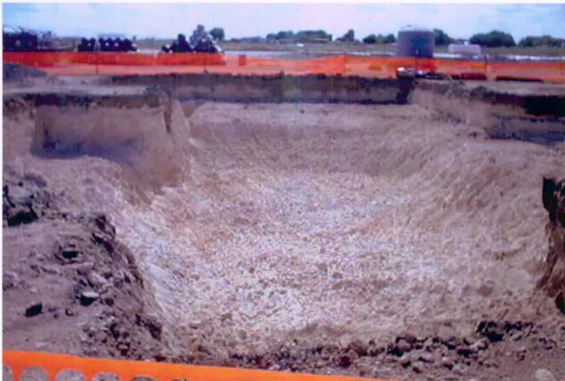
View west. Completed excavation of Area 3 "Trenched Area" (7-23-02).
