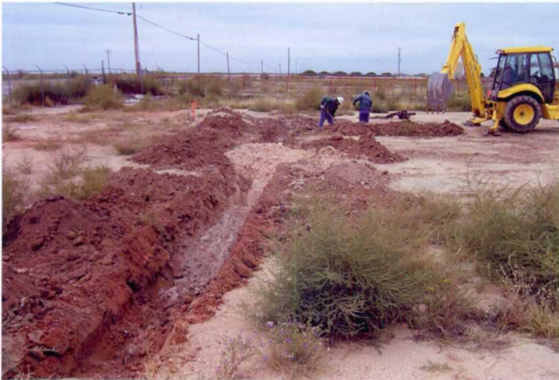
View south. East trench excavation on southeast corner of property.
