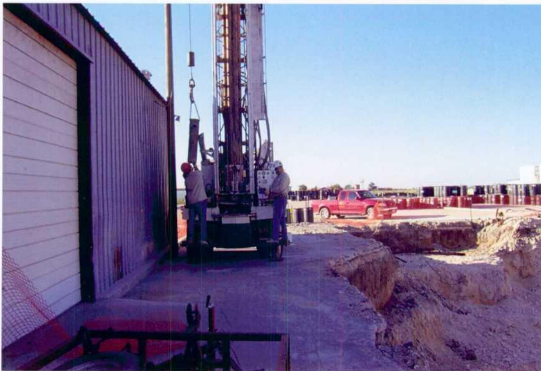
View south. Prepare to install monitor well MW-11 (9-24-02).
