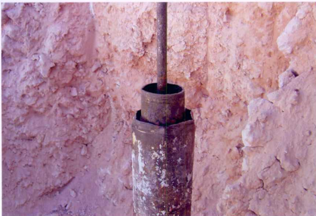
Detail of water well excavated in Area 2 excavation (2-25-03).
