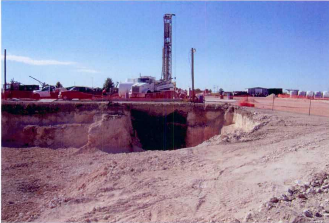
View south. Placement of soil boring SB-49 (9-27-02).
