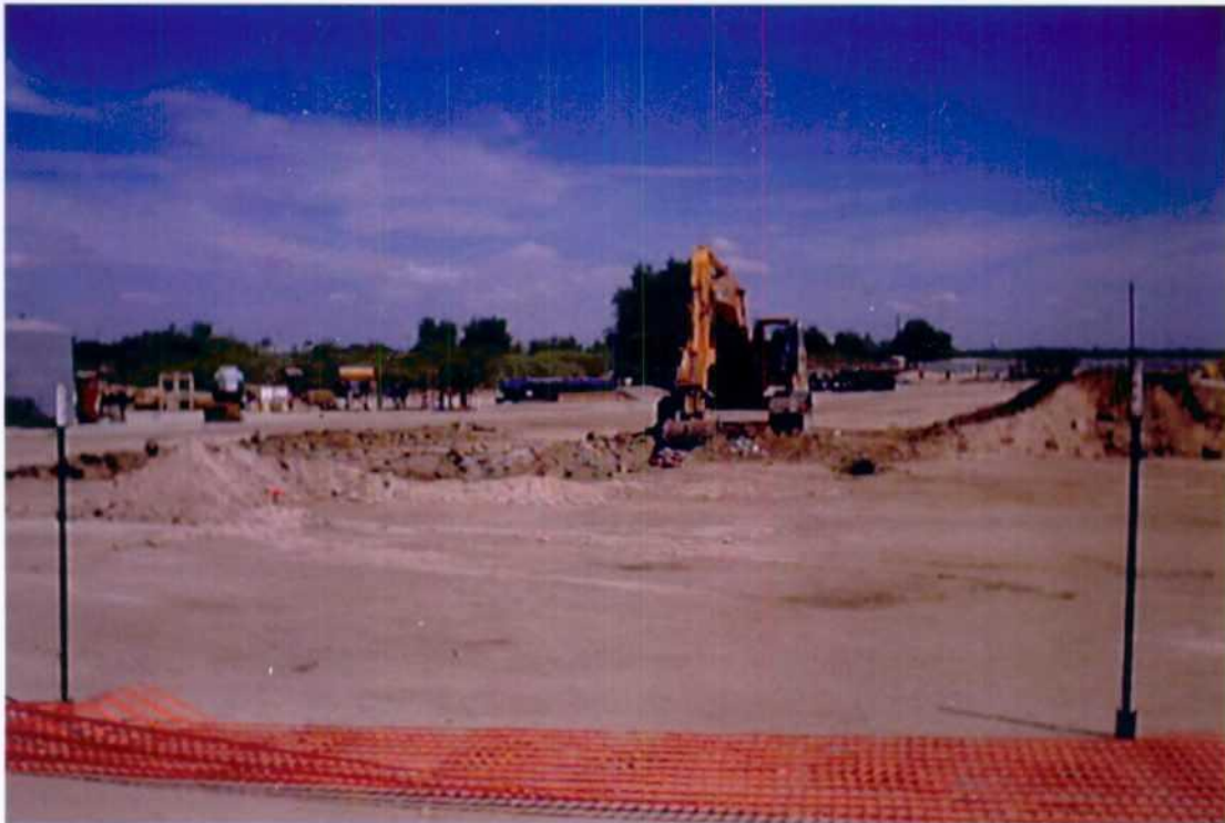
View north. Beginning of excavation of Area 3 "Trenched Area" (7-22-02).
