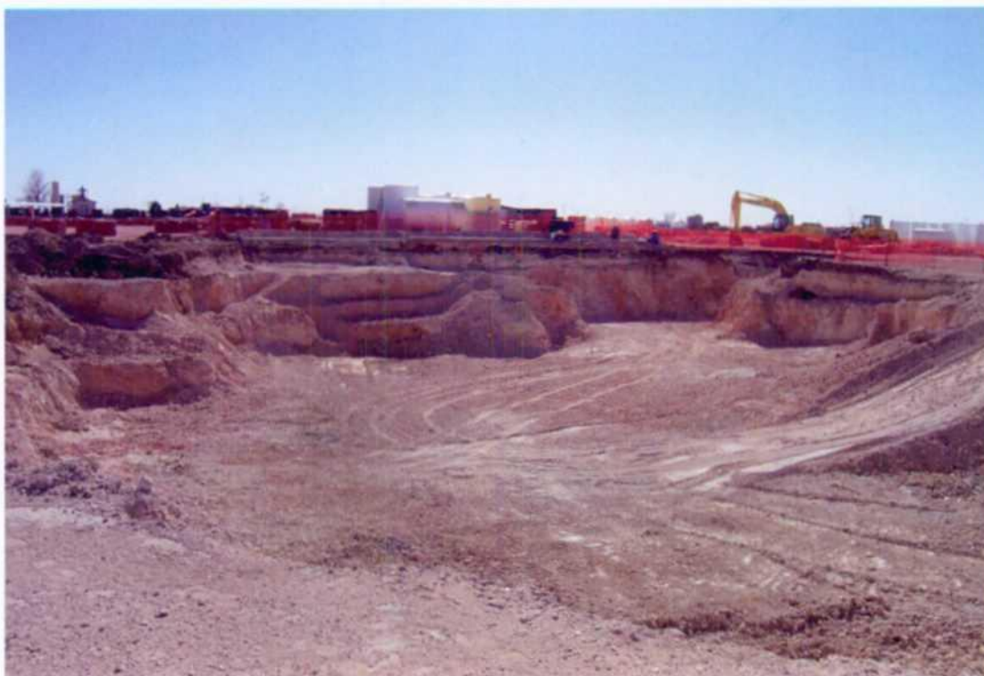
View south. Area 2 excavation complete (1-29-03).
