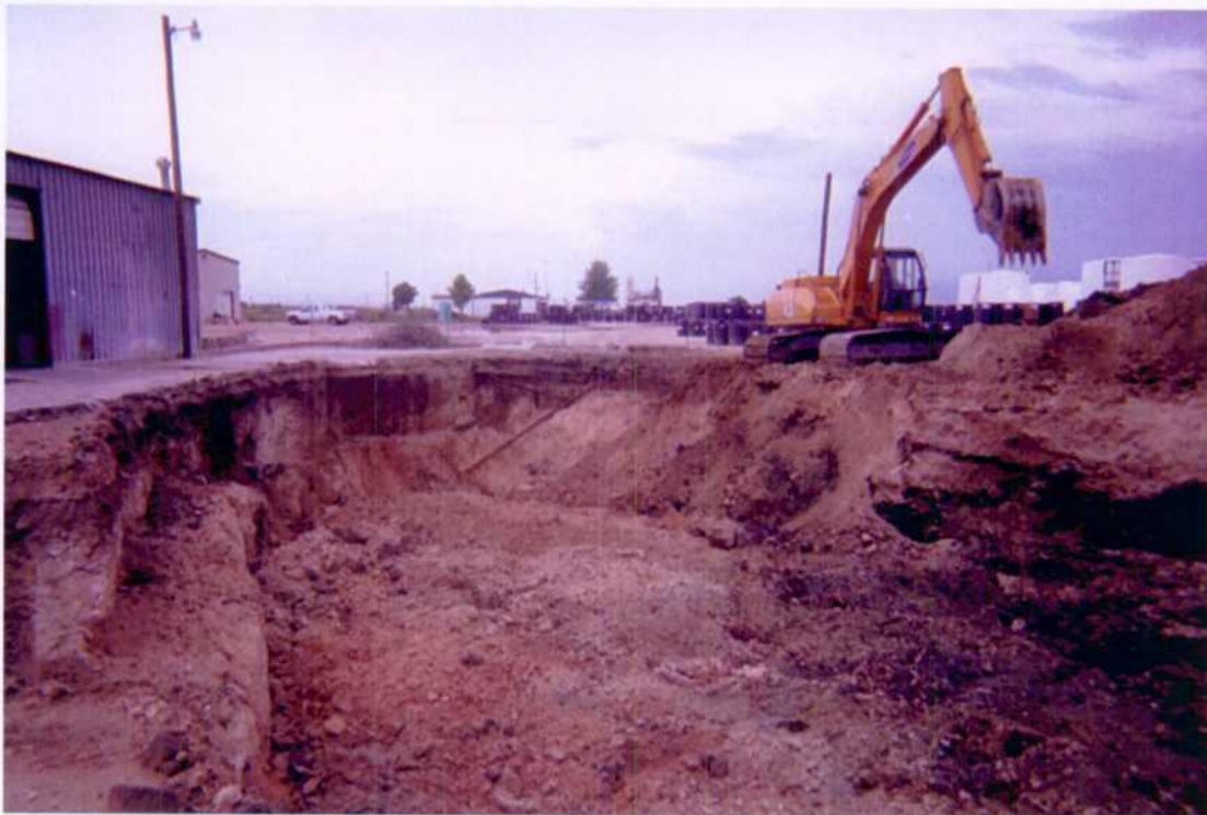
View south. East side of Area 2 excavation (7-31-02).
