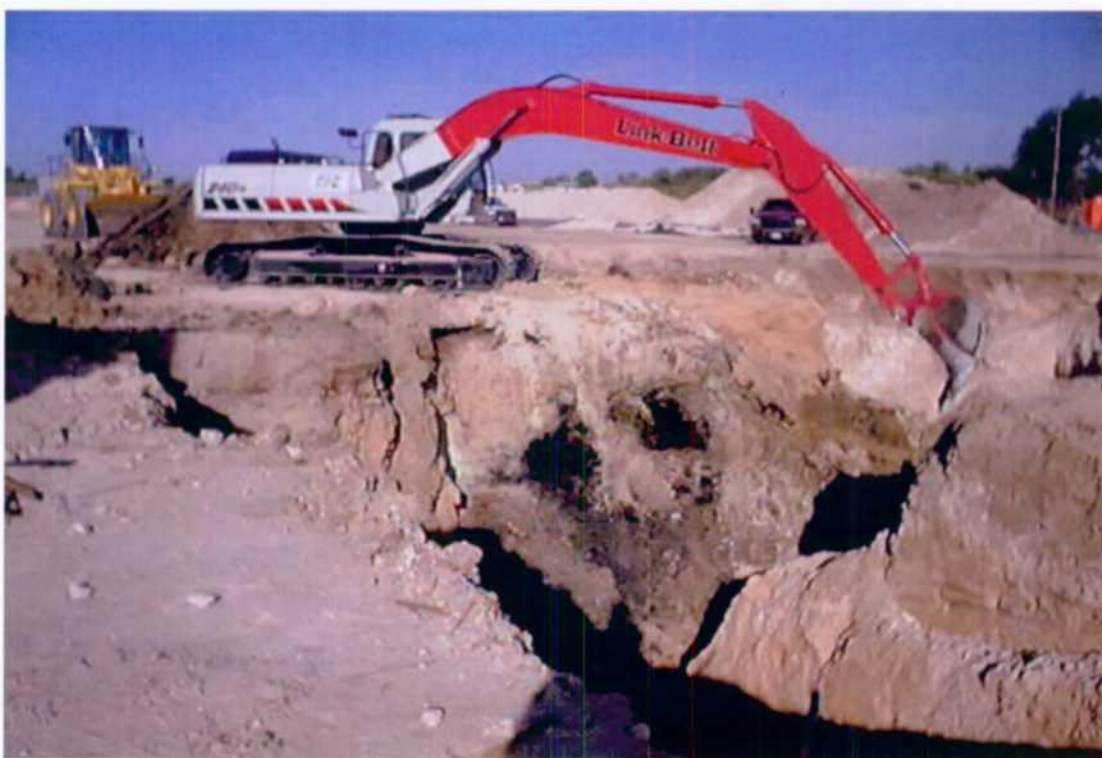
View west. Excavating toward center of Area 2 (7-31-02).
