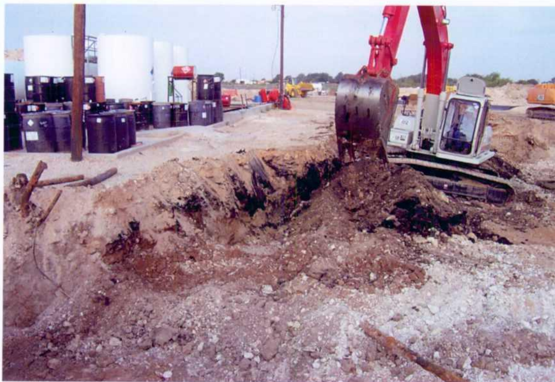
View west. Area 2 excavation north of drum storage area (8-06-02).
