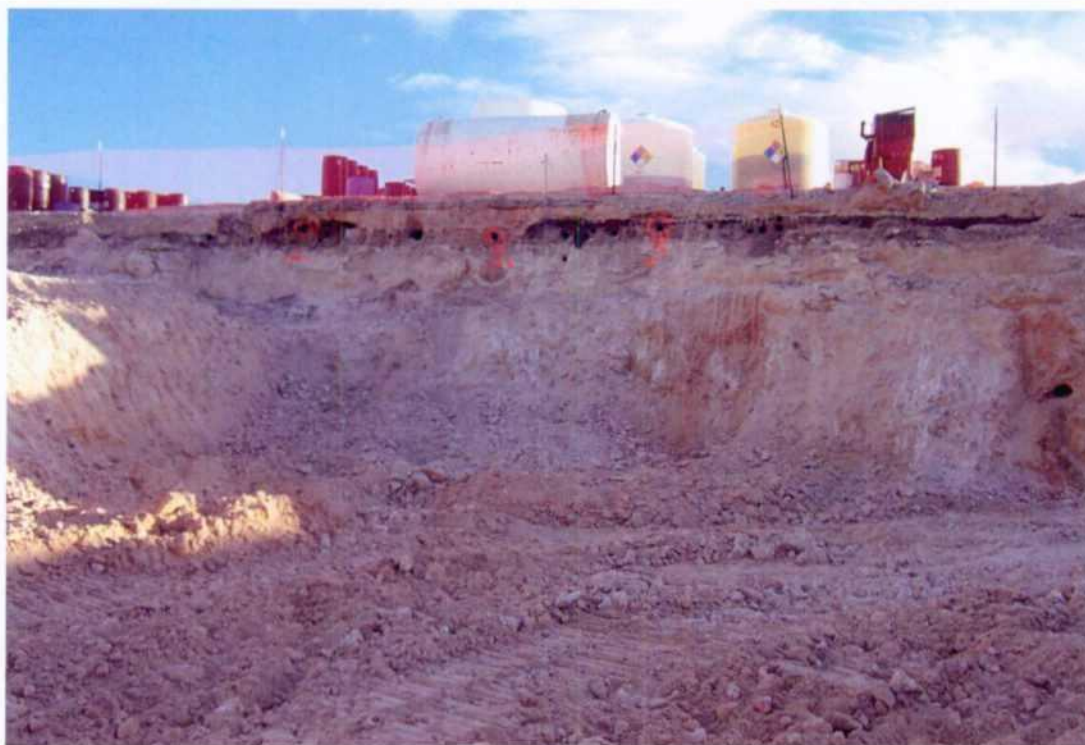
View south. South sidewall of Area 2, view from bottom of Area 2 excavation. (1-24-03)
