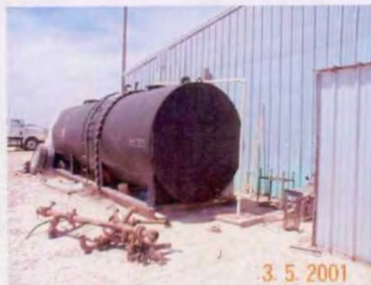
Pic # 5- Wastewater tank and sump receives water from washbay.
