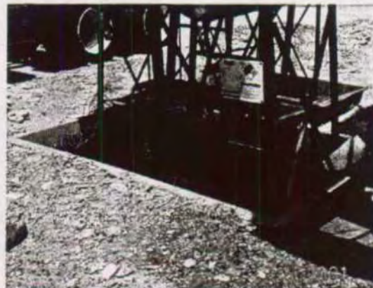
Pic # 12- Chemical storage tanks. Secondary containment has standing chemical and water.
