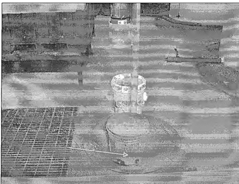
Photo 4: Bucket will need to be replaced with a non-corrosive bucket.
