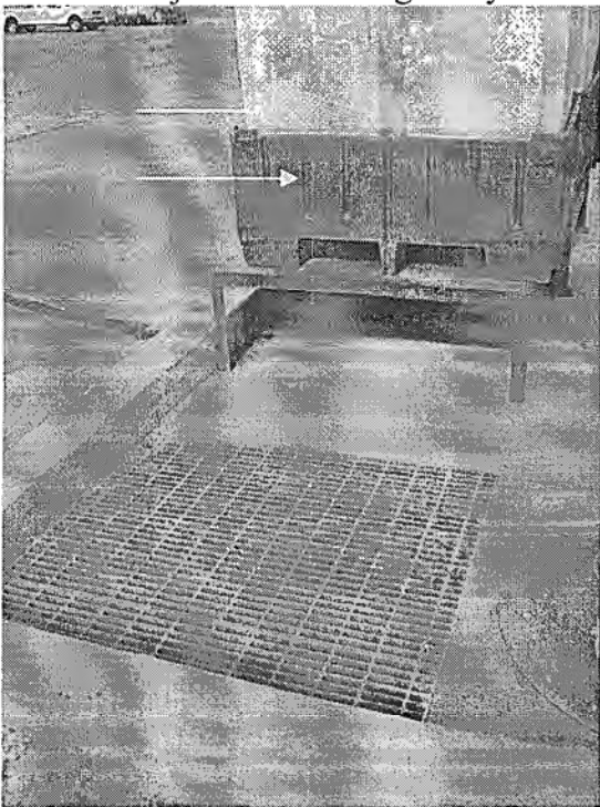
Photo 2: Tote tanks need to move back and away from curbed edge to prevent spillage from loading.
