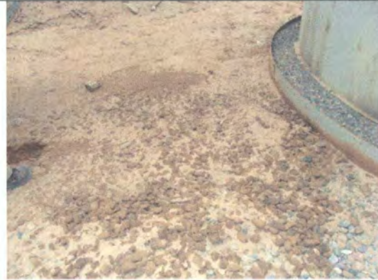
Photo 10: Discharge from AST on to unlined secondary containment area.
