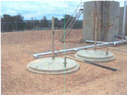
Photo 2: 2 and 3 BGT for AST's. Lead detection verified dry.
