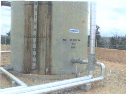
Photo 9: Overflow of AST on to unlined secondary containment.
