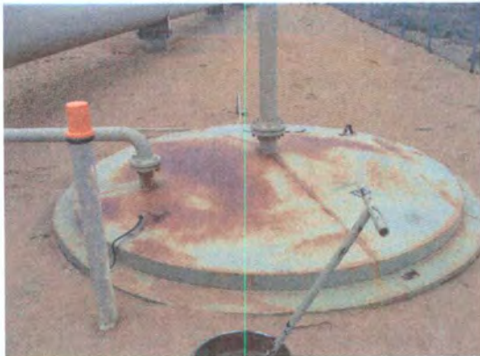
Photo 1: 1 BGT, for pigging liquids. Leak detection verified dry.
