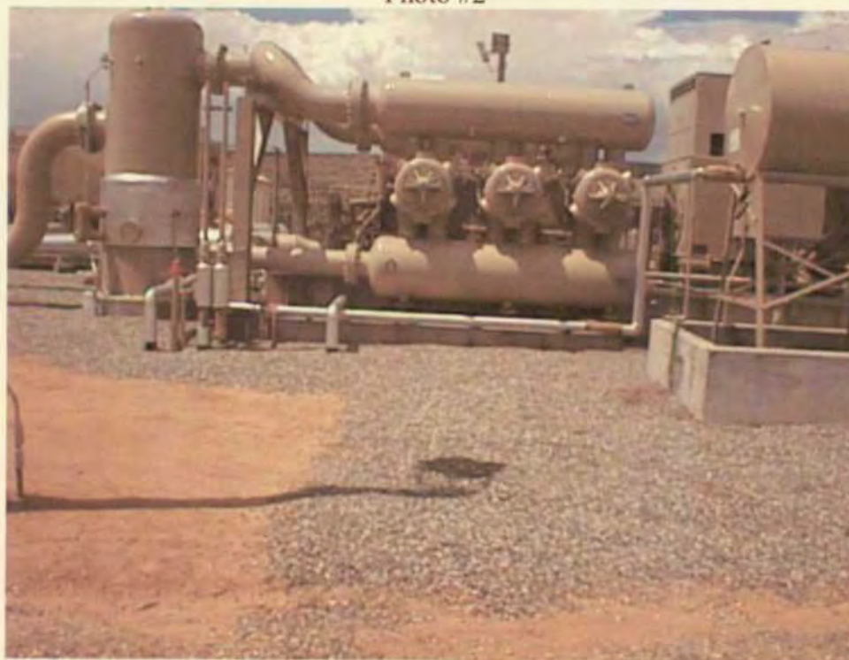
GW-303 EL PASO FIELD SERVICES NAVAJO CITY COMPRESSOR STATION Compressor unit with saddle tank within concrete containment structure
