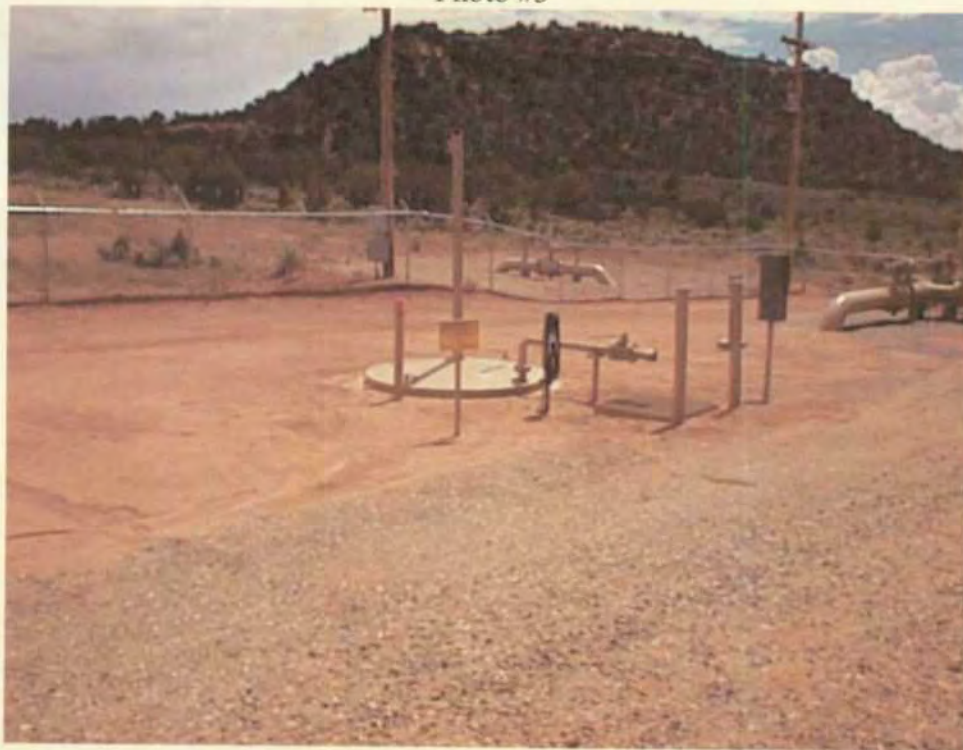
GW-303 EL PASO FIELD SERVICES NAVAJO CITY COMPRESSOR STATION Waste water collection tank with internal monitoring system
