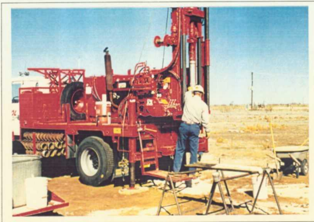
Photograph No. 5 Drilling MW - 12.
