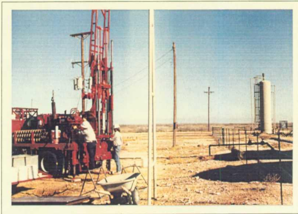
Photograph No. 2 Drilling MW - 6
