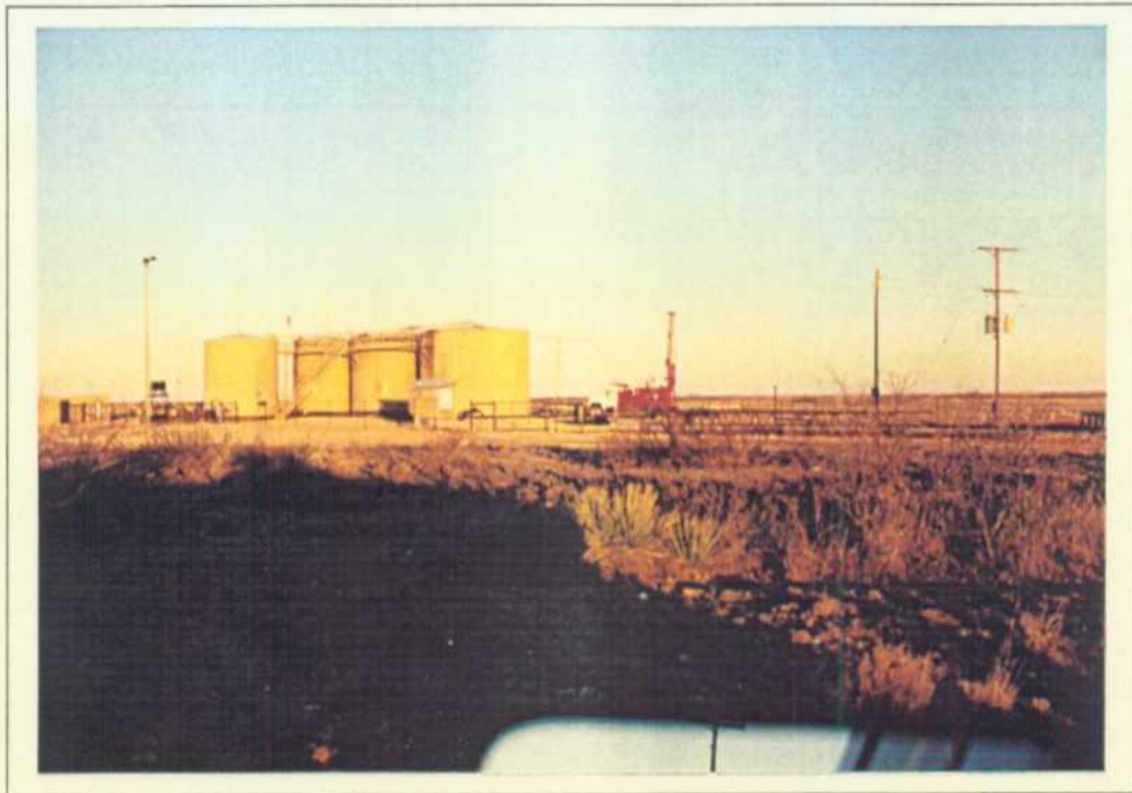
Photograph No. 1 Site Drilling Operations
