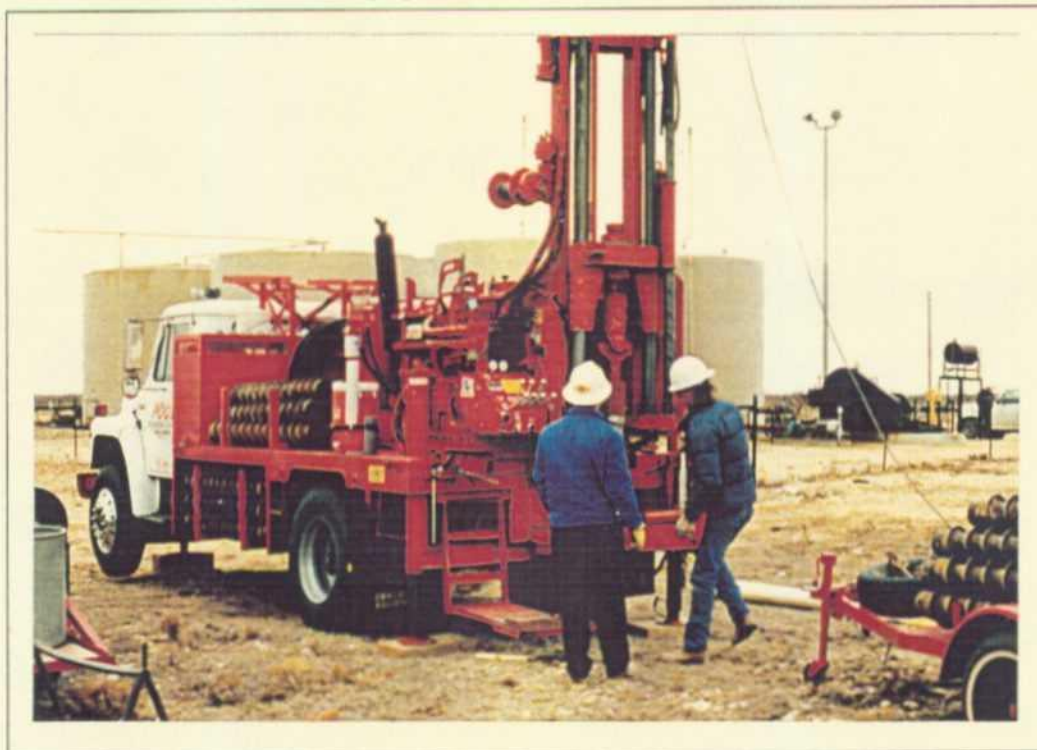
Photograph No. 6 Drilling of MW - 5.
