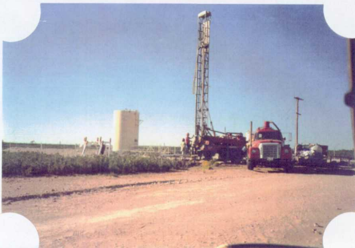
Photograph 2: View of drilling operations on monitor well MW-.1
