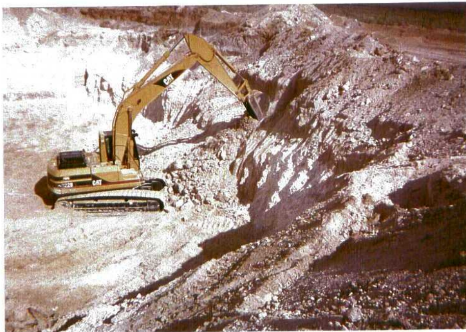
Photo 8: Removal of clean overburden in order to access contaminated soils.
