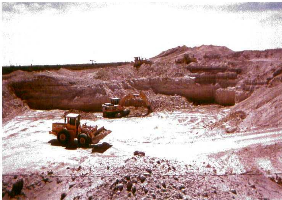
Photo 12: Excavation of south side of the site.
