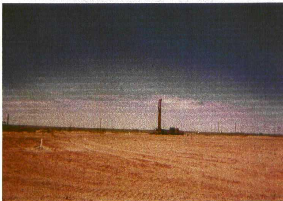
Photo 21: Drilling of soil boring SB-1.
