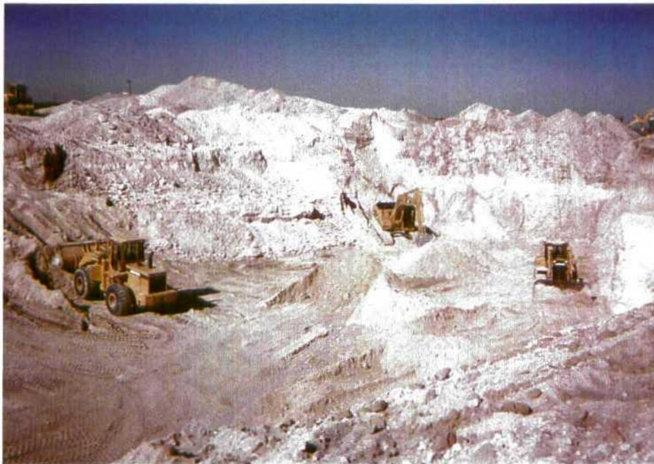
Photo 9: Excavation of contaminated soils.
