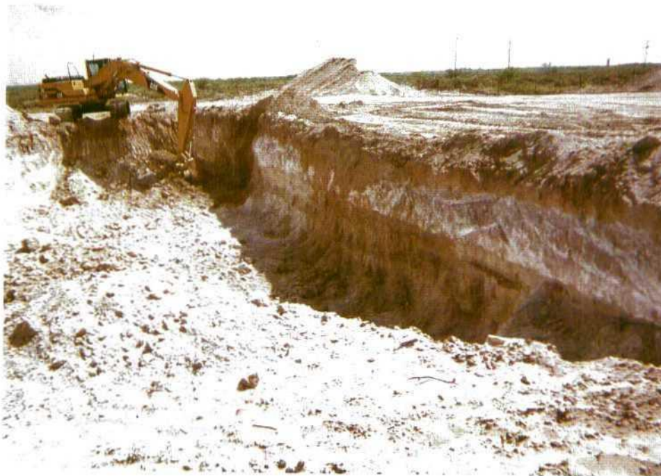
Photo 4: Excavation of contaminated soils to south along pipeline right-of-way.
