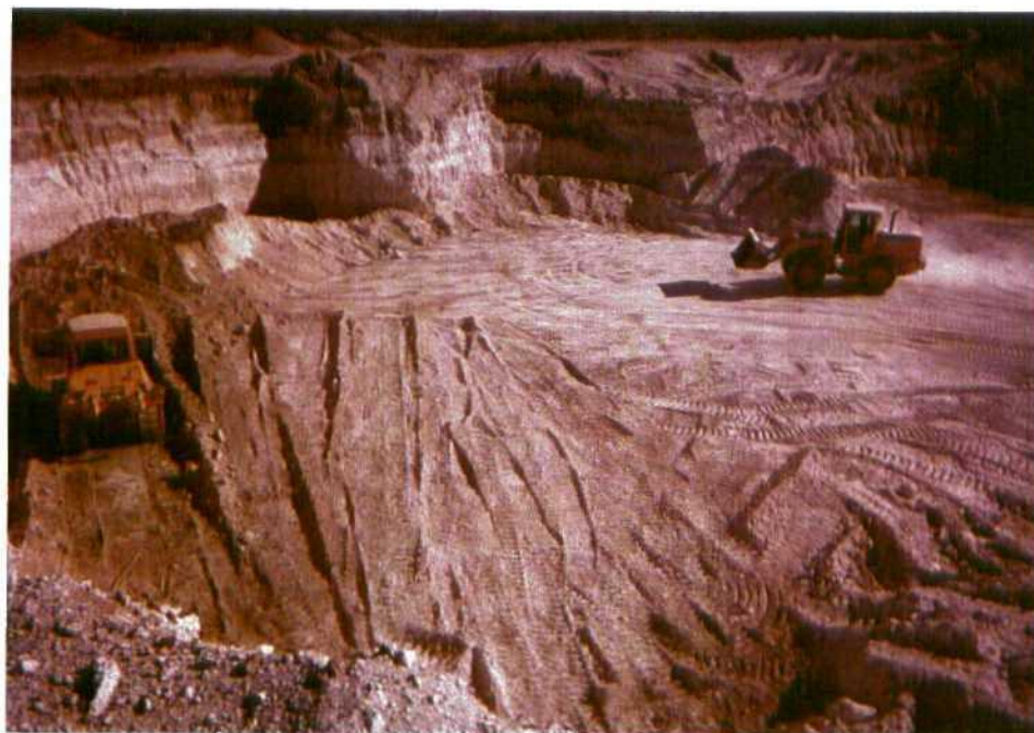
Photo 14: Removal of contaminated soils from bottom of pit.
