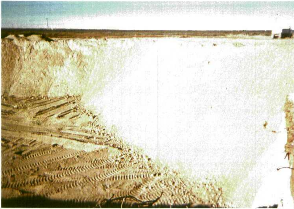
Photo 23: Backfilling clean soils along west side of pit
