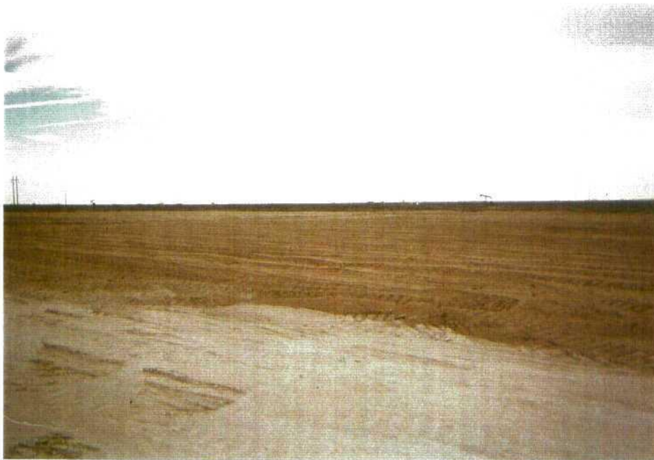
Photo 28: Completed backfilling of site.
