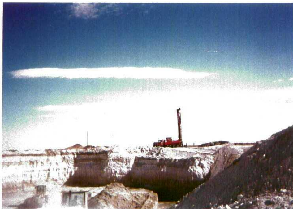
Photo 16: Drilling soil borings along GPM gas line located on southeast corner of site.
