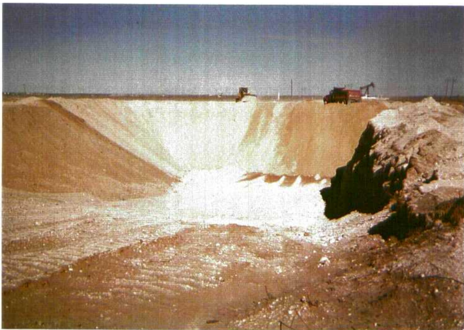
Photo 24: Backfilling of site.
