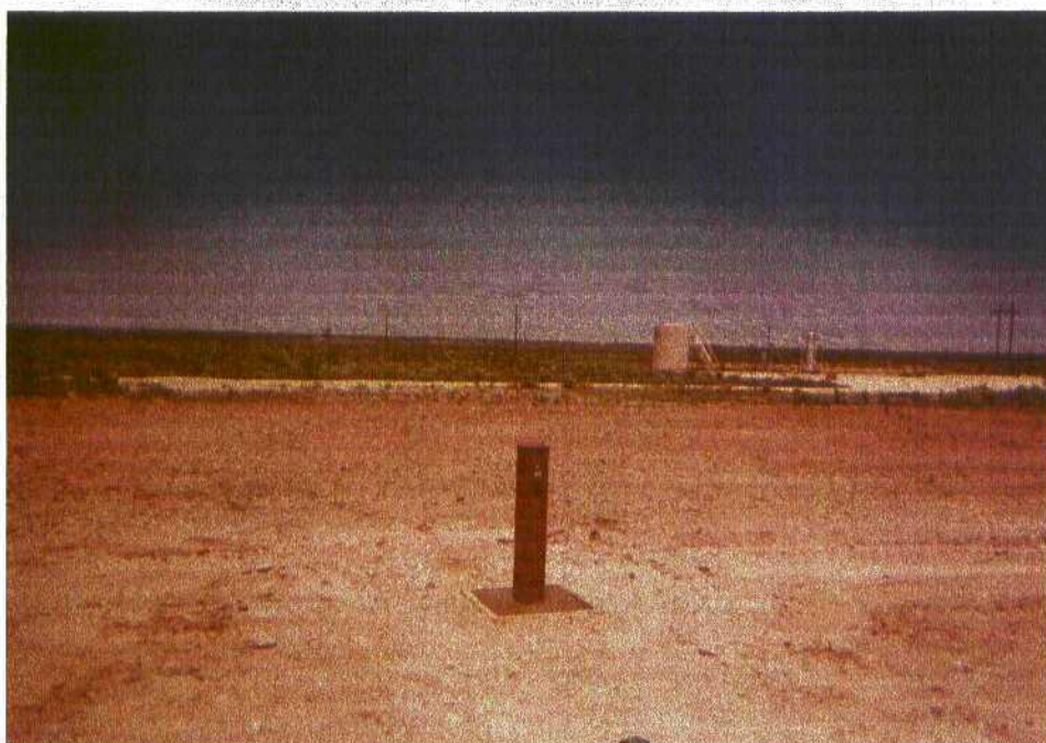
Photo 3: Installation of pipe for monitor well MW-1.
