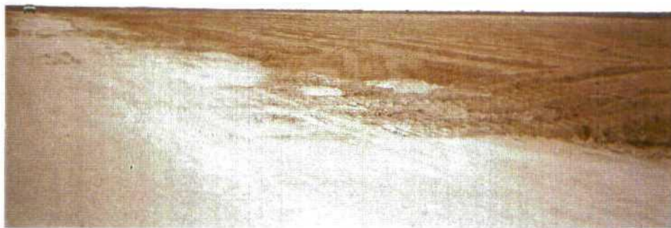
Photo 30: Completed backfilling of site.
