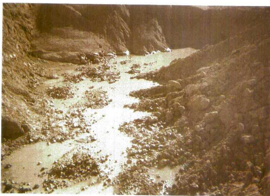
Photo 22: Groundwater along the east side of the pit.
