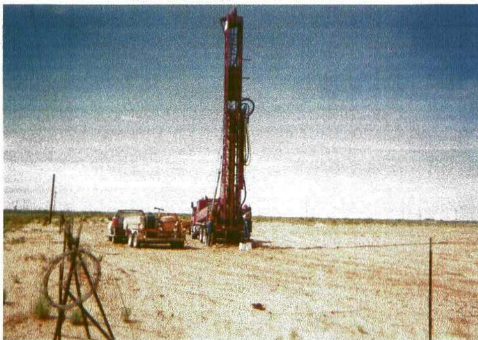
Photo 6: Drilling of monitor well MW-2.
