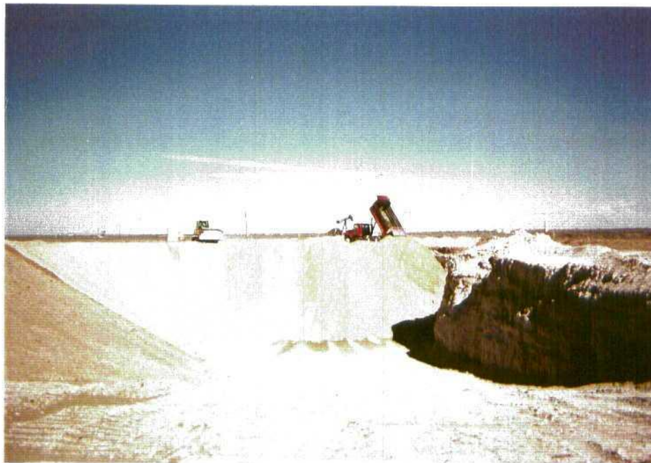
Photo 26: Backfilling of site.
