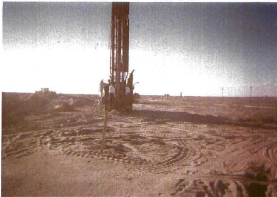
Photo 18: Drilling of soil boring C-2 along GPM gas line on east side of site.
