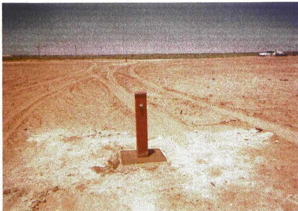
Photo 12: Completed monitor well MW-3.
