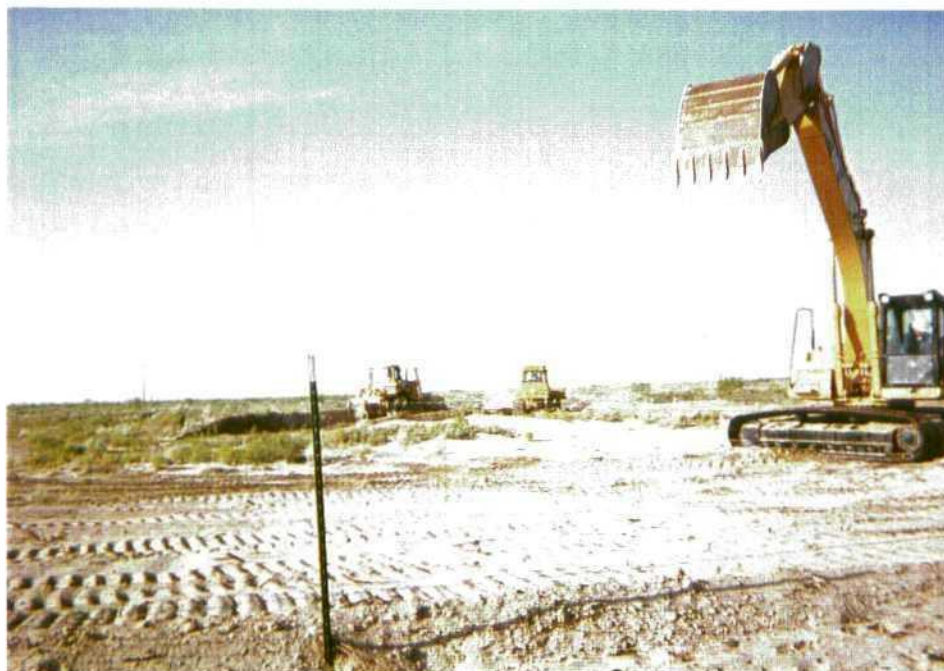
Photo 2: Removal of clean overburden soil in order to access contaminated soils.
