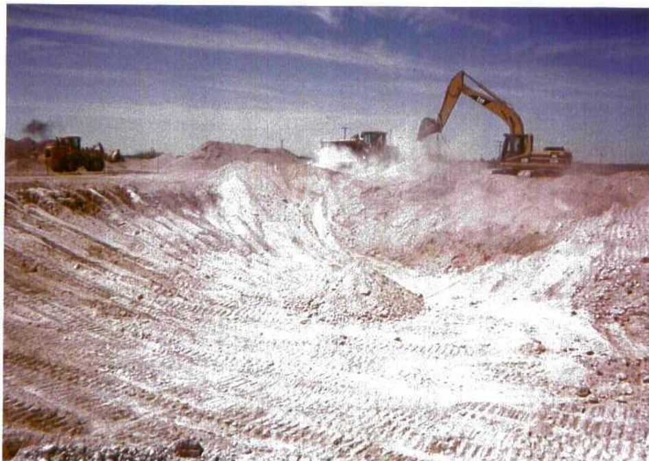
Photo 6: Removal of clean overburden to get to contaminated soils.
