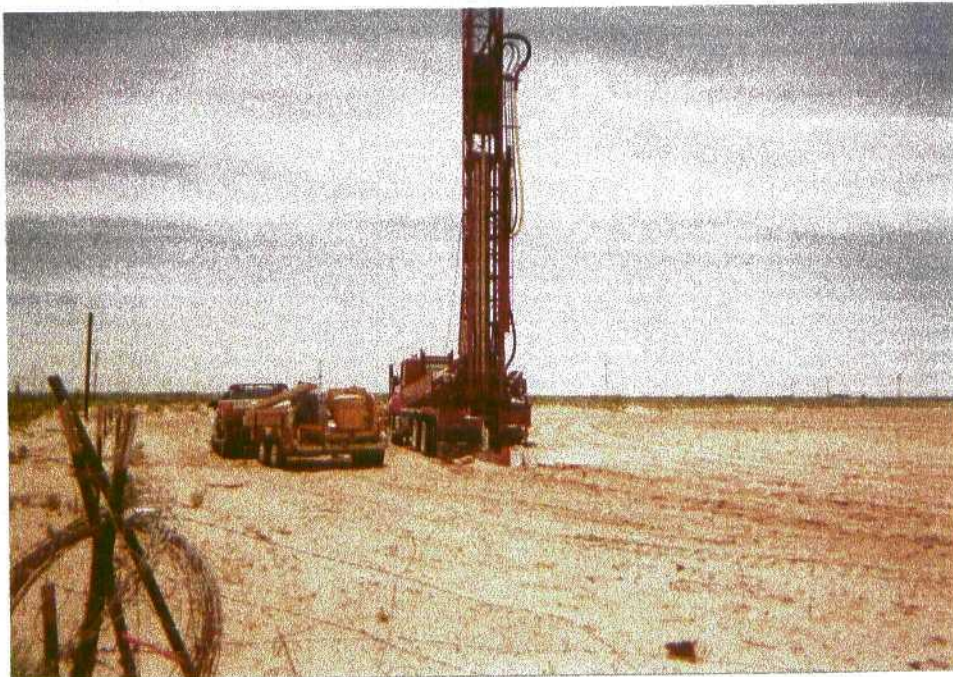
Photo 7: Drilling of monitor well MW-2.
