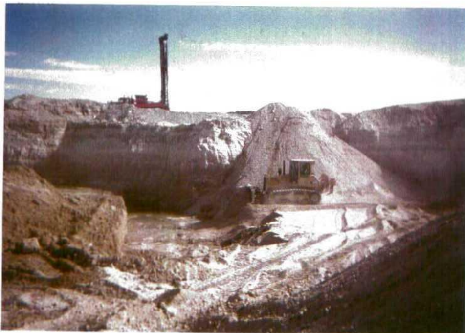
Photo 17: Backfilling soils on south side of site.
