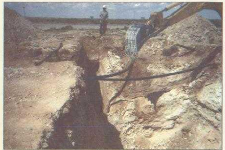
Backhoe Delineation & Excavation
