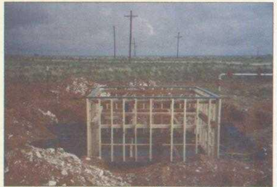
Construction of New Junction Box 150 ft West of Old
