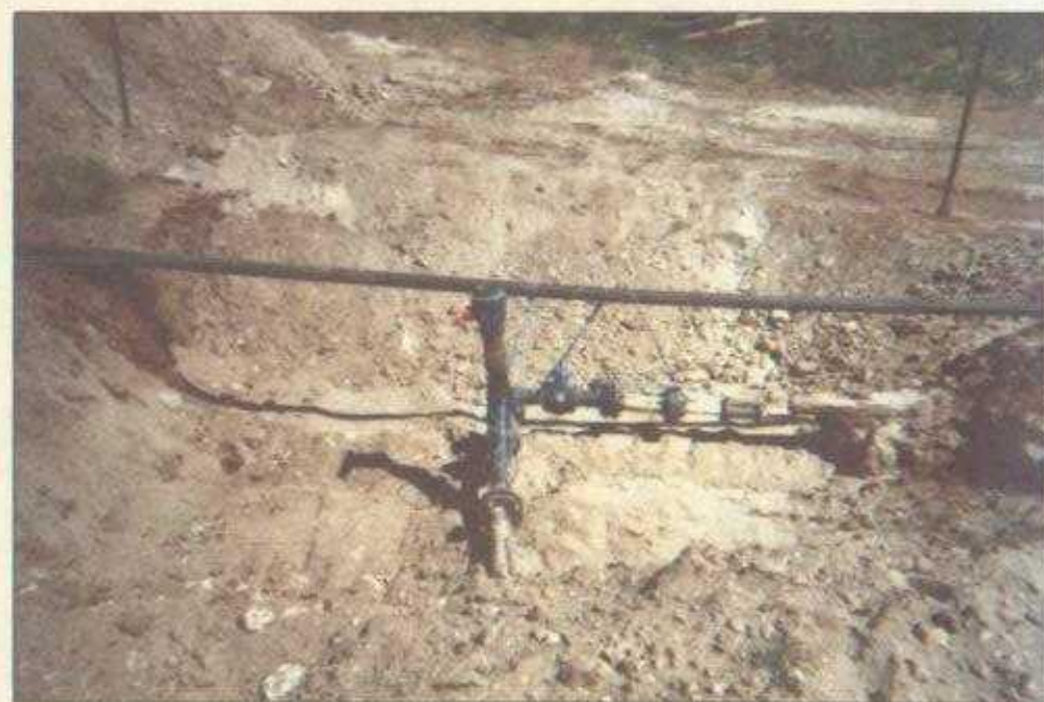
Backfilled to the pipeline 8/1/2003
