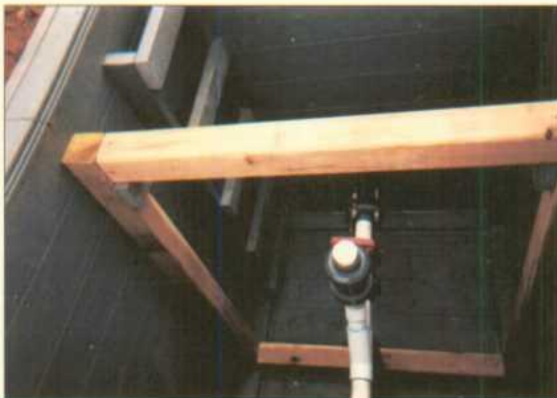
New Box Construction
