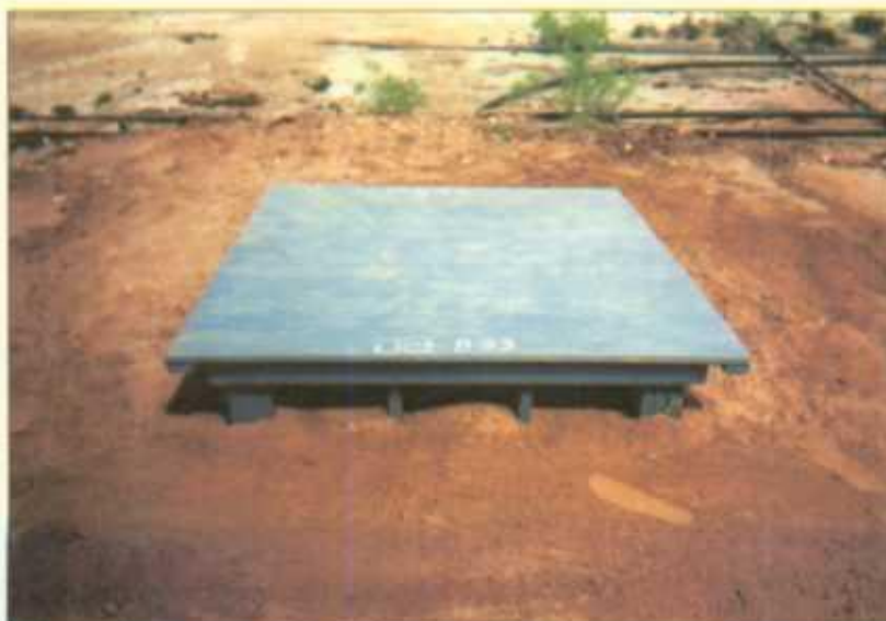
Completed Junction Box
