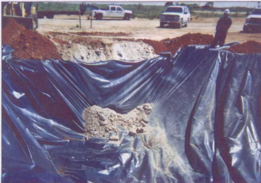
Installation of Poly Liner
