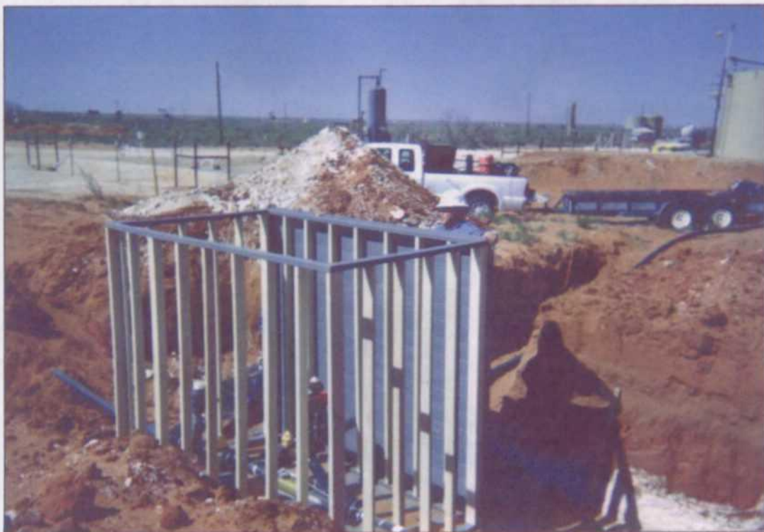
New Junction Box Construction (40' west of excavation)
