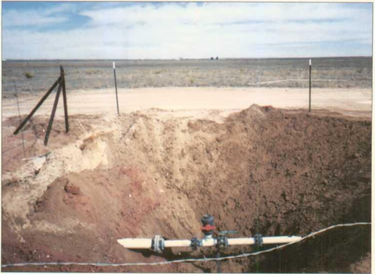
Remediation with New Plumbing
