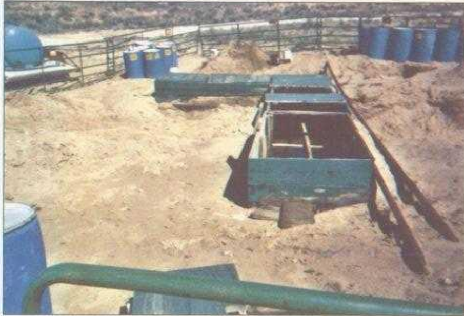
Removing NORM From Old Jct. Box (April 2003)
