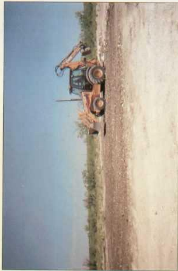
contouring surface of backfilled site
