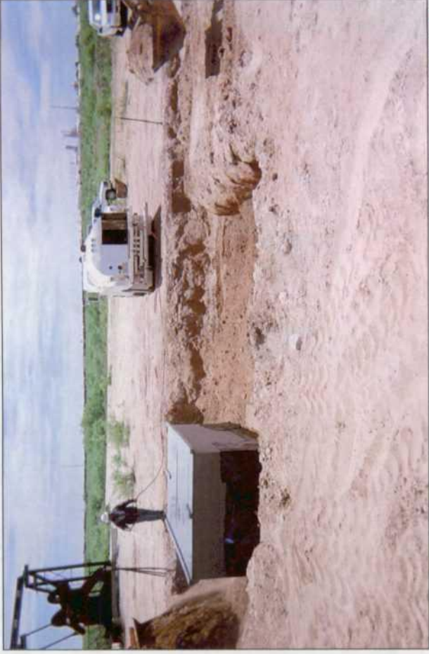
completing junction box; compacting surrounding soils
