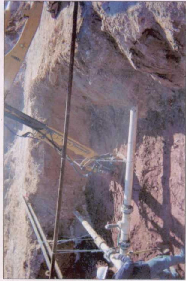
Installing and compacting clay barrier
