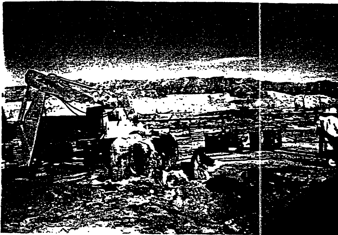
9: Jackhammer on backhoe used to remove concrete from metal tank.
