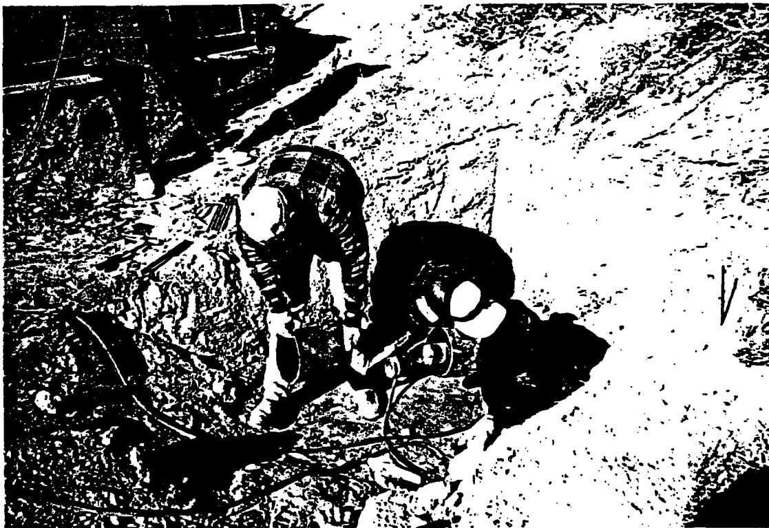
7: Three-inch pipes cut and capped; placing cap on ten-inch conduit.
