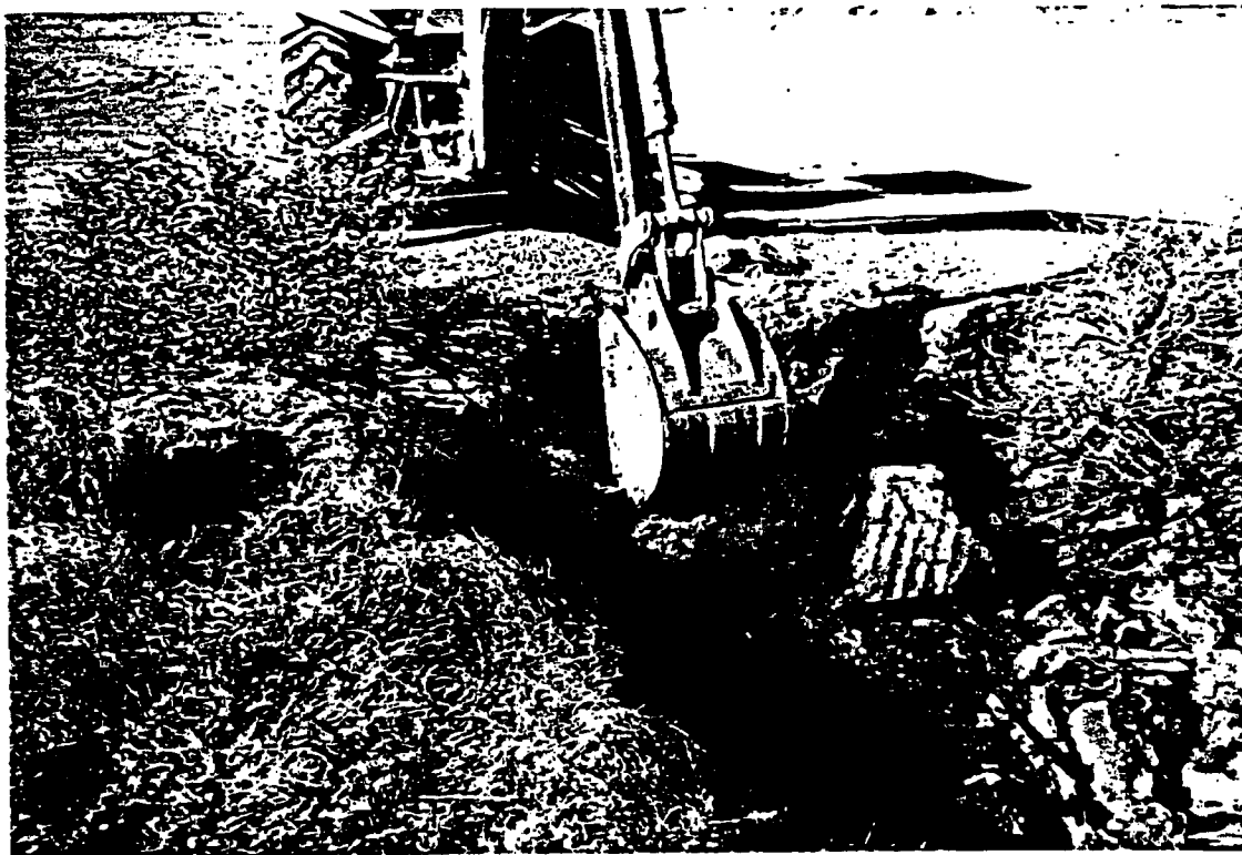
3: View looking northwest: pushing in sides of wash water collection sump.
