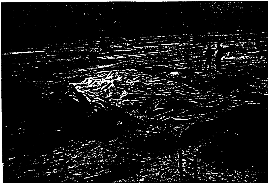
22: View looking west; HDPE covering north asphalt spill area; backfilling trench on south side of spill.
