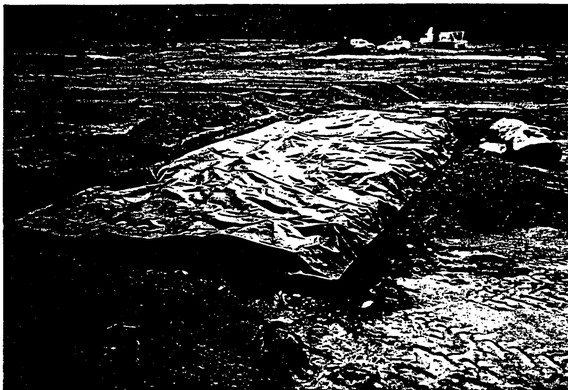
21: View looking west; HDPE covering north asphalt spill area.
