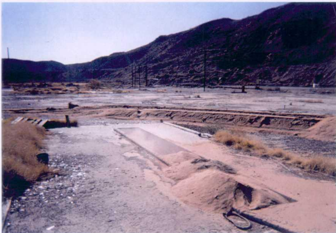
1: View looking south; backfilling service pit.
