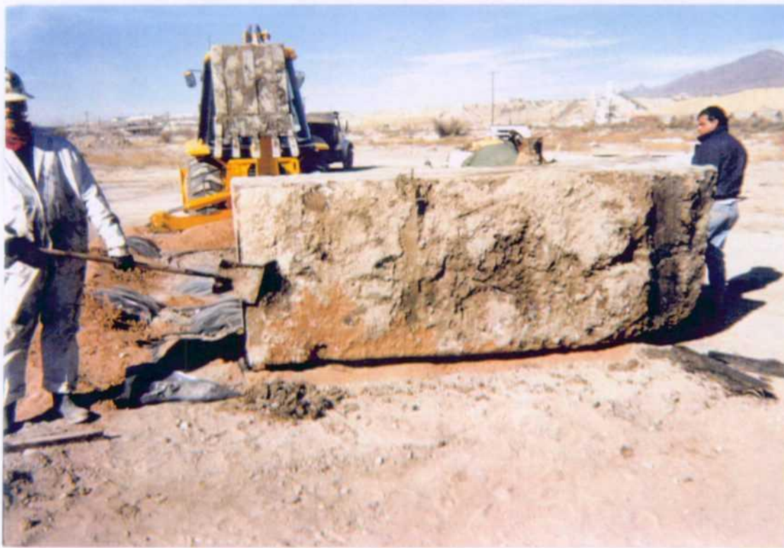
8: Sump placed in containment structure. View looking at base of sump.
