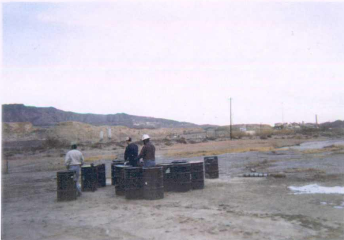
11: Waste is placed in DOT approved drums and sealed for transportation.
