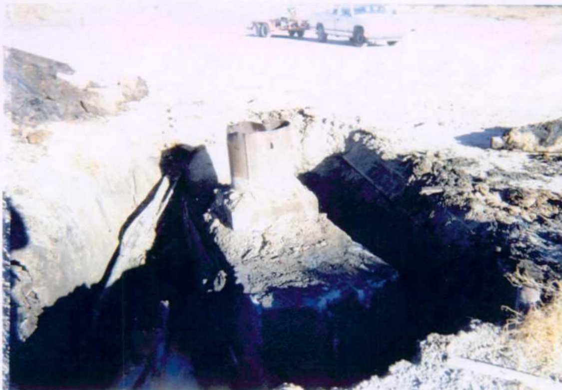
3: Excavated top and sidewalls revealing concrete sump.
