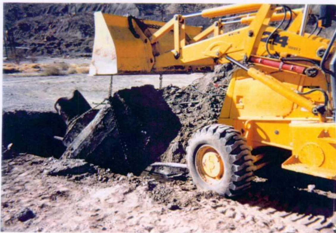
6: View looking southwest; lifting sump from tankhold.
