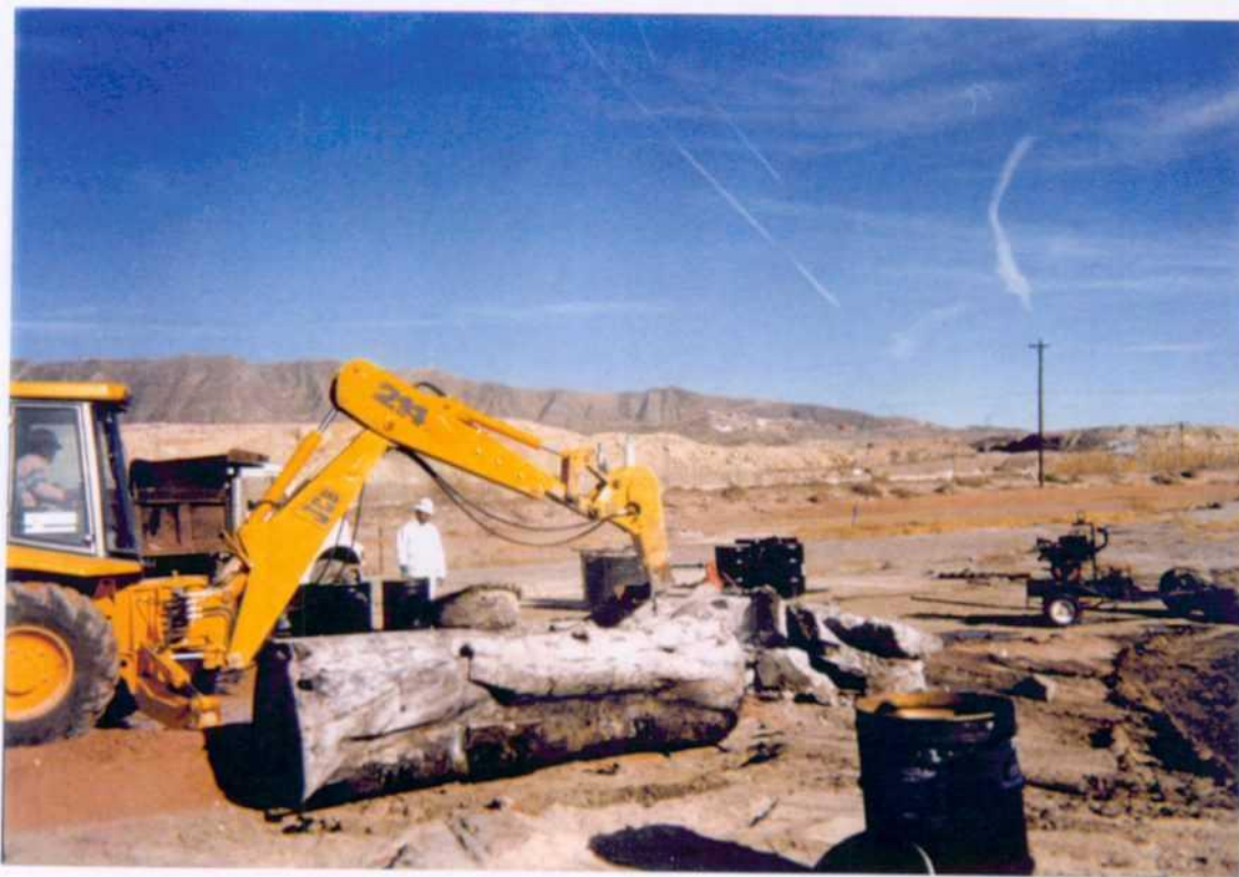
10: Concrete from sump is segregated to prevent coming in contact with the tank contents.
