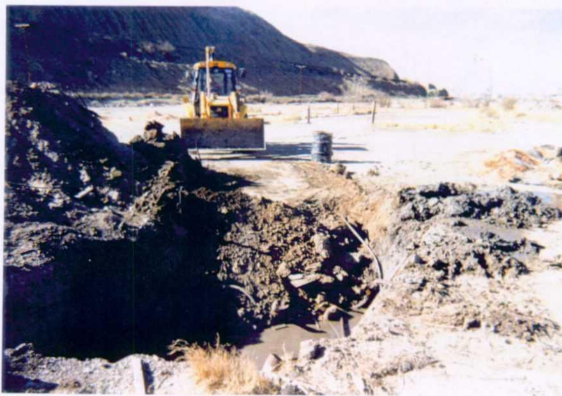
4: View looking northwest at groundwater in tankhold.
