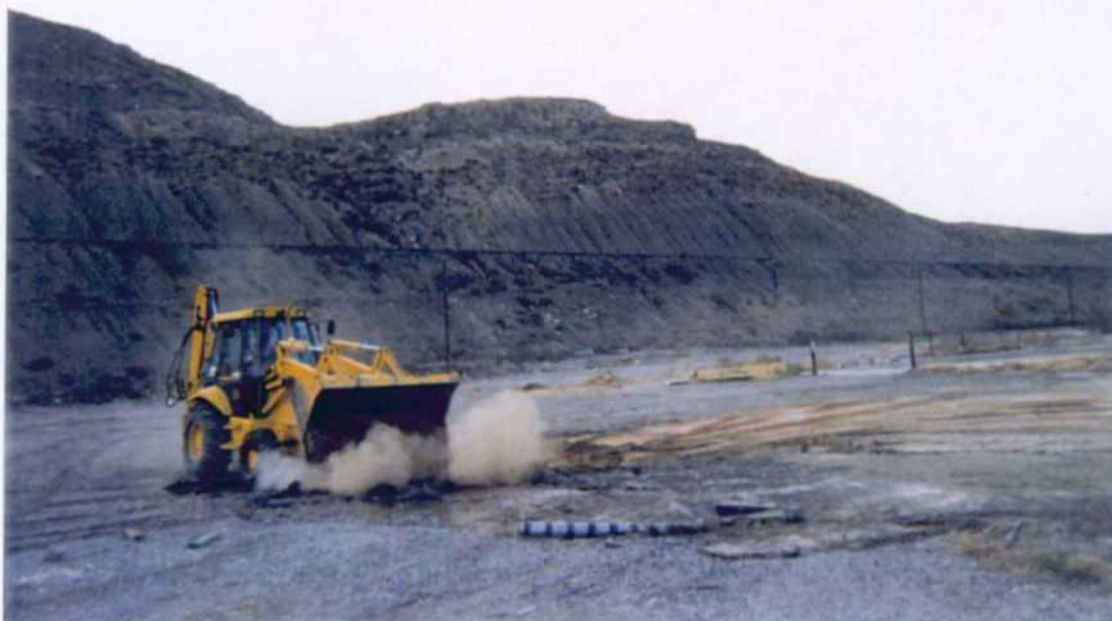
12: Sump tankhold is backfilled and wheel rolled.
