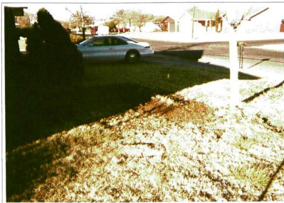
Trenching to the North in Front Yard at 1331 Tasker Road
