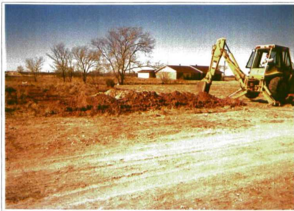
Trenching North on West Side of Alley
