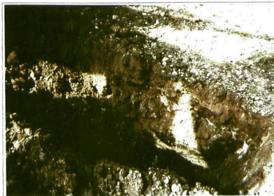
Tasker Road Trench at SS #2
