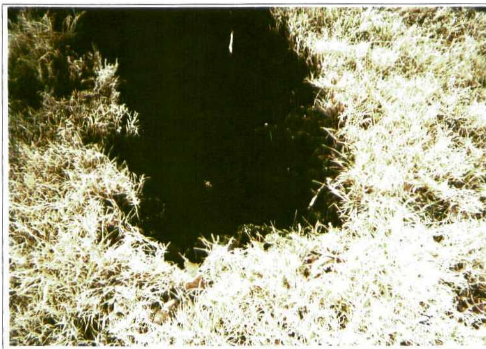
Tasker Road Trench - SS #3 at 2'
