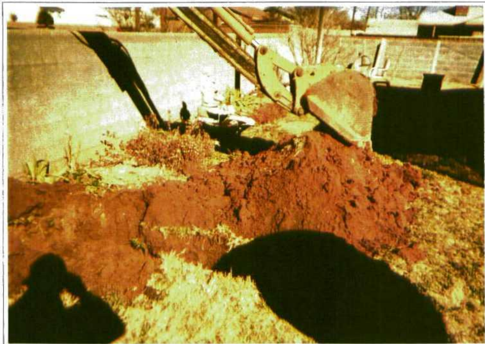
Trenching to the North in Backyard at 1331 Tasker Road
