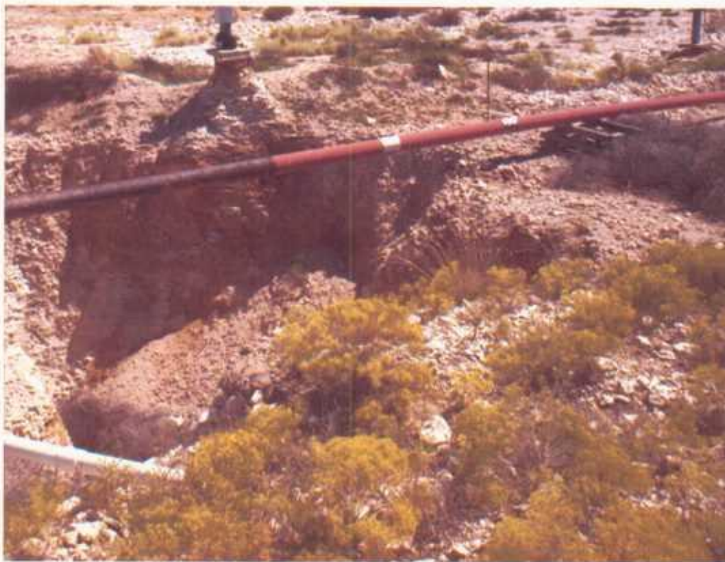
Looking Southeast toward South sidewall of deep excavation
