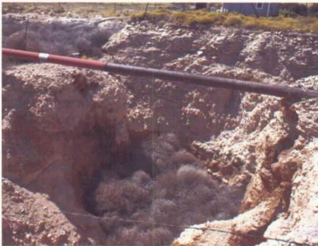
Looking West toward West Sidewall of Deep Excavation
