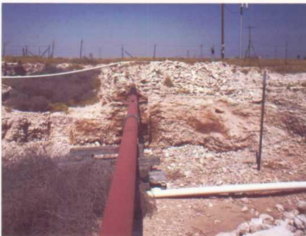
Looking North, deep excavation in photo center
