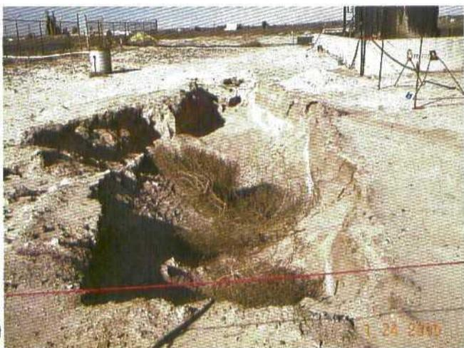
View facing north showing area of line leak located near the southwest corner of a tank battery and approx. 50 feet east of lined pond on Dynegy plant property.
