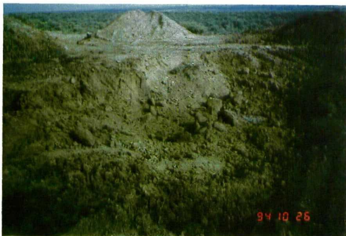
#4 VIEW TO NE SHOWING PIT EXCAVATION & STOCKPILED SOILS
