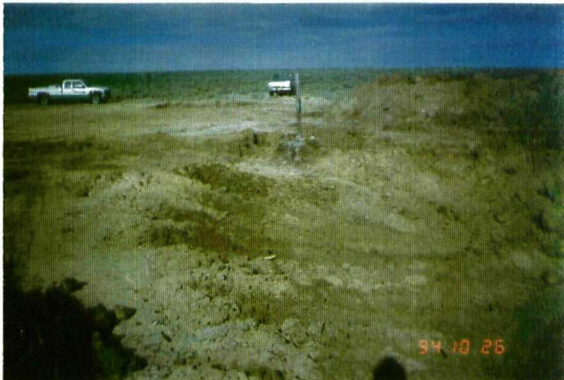
#3 VIEW TO WEST SHOWING WELLHEAD AND EXCAVATION OF PIT
