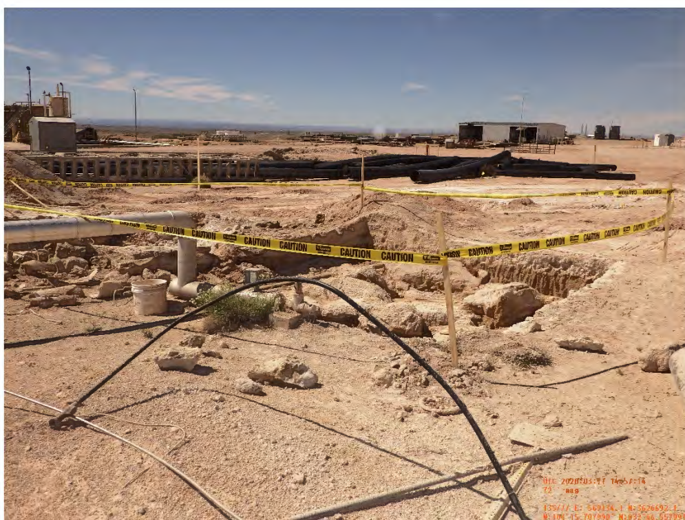
Slop Oil Tanks Excavation EA-05-01 Viewing Northwest, March 25, 2020
