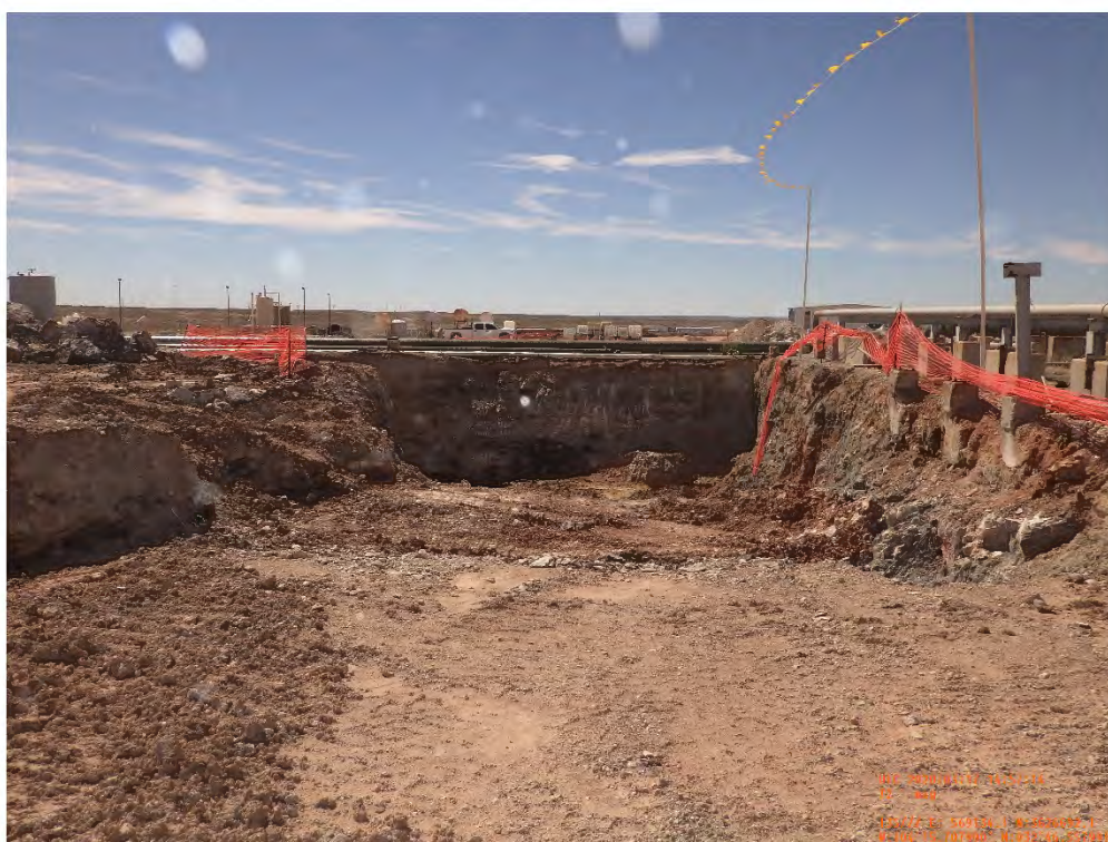
Clark Building (EA-12) Excavation (C-10 – C-12) Viewing South, March 25, 2020
