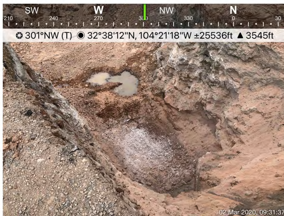
Clark Building (EA-12) Sidewall Seepage Excavation (C-12), March 2, 2020
