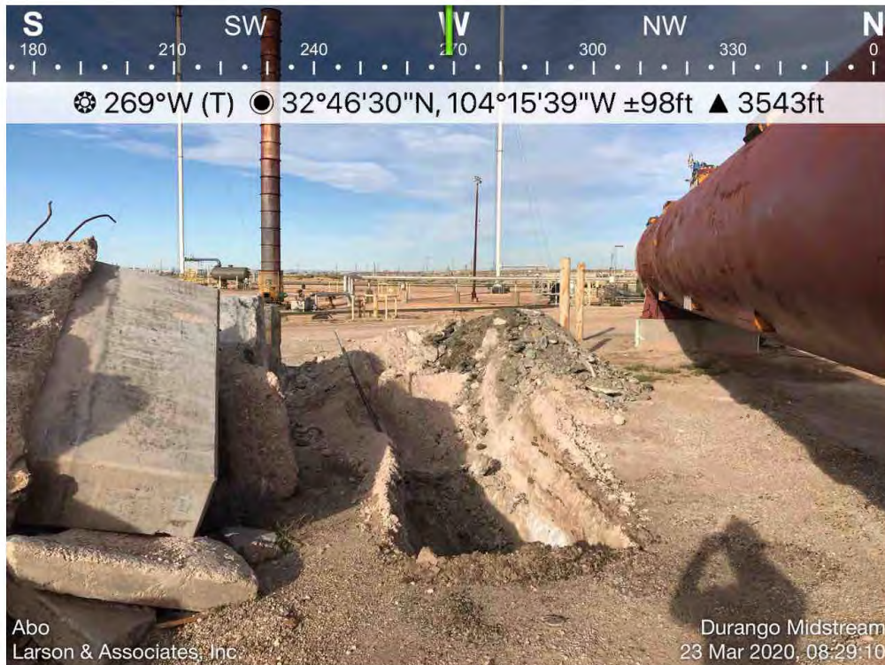
Area North of Engine 9 (EA-14) Building (S-11) Viewing West, March 23, 2020
