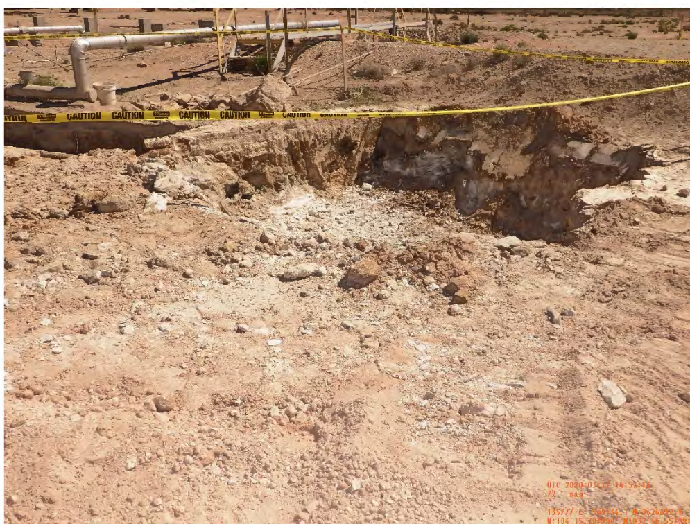
Slop Oil Tanks Excavation EA-05-02 Viewing Northwest, March 25, 2020
