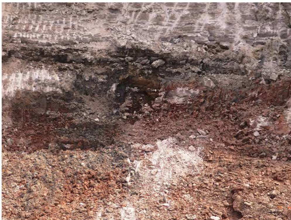
Clark Building (EA-12) South Sidewall Seepage Excavation (C-12), February 28, 2020
