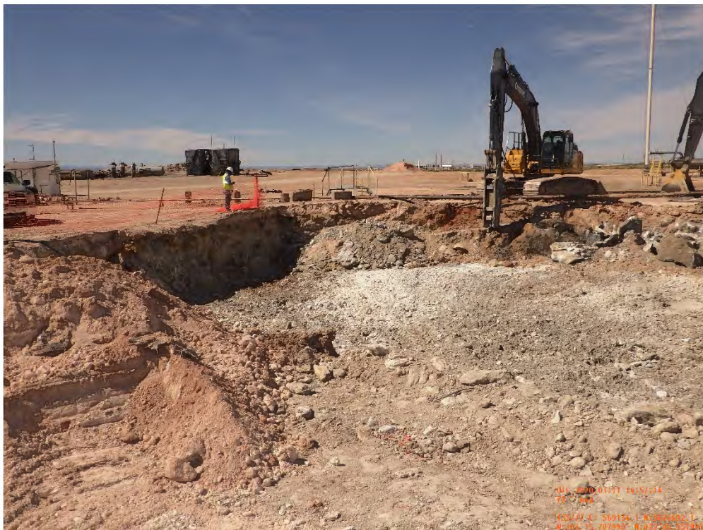
Engine 9 Building (EA-13) Excavation Viewing Northwest, March 25, 2020
