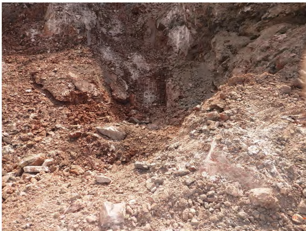
Clark Building (EA-12) Excavation (C-10) Viewing West, February 28, 2020
