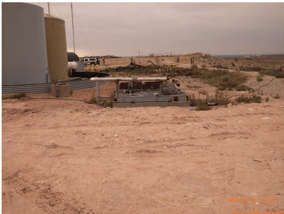
Amine Sump Viewing South
