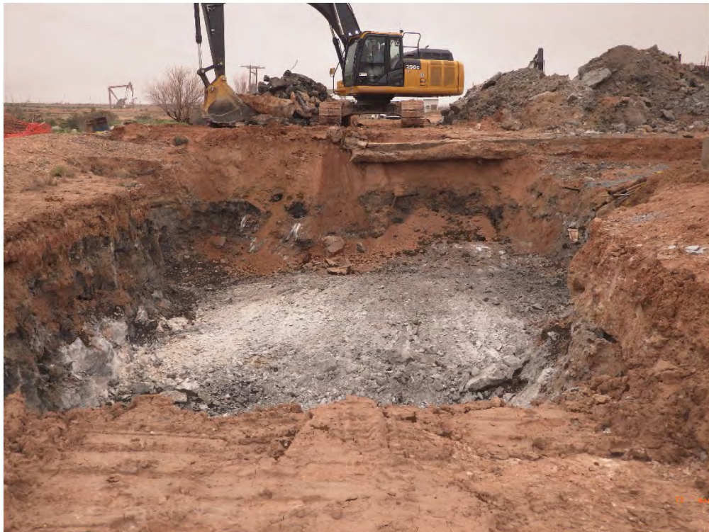
Amine Sump Excavation Viewing North, March 17, 2020
