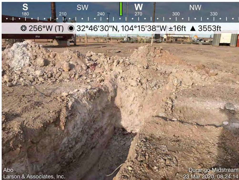
Area North of Engine 9 (EA-14) Building (S-5B) Viewing West, March 23, 2020
