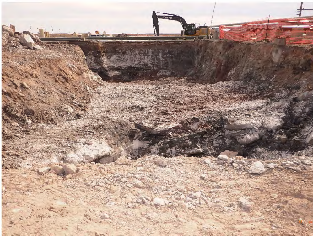
Clark Building (EA-12) Excavation (C-10) Viewing South, February 28, 2020
