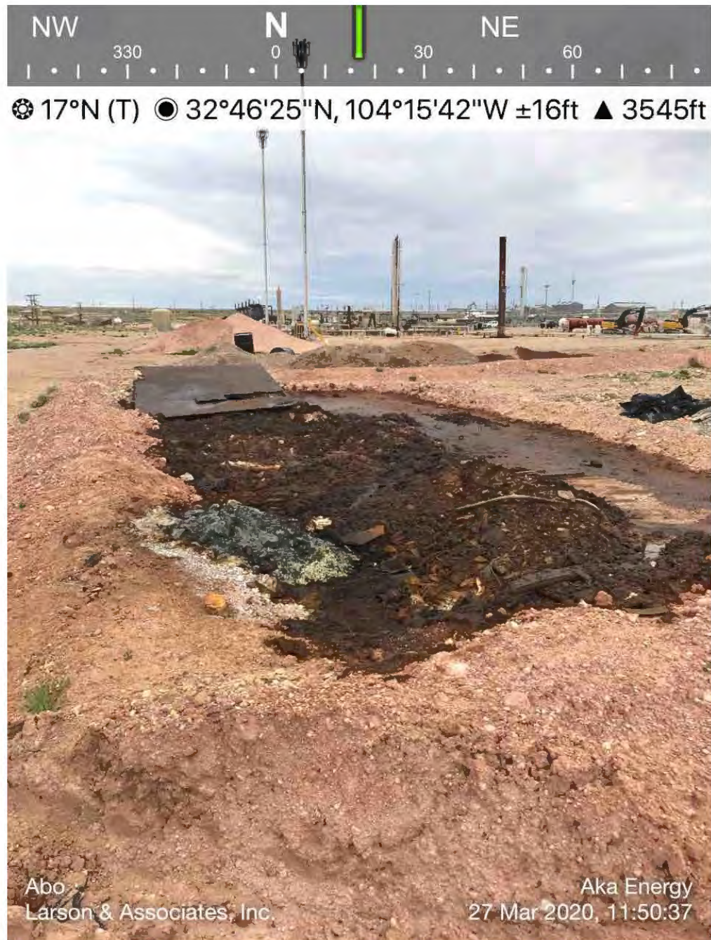
West Containment (EA-15) Viewing North, March 27, 2020
