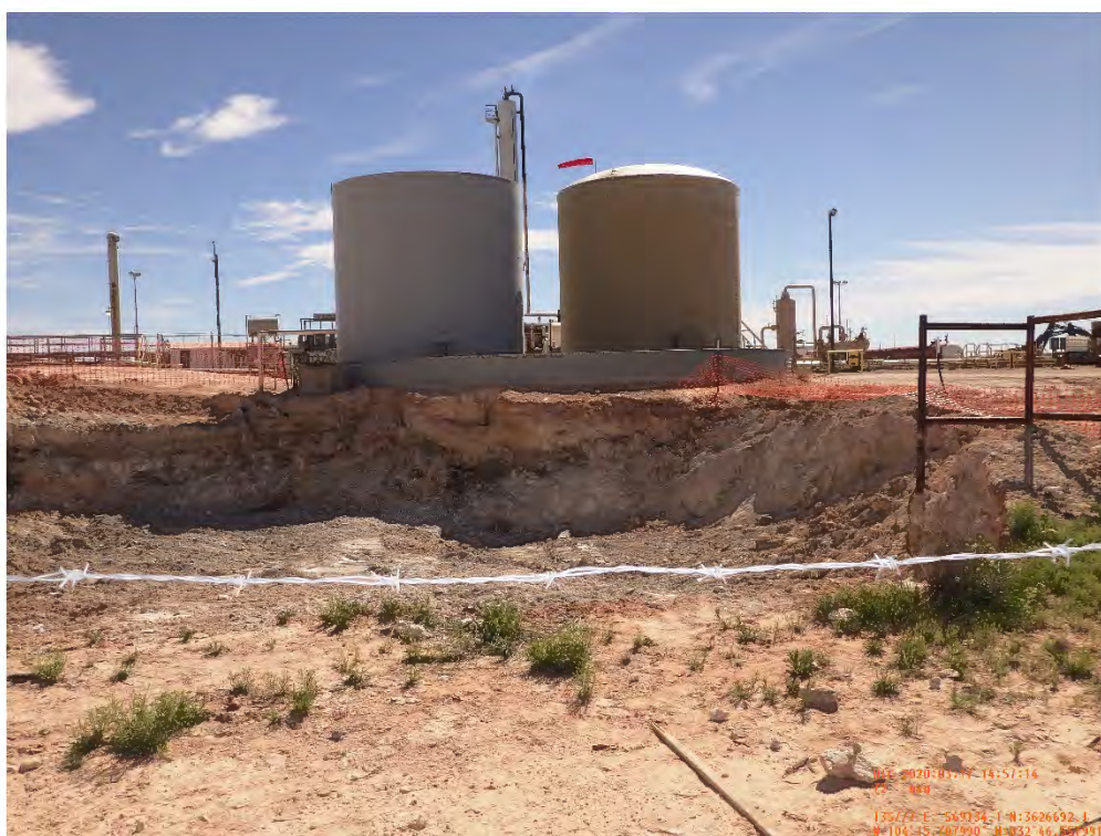
Amine Sump Excavation Viewing East, March 25, 2020
