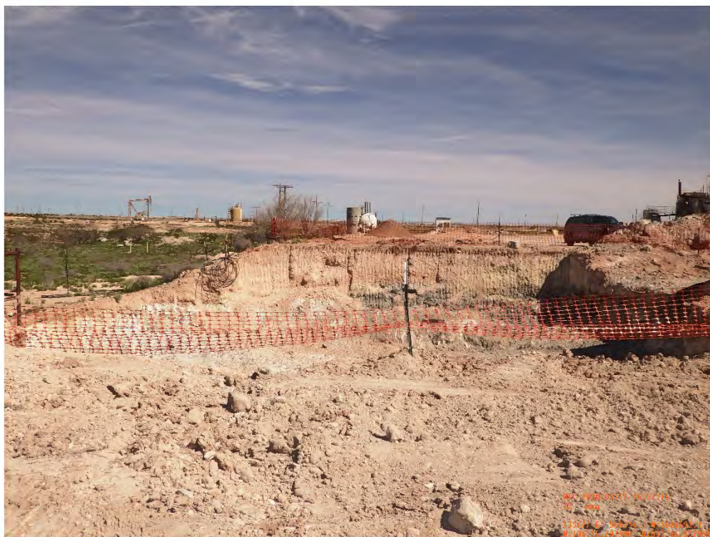
Amine Sump Excavation Viewing North, March 25, 2020
