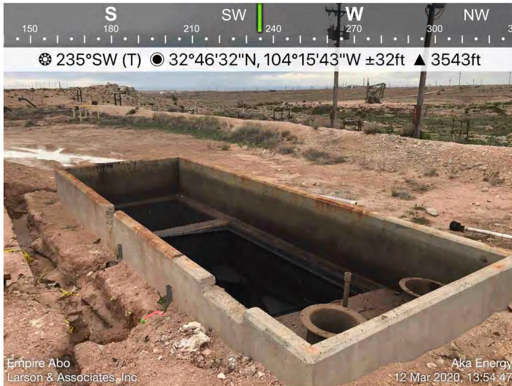
Amine Sump Viewing Southeast, March 12, 2020
