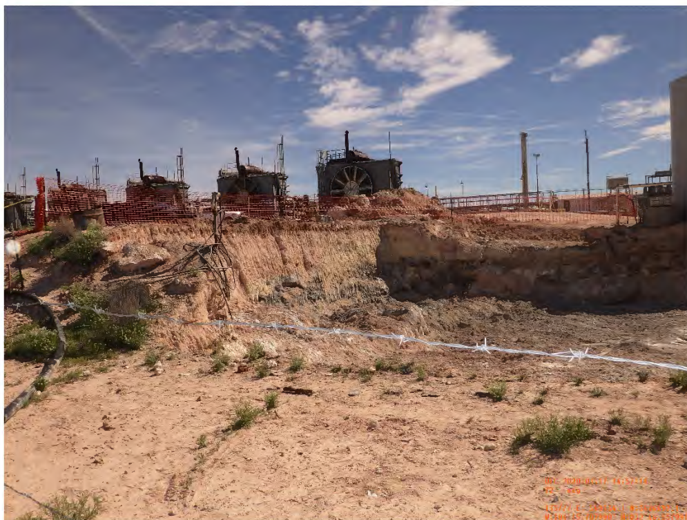
Amine Sump Excavation Viewing Northeast, March 25, 2020
