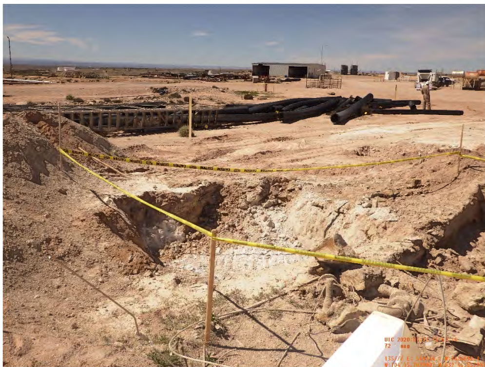
Slop Oil Tanks Excavation EA-05-03 Viewing Southeast, March 25, 2020
