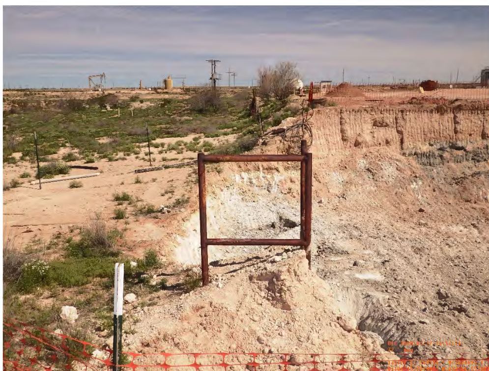
Amine Sump Excavation (West Side) Viewing North, March 25, 2020
