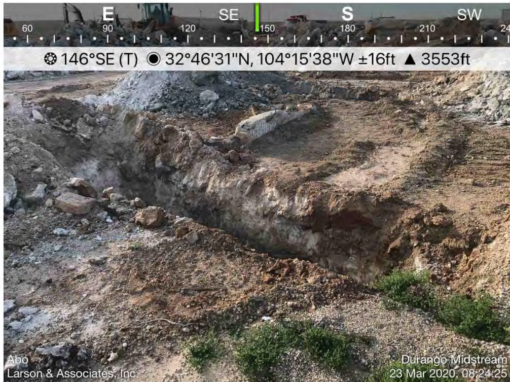
Area North of Engine 9 (EA-14) Building (S-10) Viewing Southwest, March 23, 2020
