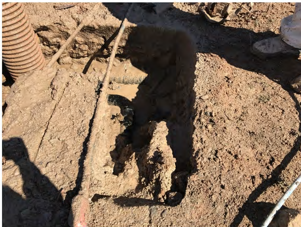
Slop Oil Tanks Hydroexcavating Location EA-05-01, March 8, 2020
