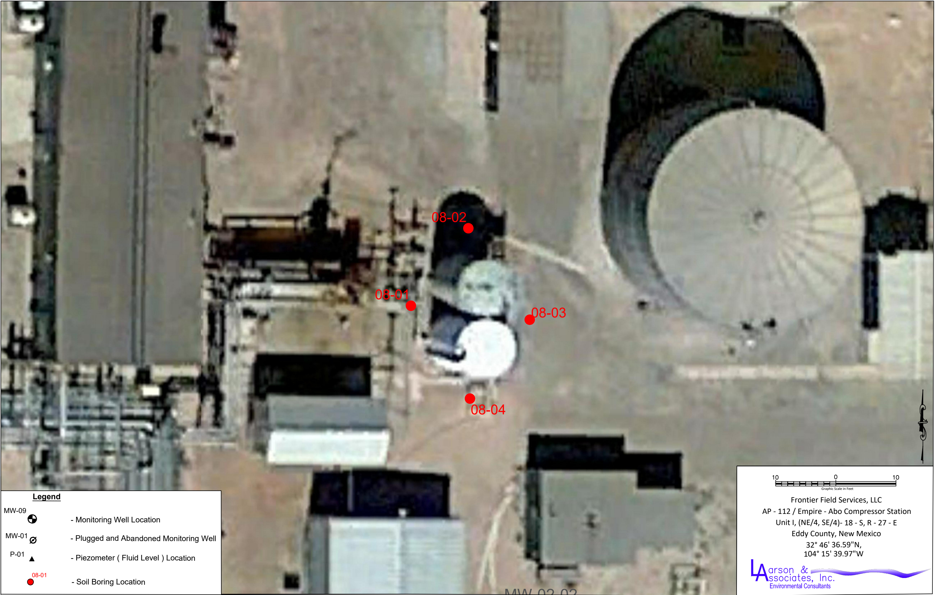
Figure 3e - Lube Oil Tank (EA-08)
