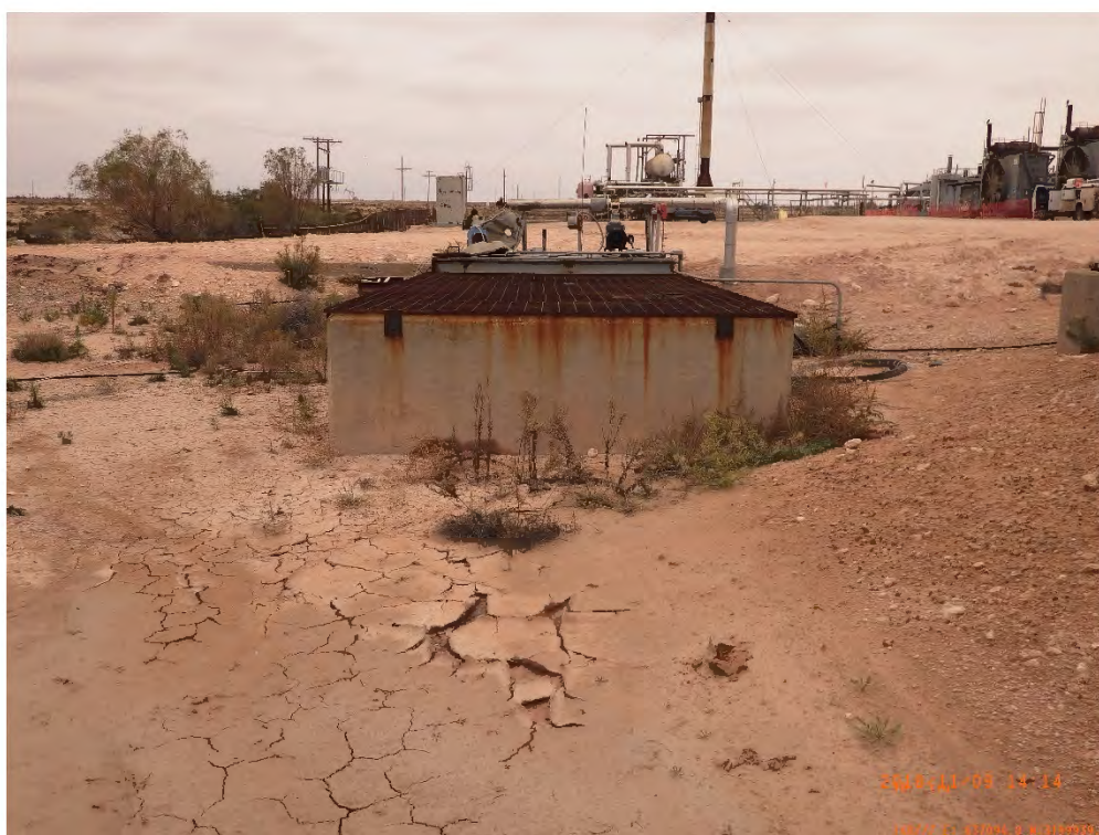
Amine Sump Viewing North
