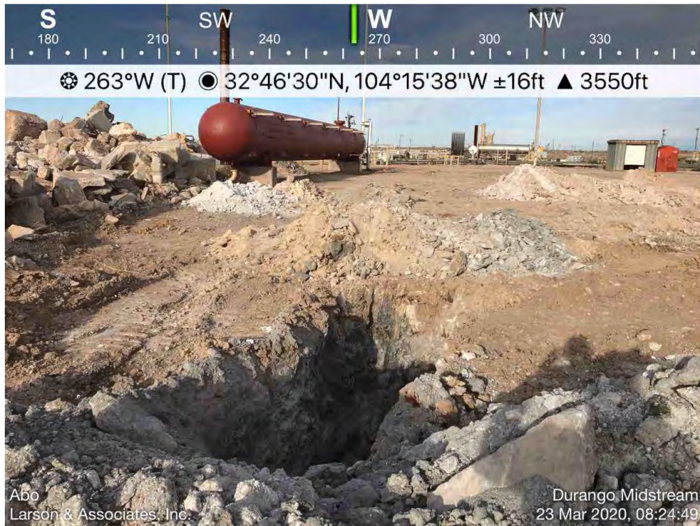
Area North of Engine 9 (EA-14) Building (S-4B) Viewing West, March 23, 2020
