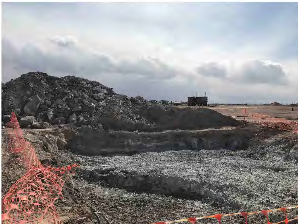
Engine 9 Building (EA-13) Excavation Viewing South, February 25, 2020
