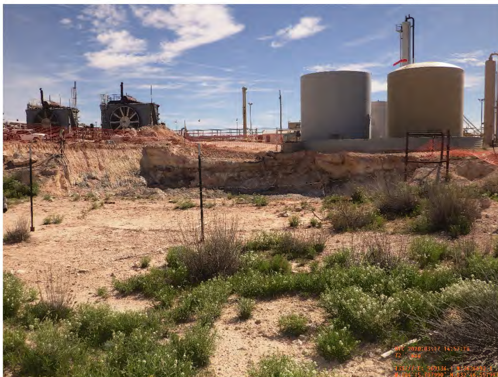
Amine Sump Excavation Viewing North, March 25, 2020
