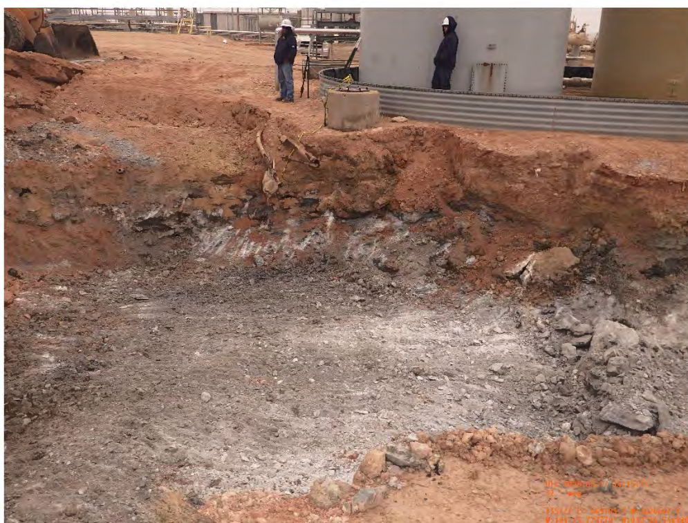
Amine Sump Excavation Viewing East, March 17, 2020
