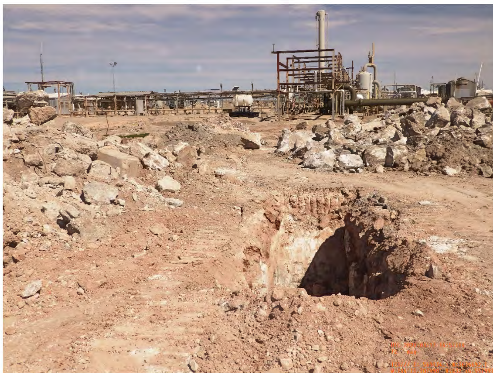
Area North of Engine 9 (EA-14) Building (S-8) Viewing North, March 25, 2020
