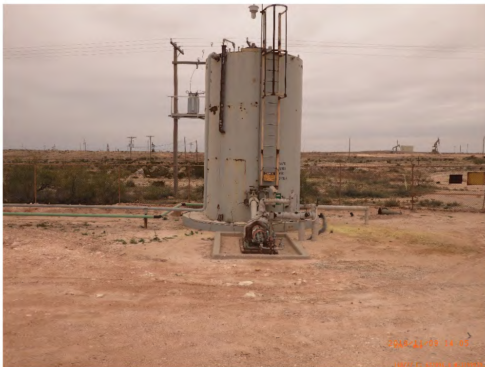
Wastewater Tank Viewing West
