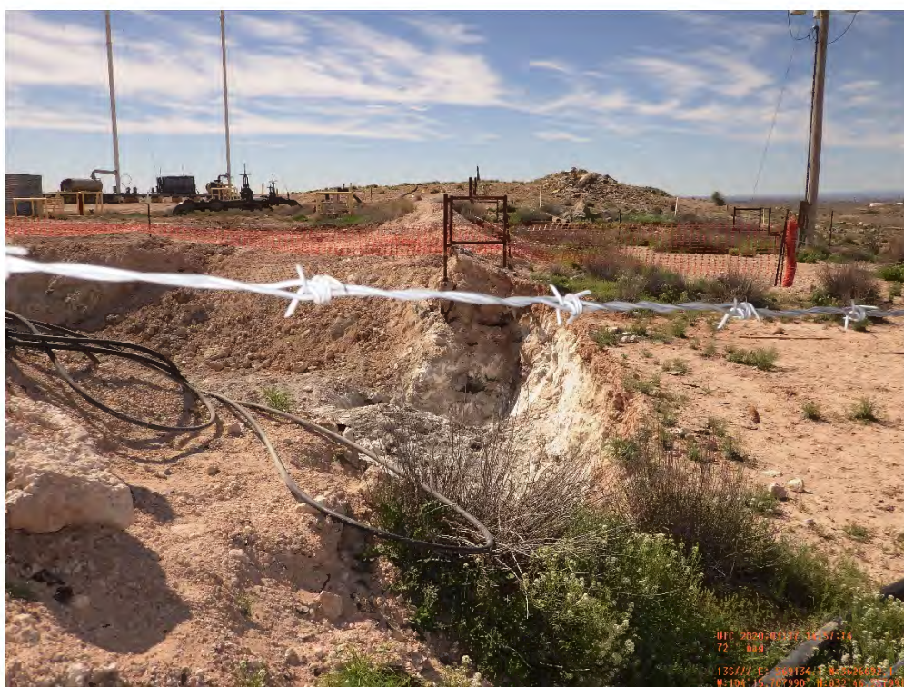
Amine Sump Excavation (West Side) Viewing South, March 25, 2020
