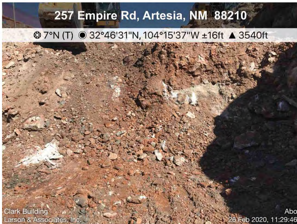
In-Situ Soil at Clark Building (EA-12) Viewing South, February 26, 2020
