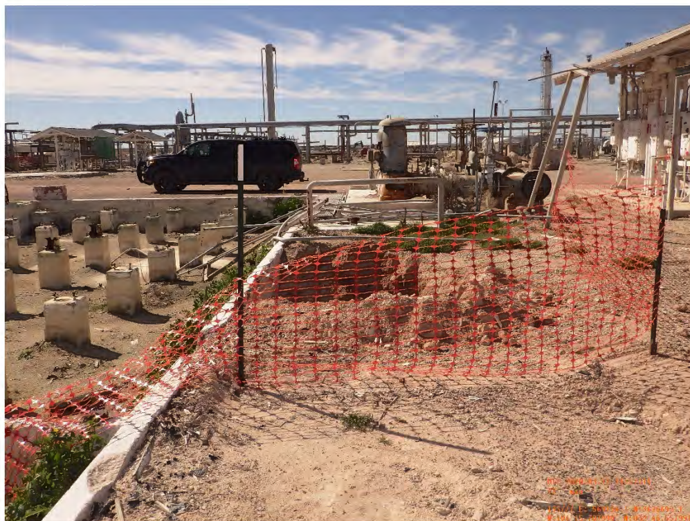
Cooling Tower Excavation EA-07-05 Viewing South, March 25, 2020
