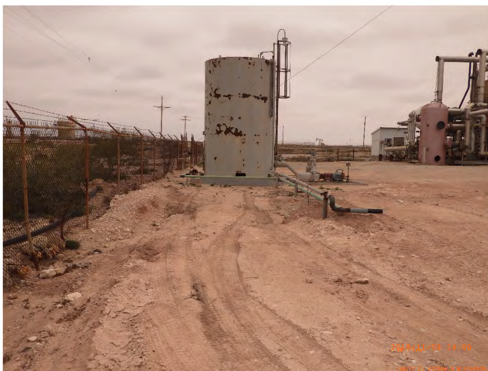
Wastewater Tank Viewing North
