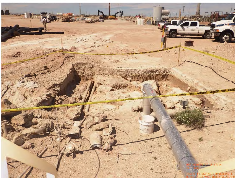
Slop Oil Tanks Excavation EA-05-01 Viewing West, March 25, 2020
