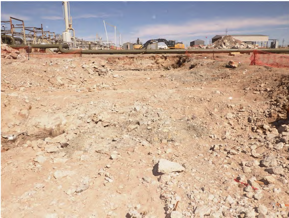
Clark Building (EA-12) Excavation (C-13 – C-14) Viewing North, February 28, 2020
