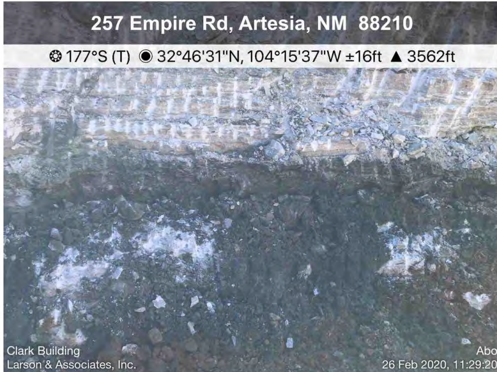
Excavated Soil at Clark Building (EA-12) Viewing South, February 26, 2020
