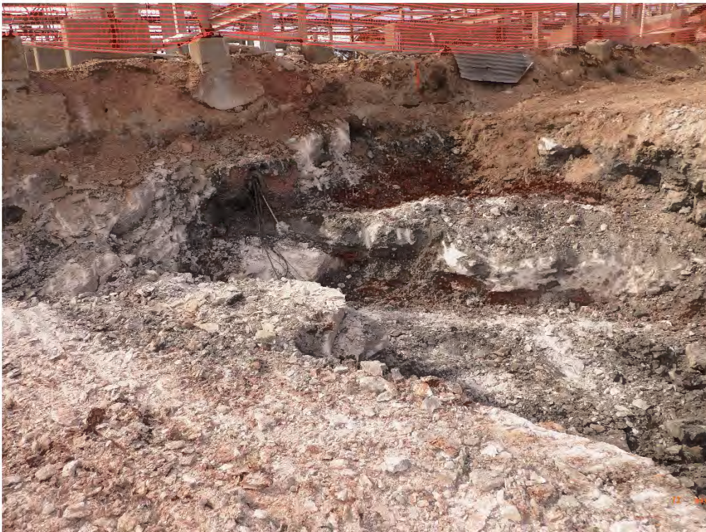
Clark Building (EA-12) Excavation (C-10) Viewing Northwest, February 28, 2020
