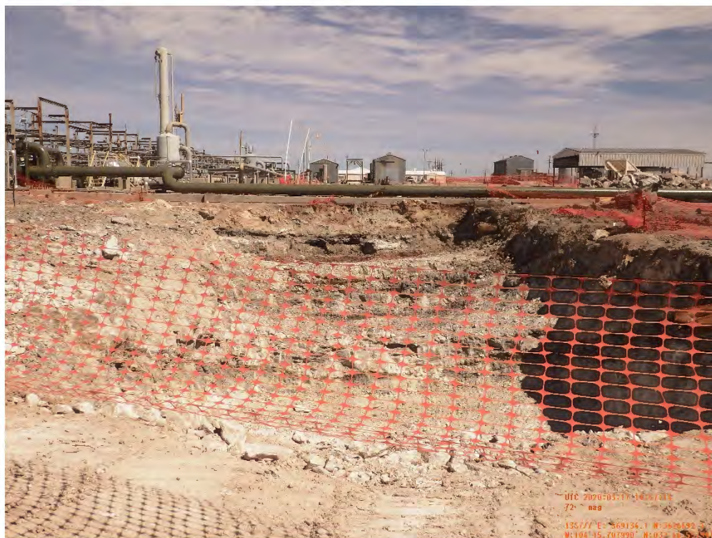
Clark Building (EA-12) Excavation (C-13 and C-14) Viewing North, March 25, 2020
