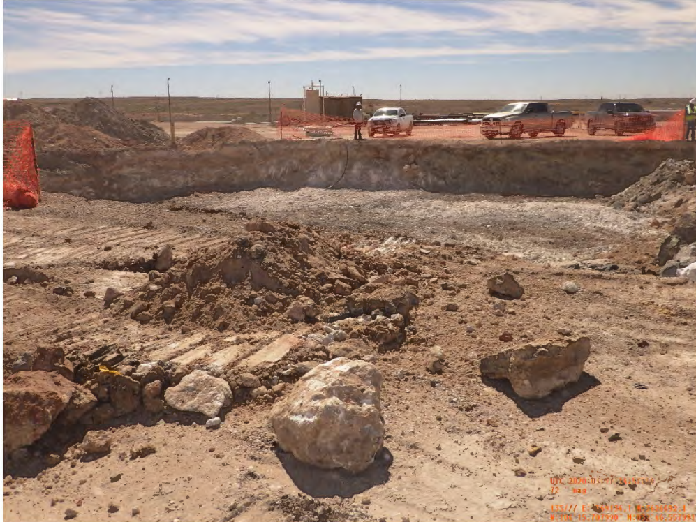
Engine 9 Building (EA-13) Excavation Viewing South, March 25, 2020
