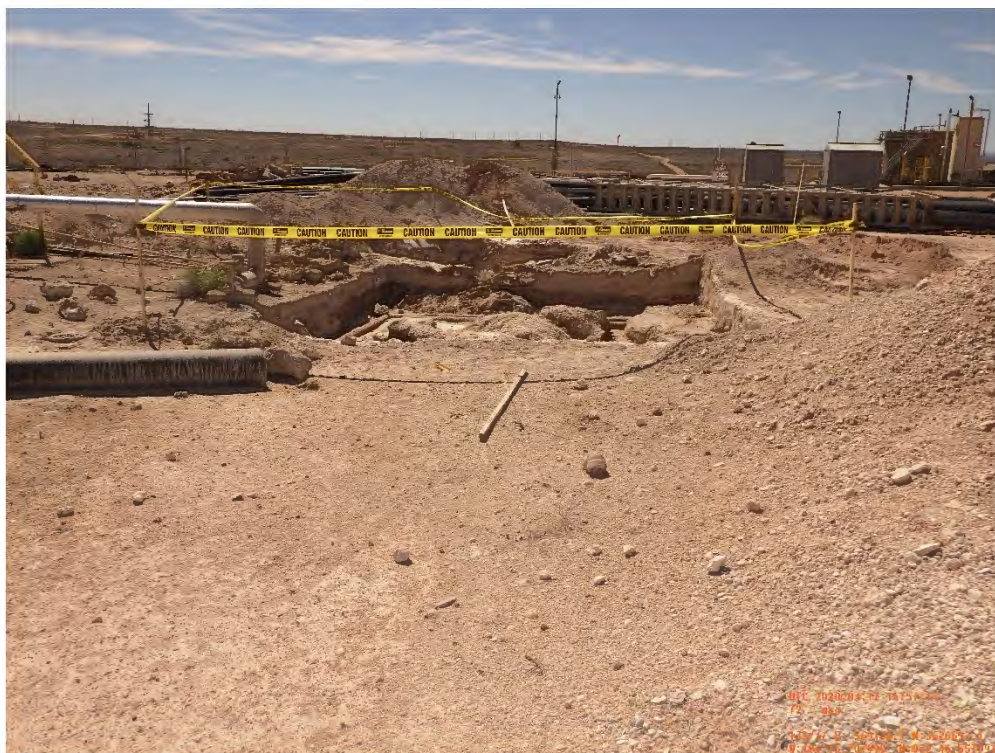
Slop Oil Tanks Excavation EA-05-01 Viewing South, March 25, 2020
