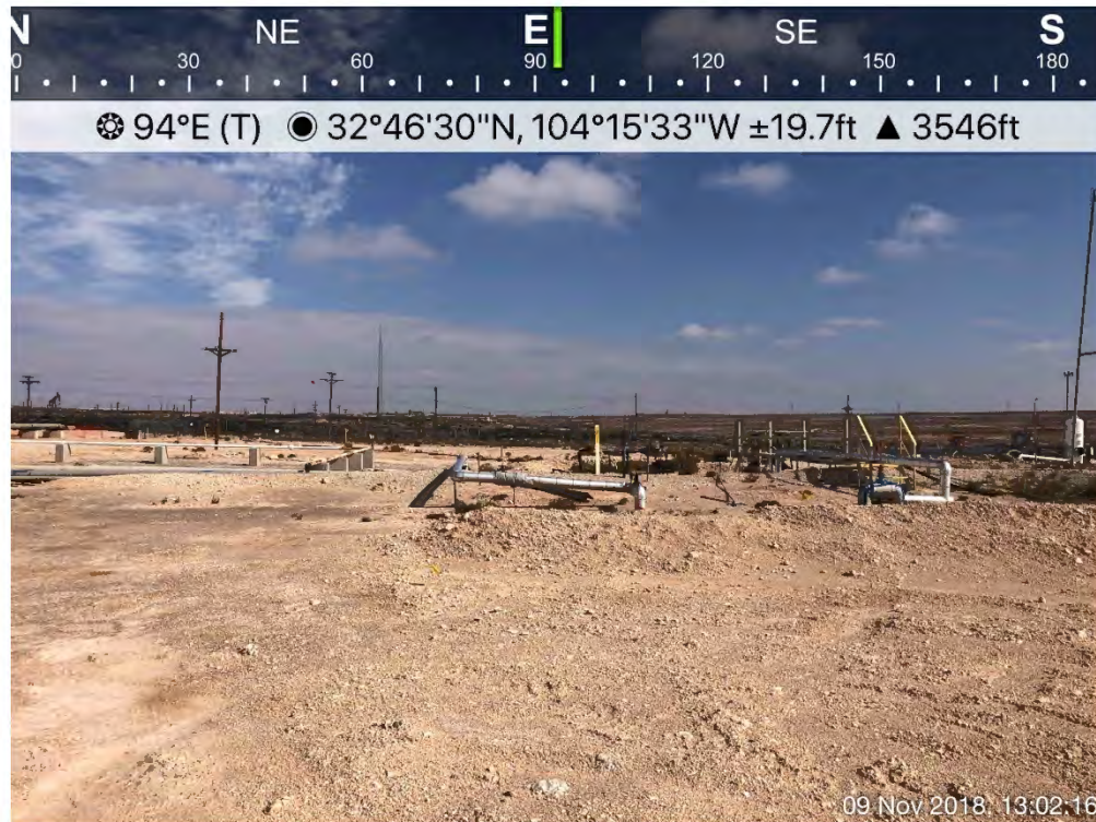
Slop Oil Tanks Location Viewing East
