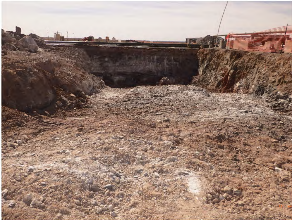
Clark Building (EA-12) Excavation (C-10 – C-12) Viewing South, February 28, 2020
