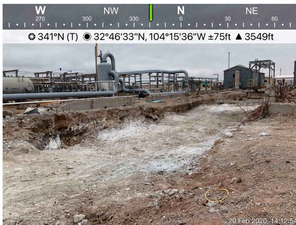
Clark Building (EA-12) Excavation (C-2 - C-4) Viewing Northwest, February 20, 2020
