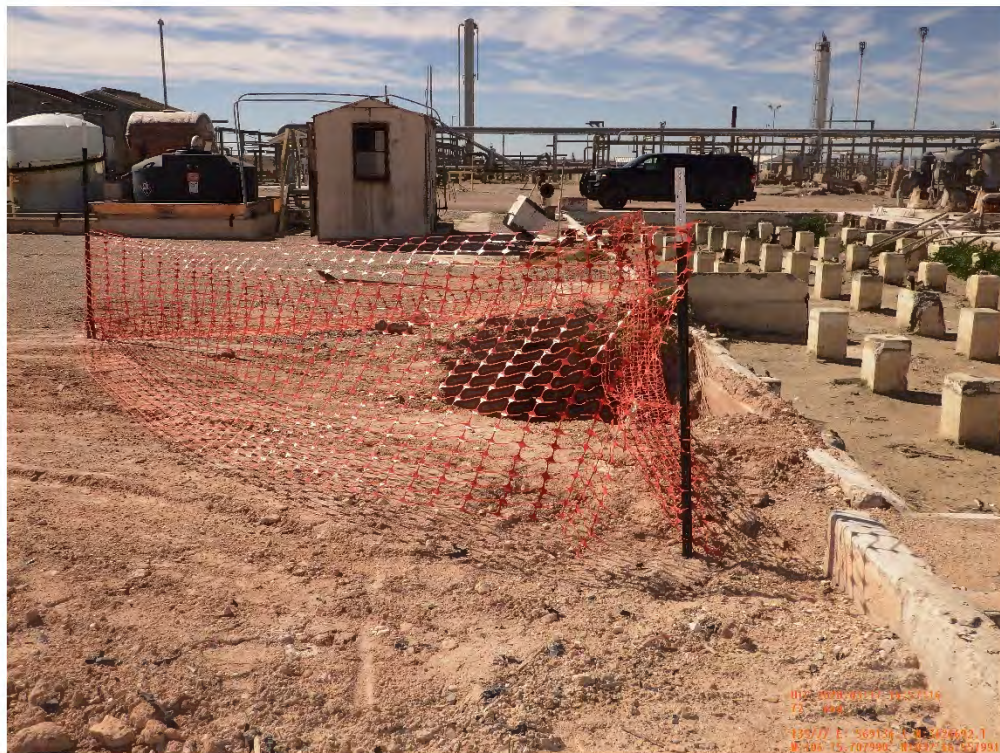
Cooling Tower Excavation EA-07-02 Viewing South, March 25, 2020
