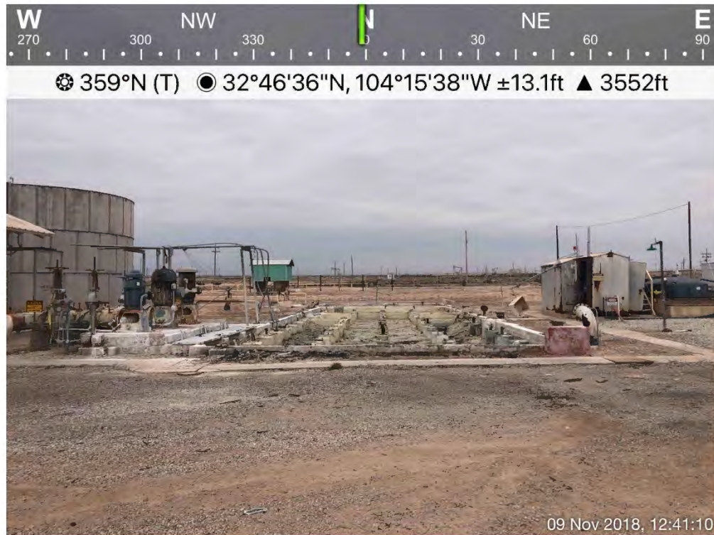
Cooling Tower Location Viewing North
