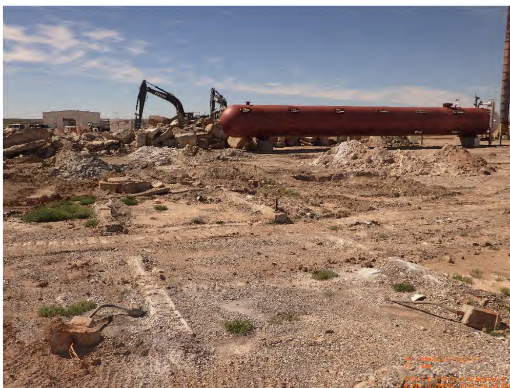
Area North of Engine 9 (EA-14) Building Viewing Southwest, March 25, 2020
