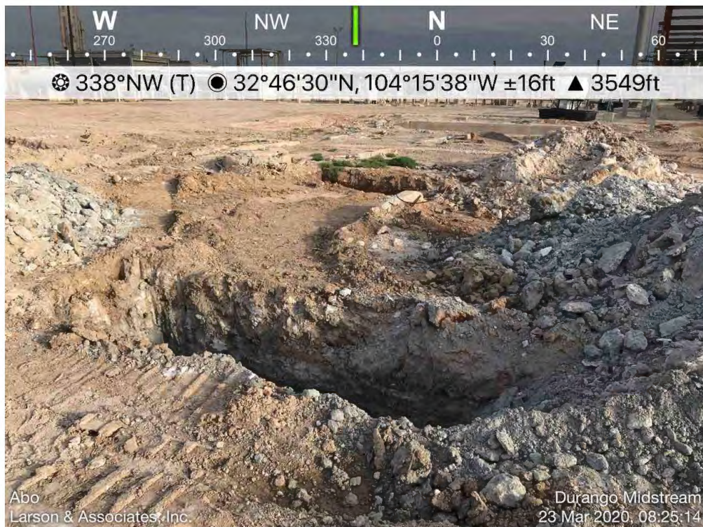
Area North of Engine 9 (EA-14) Building (S-8) Viewing North, March 23, 2020
