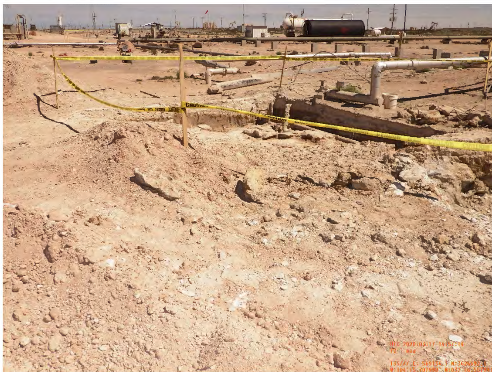
Slop Oil Tanks Excavation EA-05-01 Viewing Northwest, March 25, 2020
