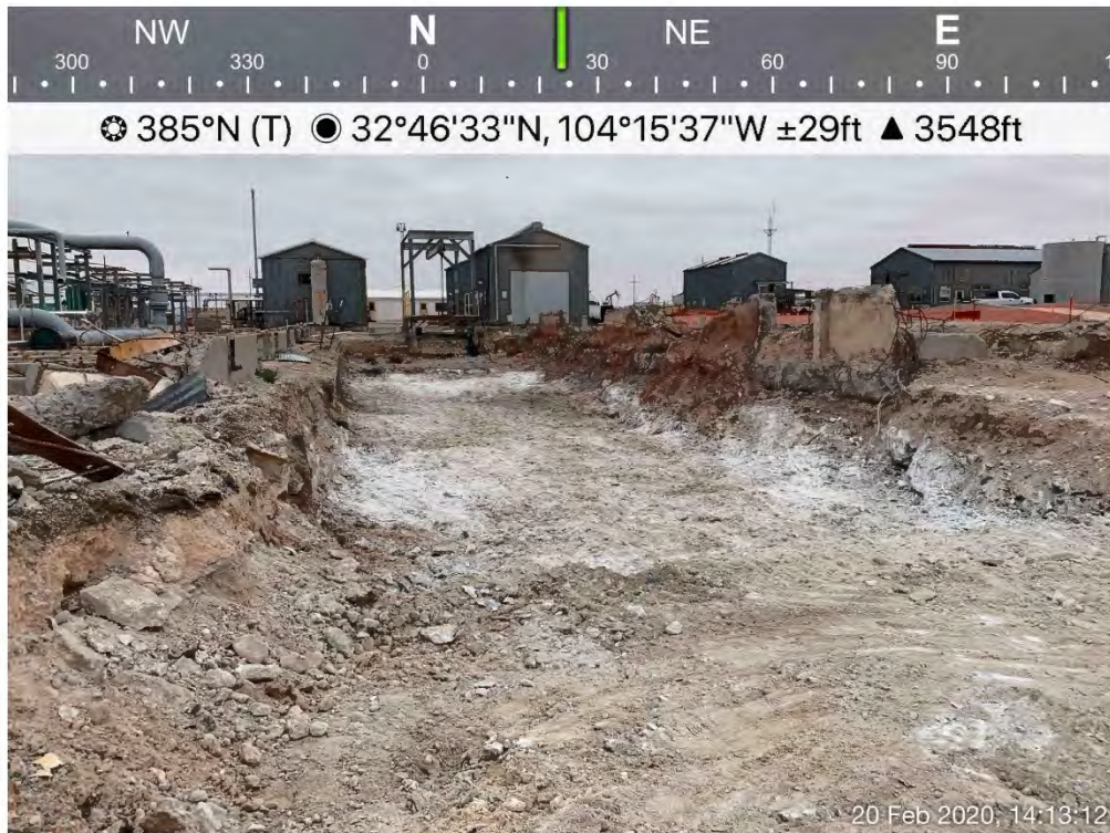
Clark Building (EA-12) Excavation (C-2 - C-4) Viewing North, February 20, 2020
