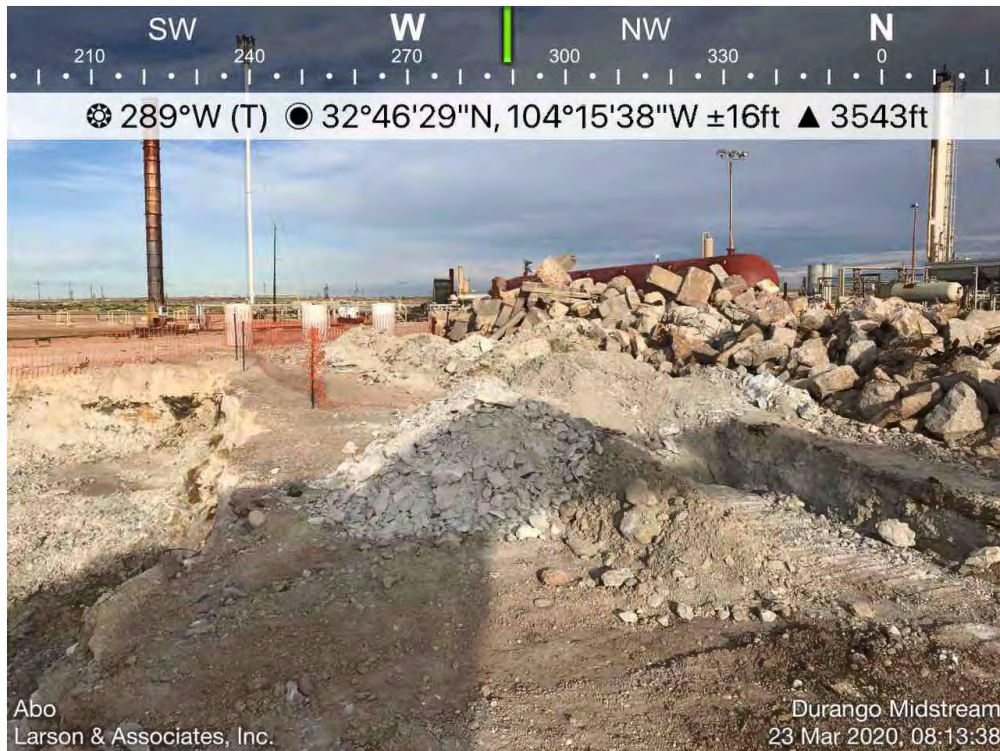
Area North of Engine 9 Building (S-4A) Viewing West, March 23, 2020
