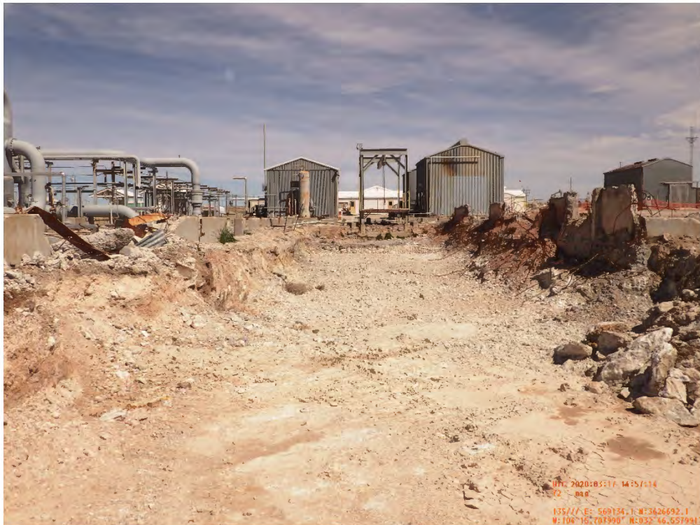
Clark Building (EA-12) Excavation (C-2 – C-4) Viewing North, March 25, 2020
