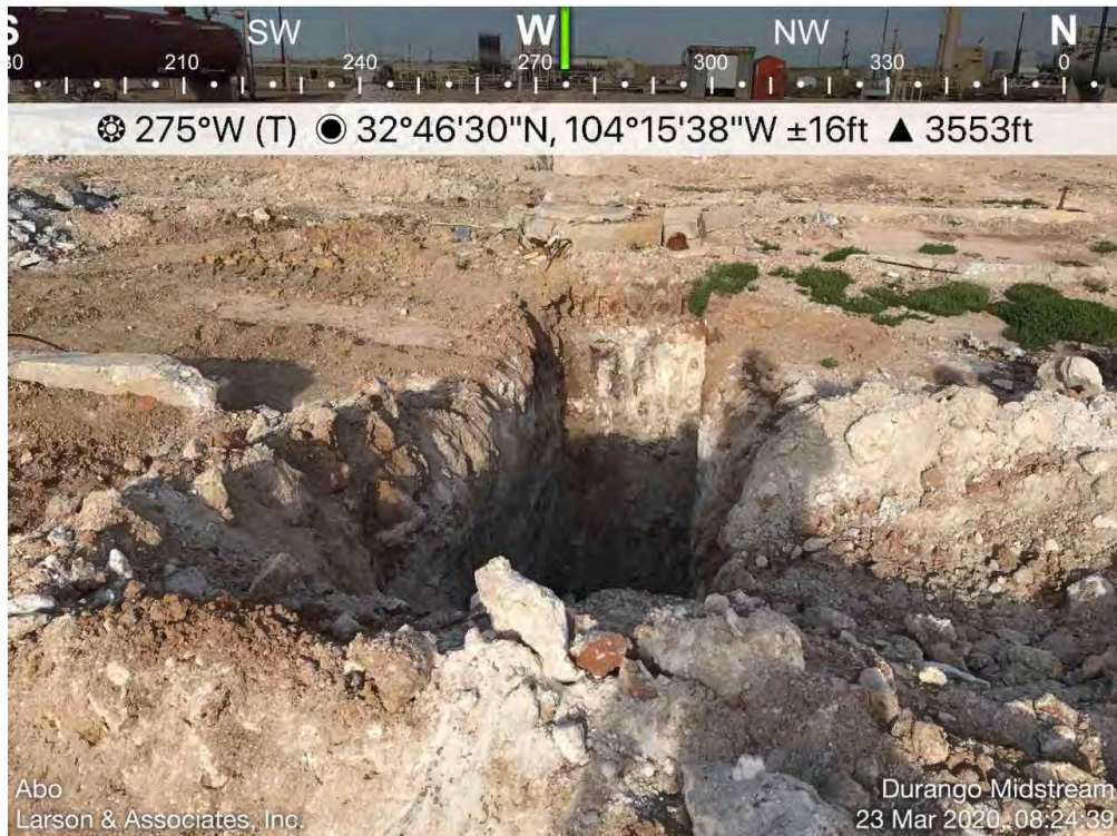
Area North of Engine 9 (EA-14) Building (S-8) Viewing West, March 23, 2020
