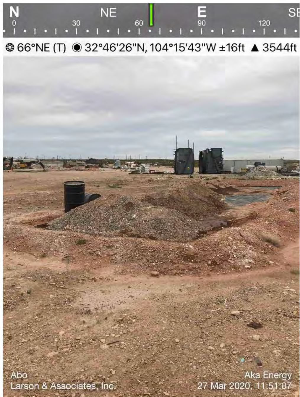
North Containment (EA-15) Viewing Northeast, March 27, 2020
