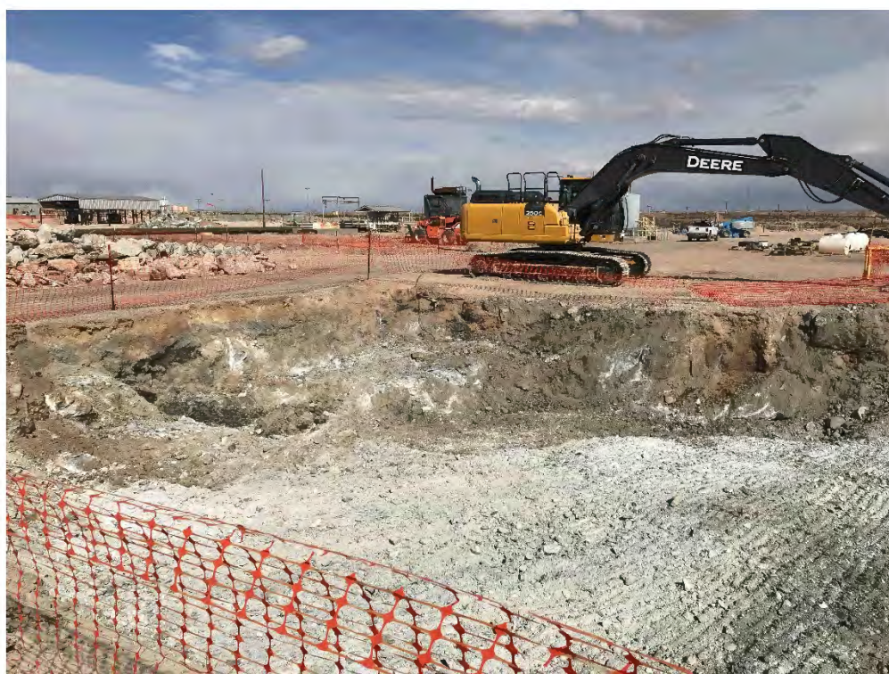
Engine 9 Building (EA-13) Excavation Viewing Northwest, February 25, 2020
