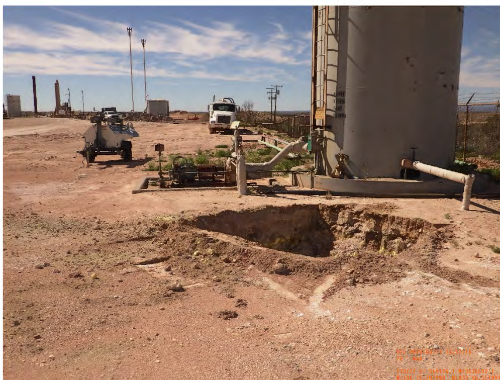
Wastewater Tank Excavation EA-02-03 Viewing South, March 25, 2020
