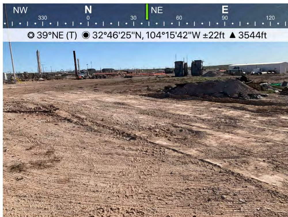
Remediated Containments Viewing Northeast, April 8, 2020
