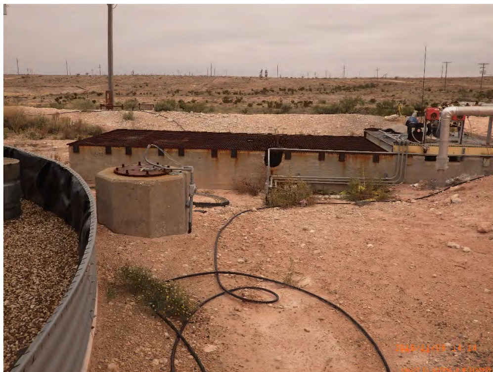
Amine Sump Viewing West
