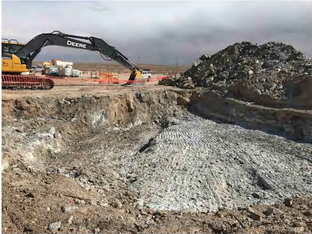
Engine 9 Building (EA-13) Excavation Viewing East, February 25, 2020
