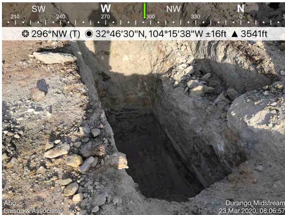
Area North of Engine 9 (EA-14) Building (S-5A), March 23, 2020
