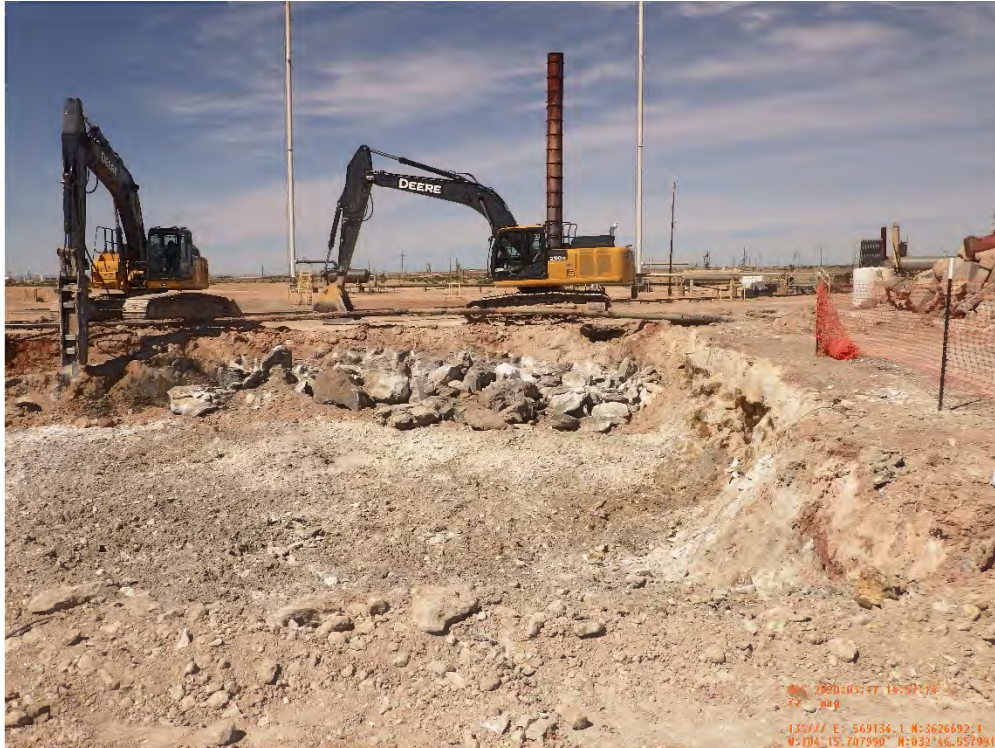
Engine 9 Building (EA-13) Excavation Viewing West, March 25, 2020
