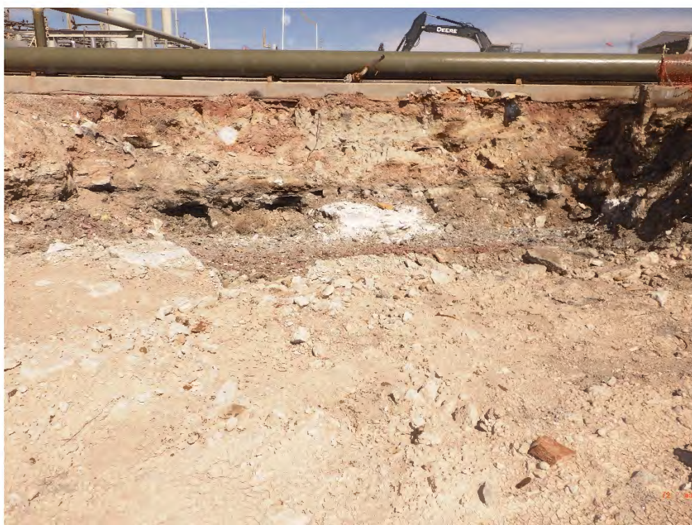
Clark Building (EA-12) Excavation (C-13) Viewing North, February 28, 2020
