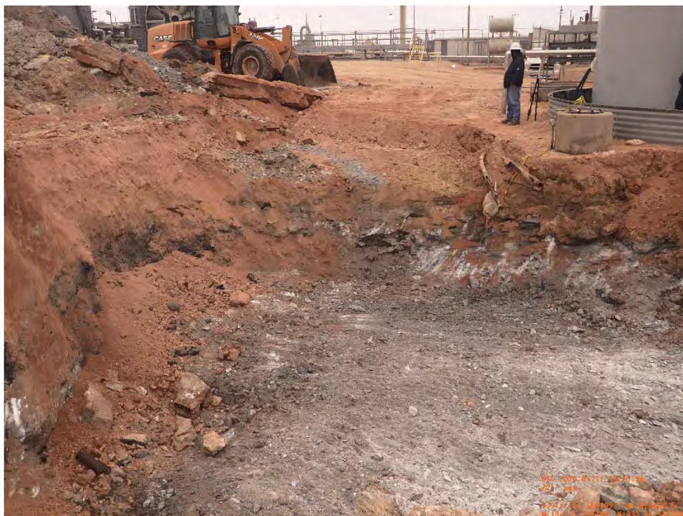
Amine Sump Excavation Viewing Northeast, March 17, 2020
