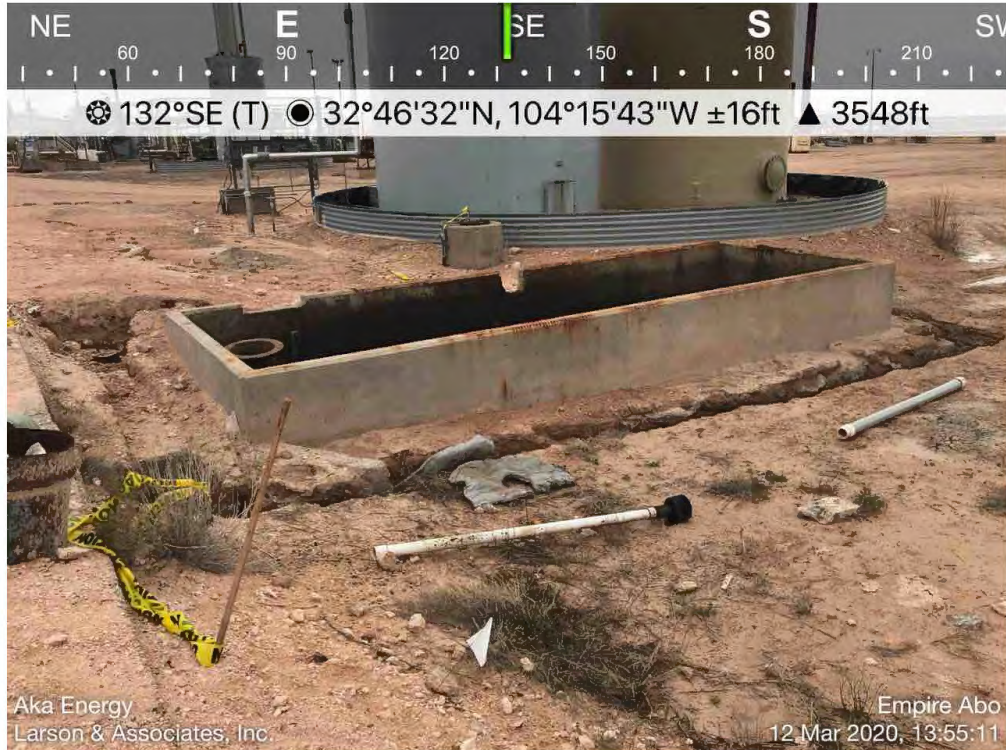
Amine Sump Viewing North, March 12, 2020
