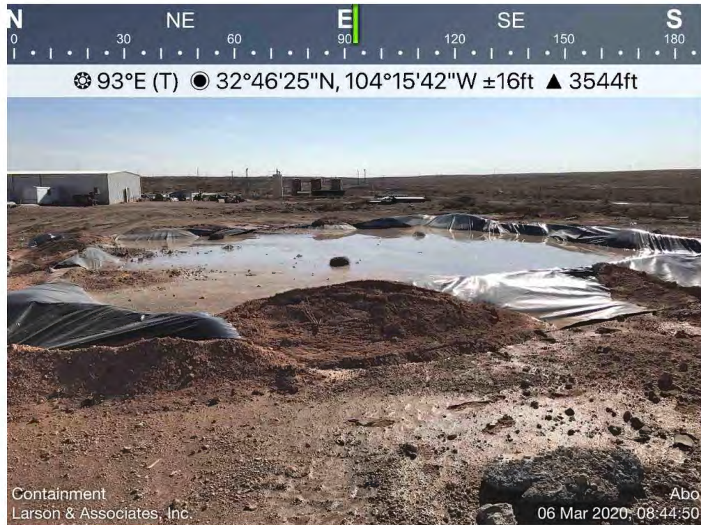
Hydrovac Containment (EA-15) Viewing East, March 6, 2020
