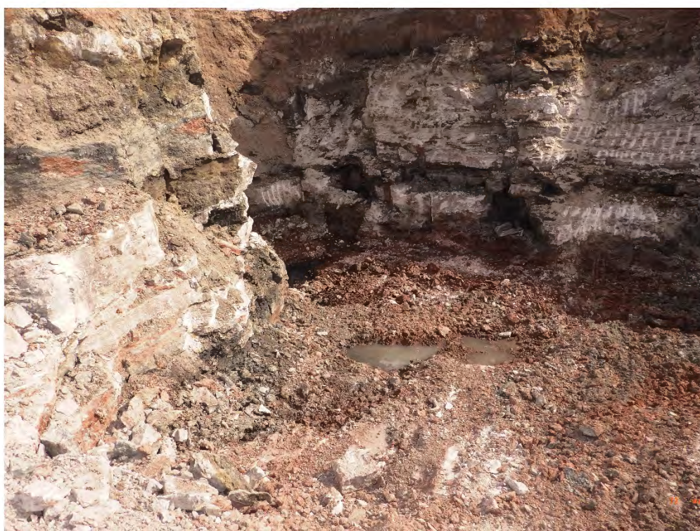
Clark Building (EA-12) East Sidewall Seepage Excavation (C-12), February 28, 2020
