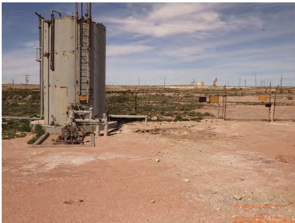
Wastewater Tank Excavation EA-02-03 Viewing West, March 25, 2020
