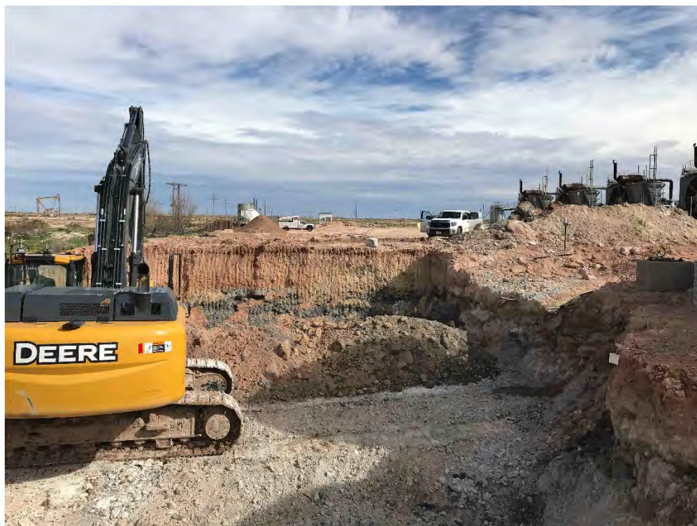
Amine Sump Excavation Viewing North, March 23, 2020
