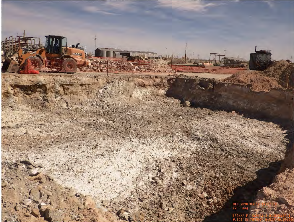
Engine 9 Building (EA-13) Excavation Viewing Northeast, March 25, 2020
