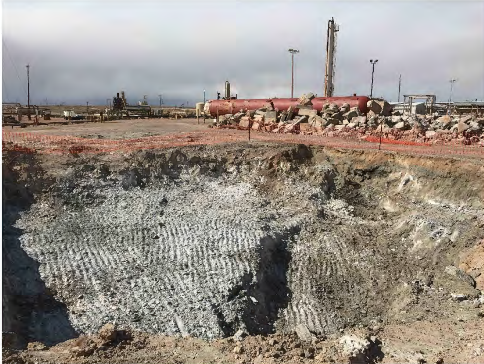
Engine 9 Building (EA-13) Excavation Viewing West, February 25, 2020
