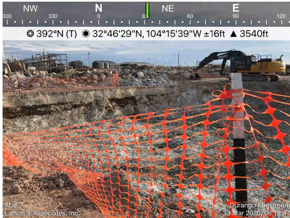
Engine 9 Building (EA-13) Excavation Viewing Southwest, March 23, 2020
