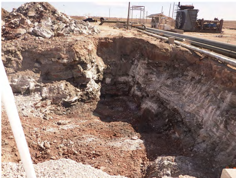
Clark Building (EA-12) Excavation (C-12) Viewing East, February 28, 2020
