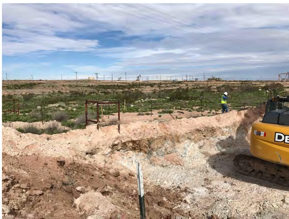
Amine Sump Excavation Viewing Northwest, March 17, 2020
