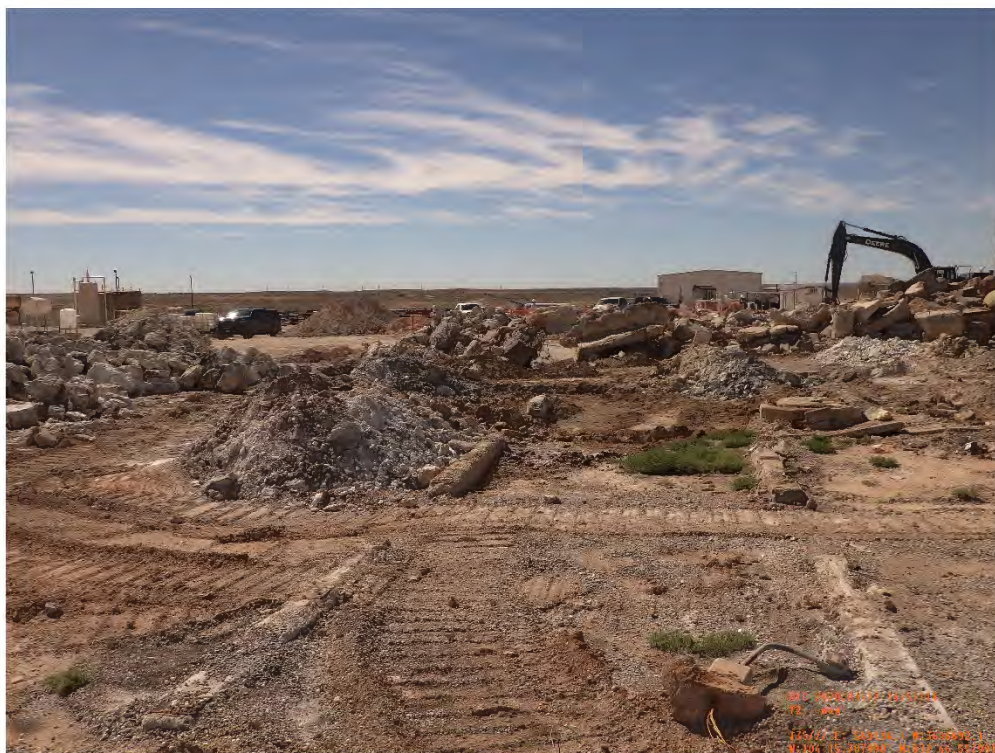
Area North of Engine 9 (EA-14) Building Viewing South, March 25, 2020
