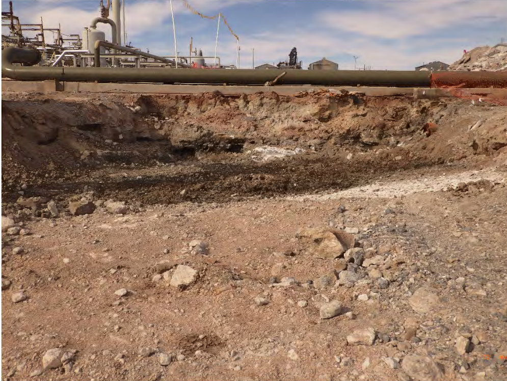
Clark Building (EA-12) Excavation (C-13) Viewing North, February 28, 2020
