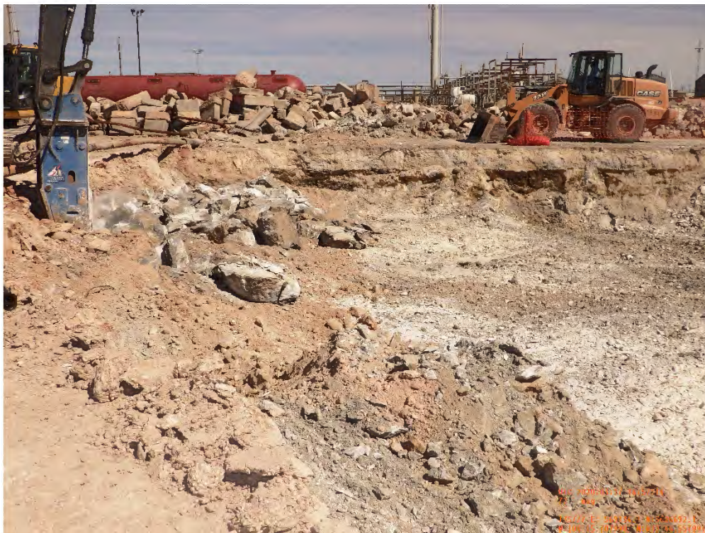
Engine 9 Building (EA-13) Excavation Viewing North, March 25, 2020
