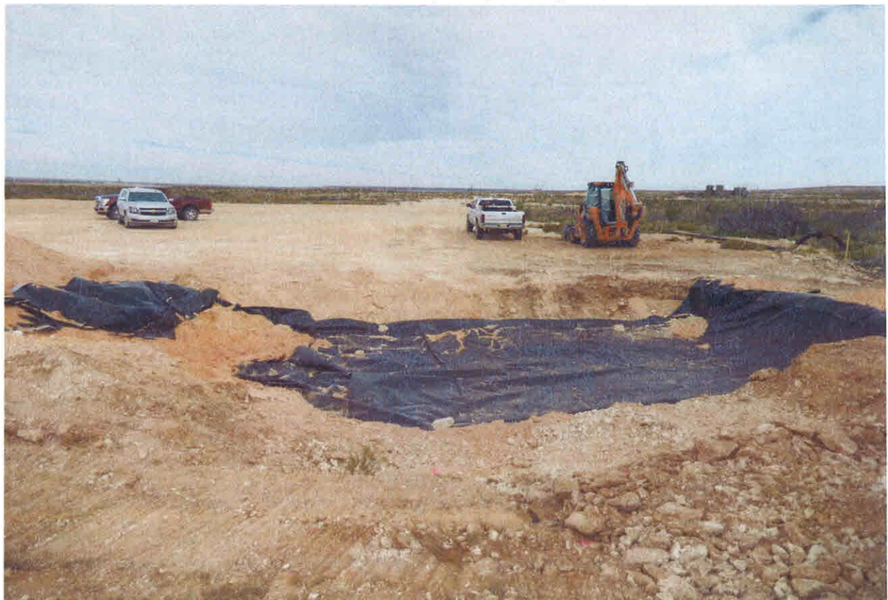
Liner Installed in Excavation DP-02-02 (4 feet) Viewing North, November 28, 2016
