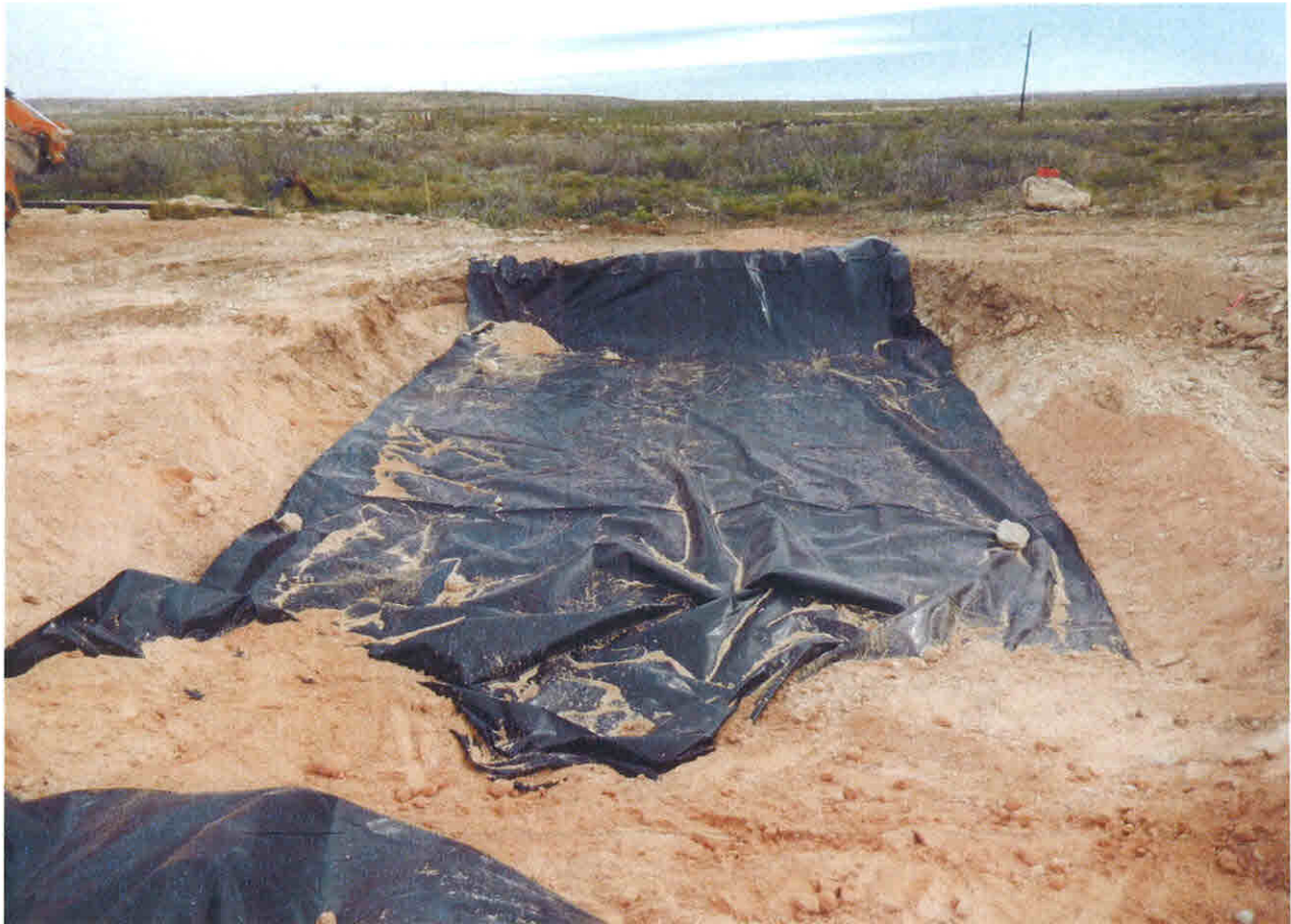
Liner Installed in Excavation DP-02-02 (4 feet) Viewing East, November 28, 2016
