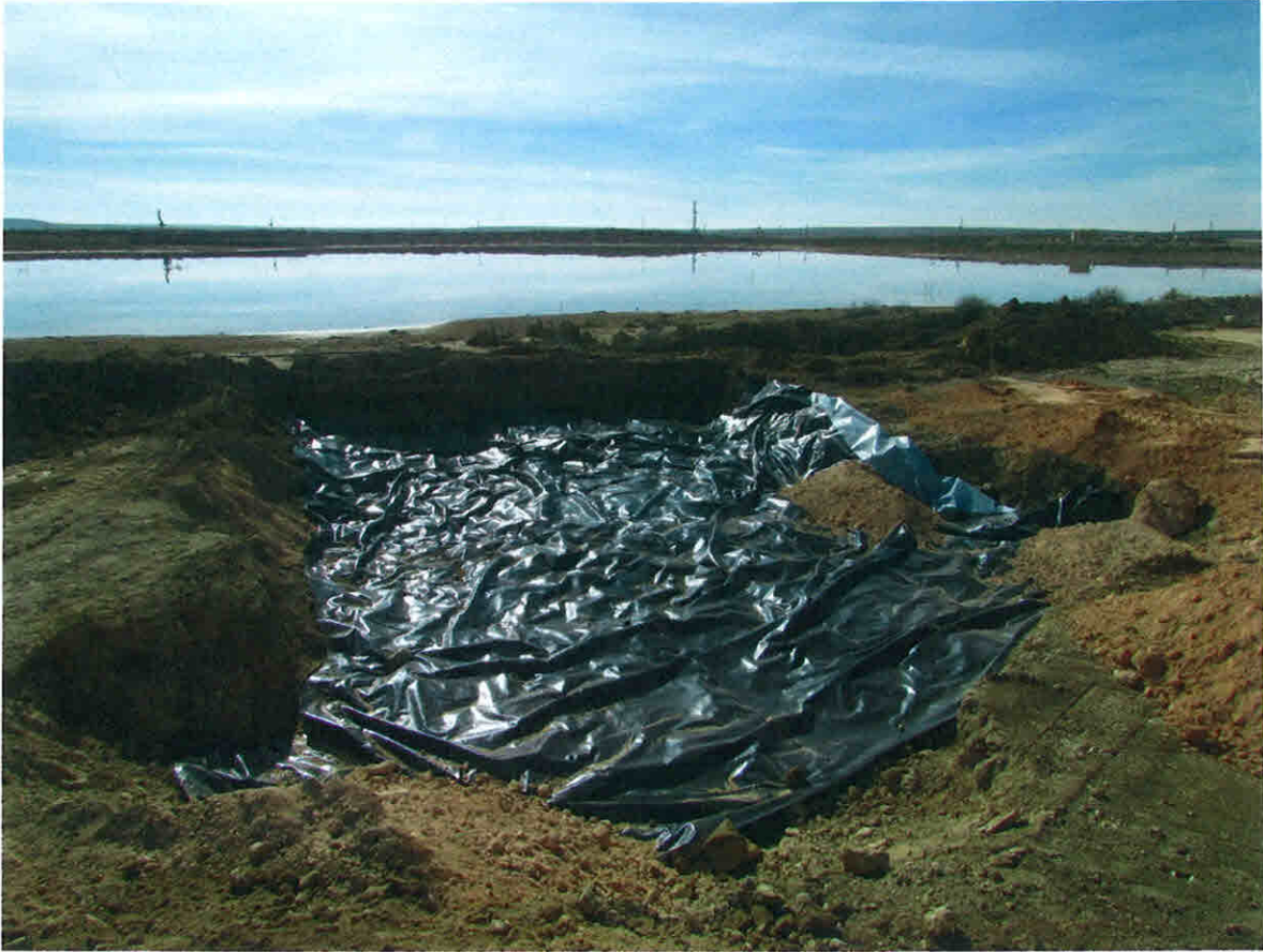
Liner Installed in Excavation (4 feet) Viewing South, December 15, 2016
