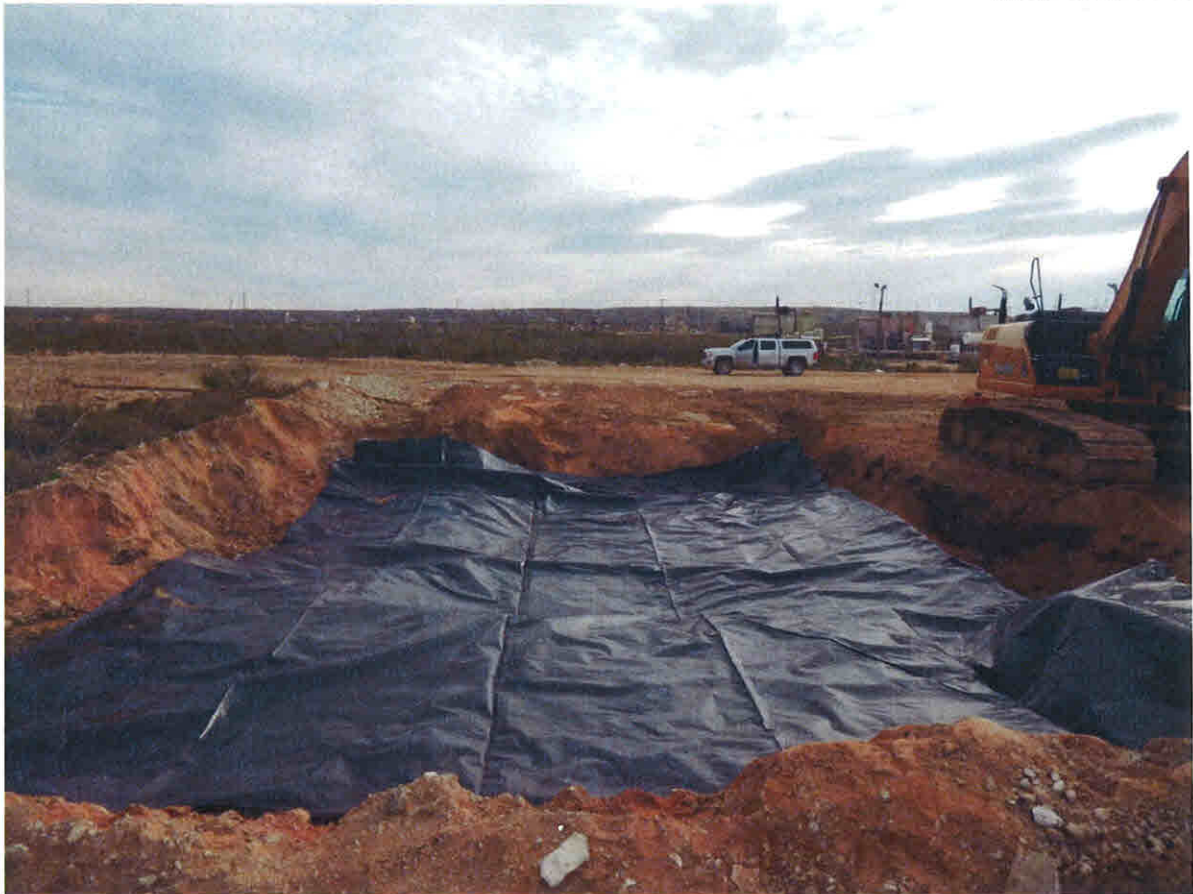
Liner Installed in Excavation (3 Feet) North of DP-01-04 Viewing East, December 6, 2016
