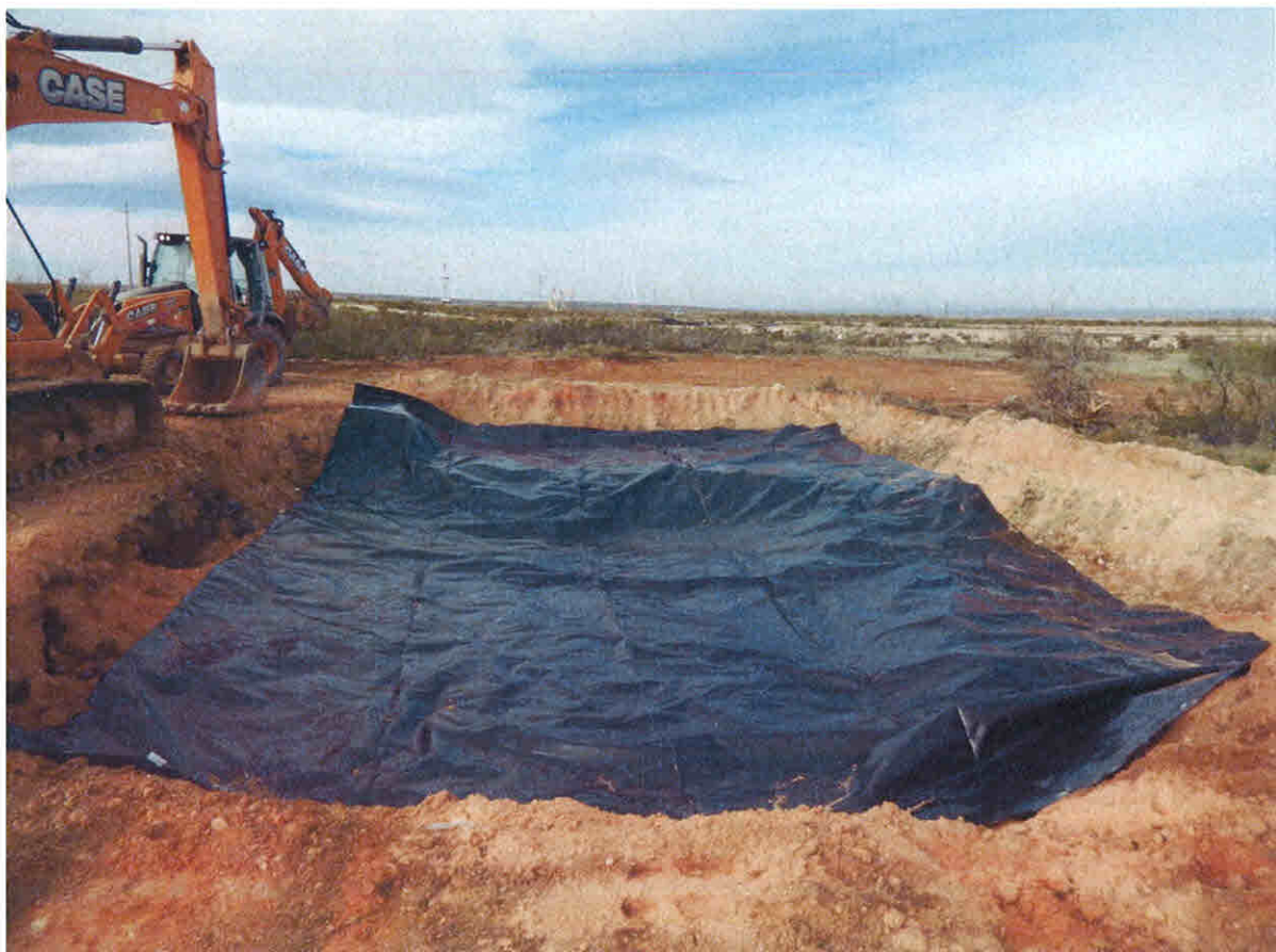
Liner Installed in Excavation (3 Feet) North of DP-01-04 Viewing West, December 6, 2016
