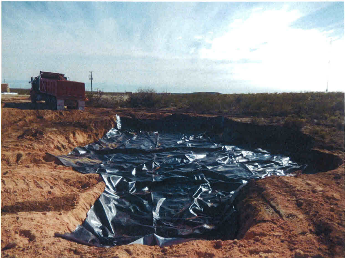
Liner Installed in Excavation (4 Feet) Viewing South, December 6, 2016
