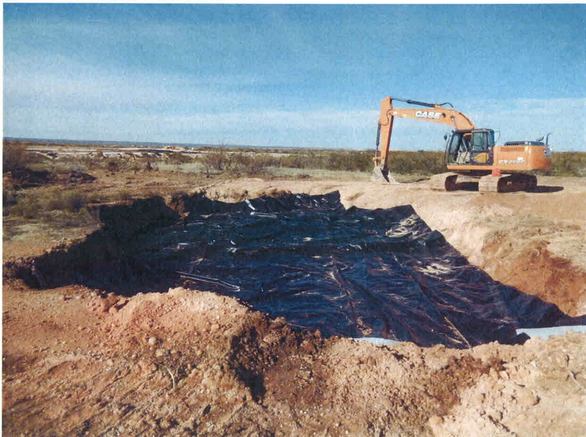
Liner Installed in Excavation (4 Feet) Viewing North, December 6, 2016
