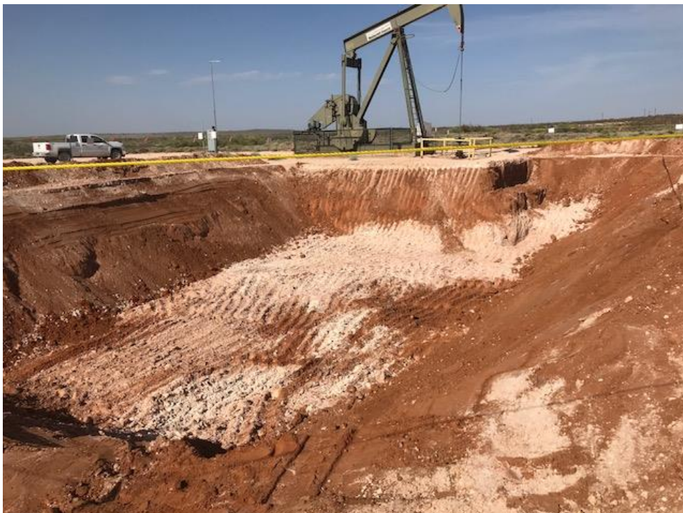
Photograph 1: View northeast of equipment and excavation.
