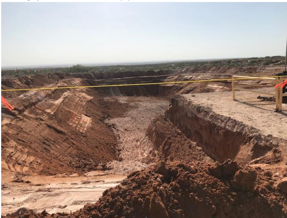
Photograph 2: View west of excavation.
