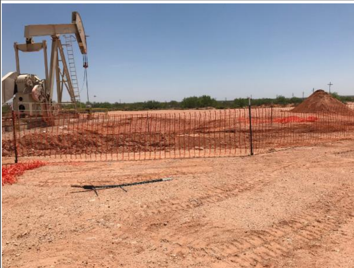
Southeastern view of final excavation extent.
