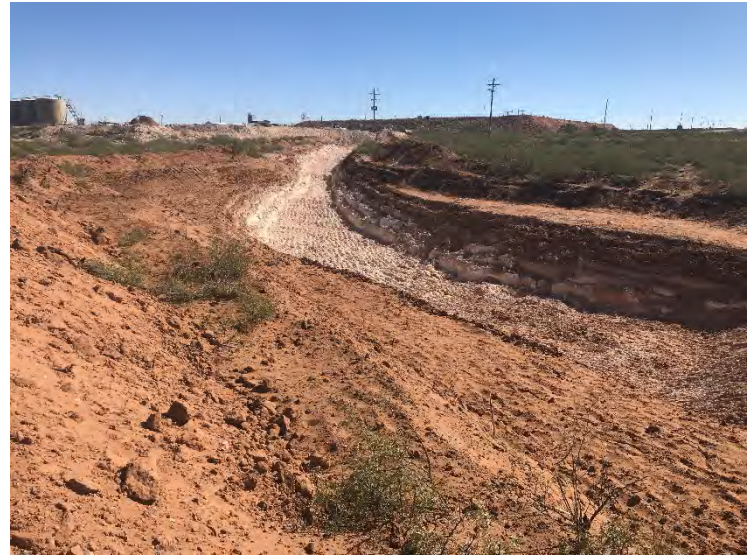
Photograph 6: Eastern view of the western end of the pasture excavation.
