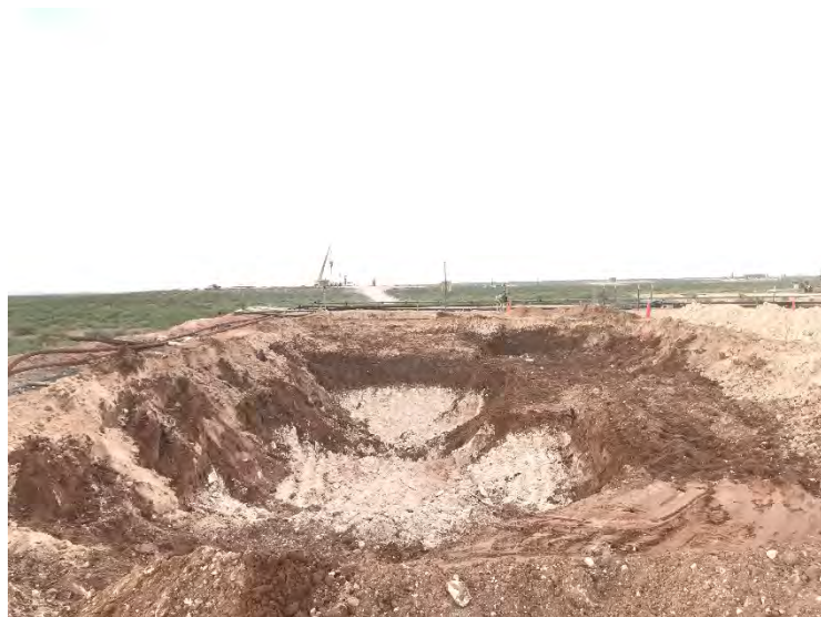
Photograph 3: Northern view of the on-pad excavation.
