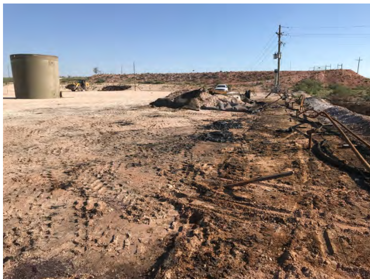
Photograph 1: Southern view of the release extent on pad.
