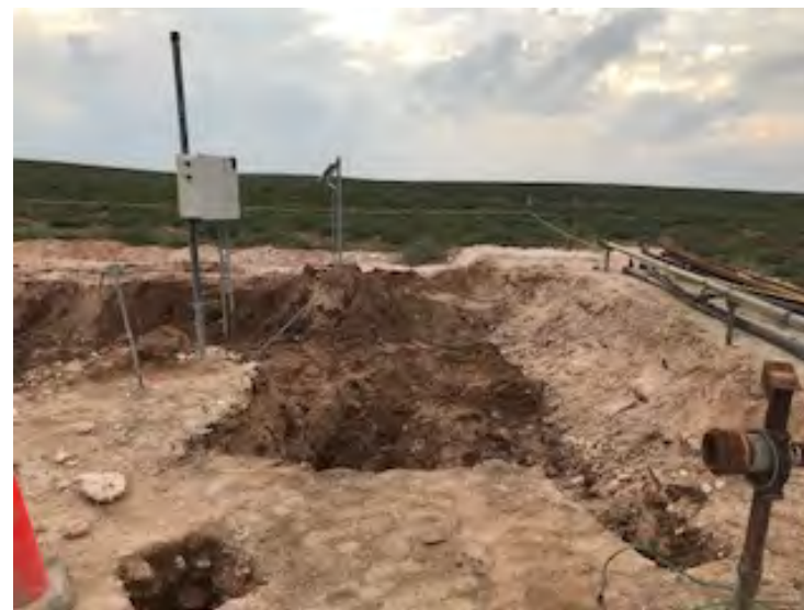
Photograph 4: View west of the on-pad excavation in the northern corner.
