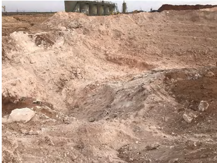
Photograph 5: View of the pasture excavation near the pad facing east.
