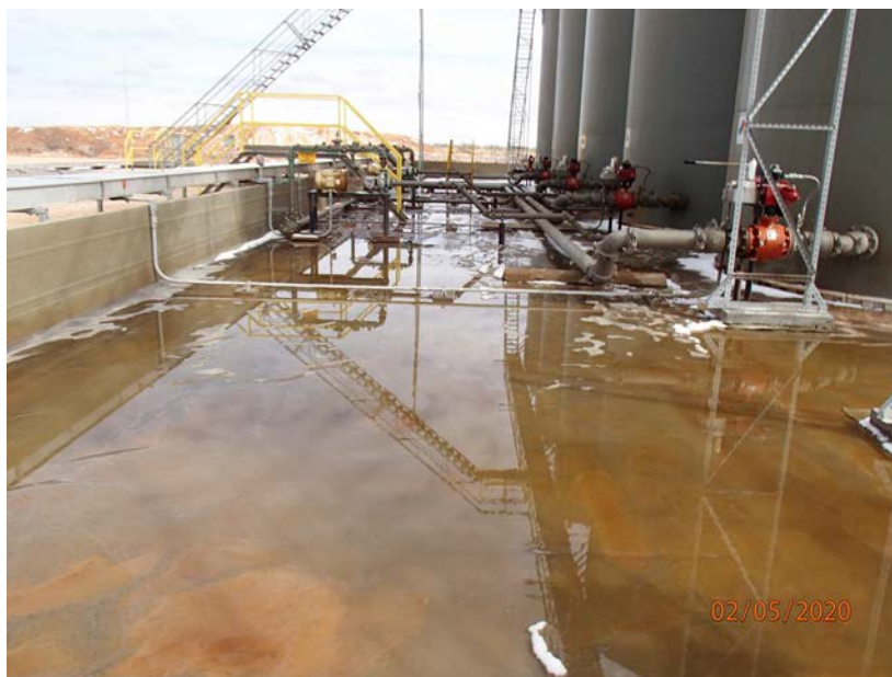
View of standing water cover the majority of the liner.
