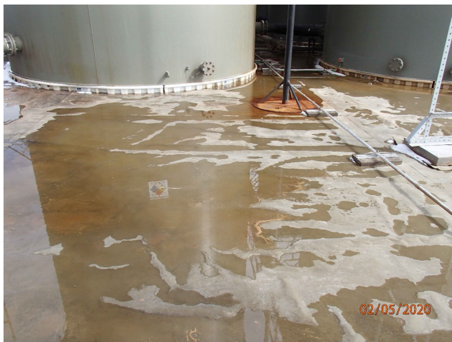
View of standing water within the liner.
