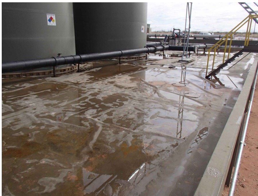
View showing standing water is prevalent within the liner.
