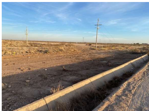
Photograph 5: View of eastern excavation along roadside facing southeast.
