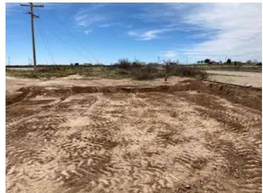
Photograph 10: View of area west of main road after further excavation.
