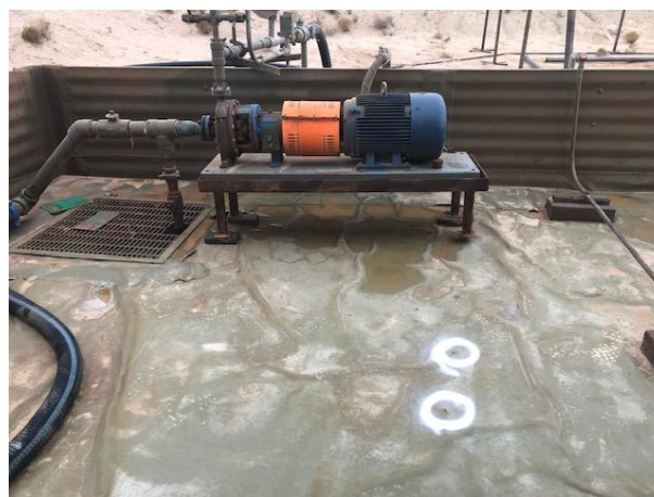
Photograph 2: View of liner tears at BH04 and BH05 sample locations.
