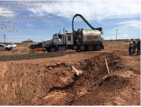
Photo 3. South view of western end of excavation to remove damaged pipeline.
