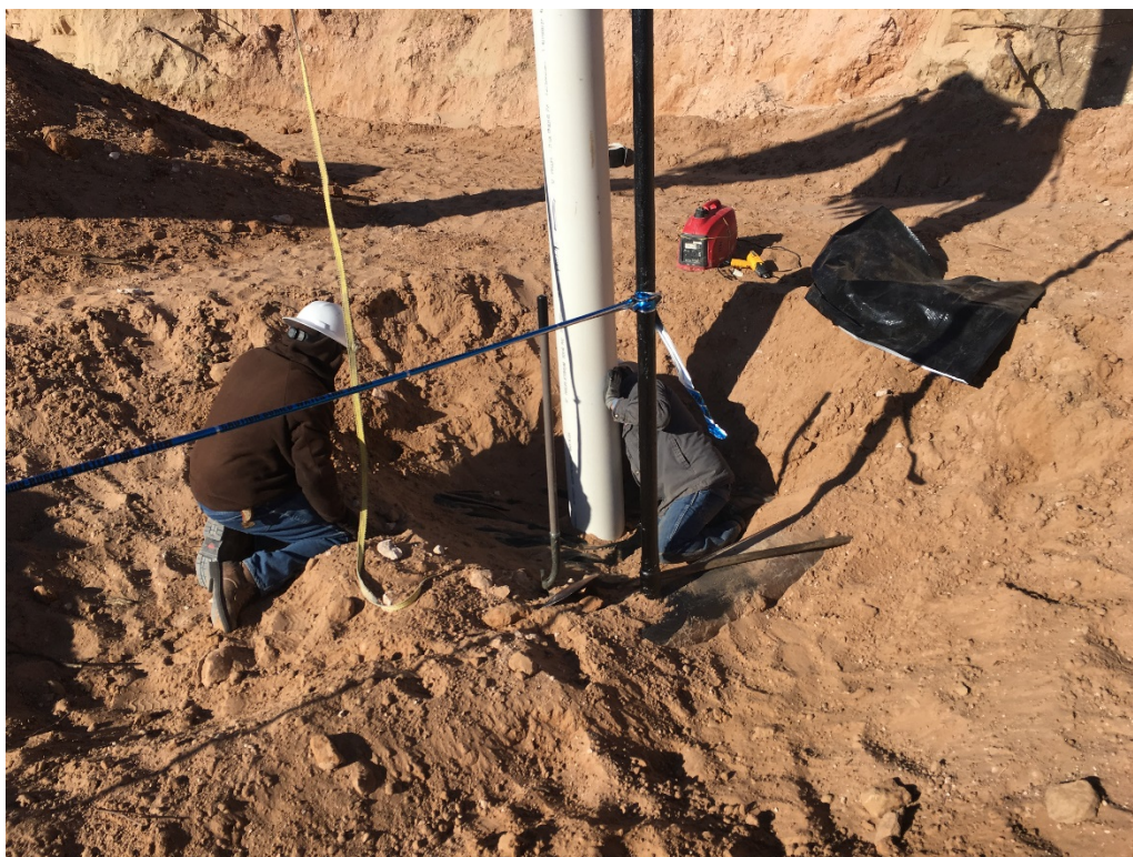
Photo of Installing 10" Casing for BH 1
