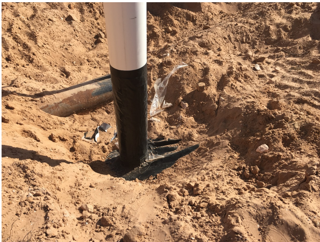
Photo of 10" Casing Complete With Liner
