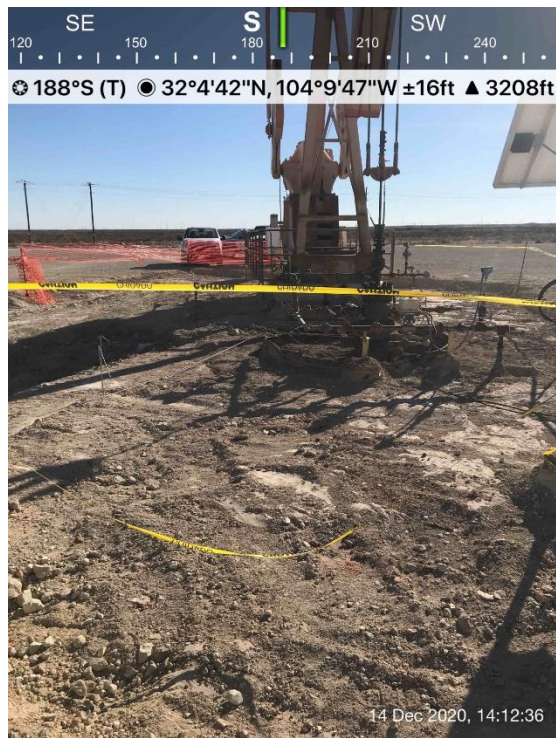
Excavated soil viewing south, December 14, 2020
