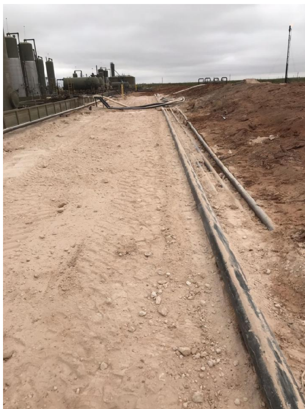
Photo of Backfilled area
