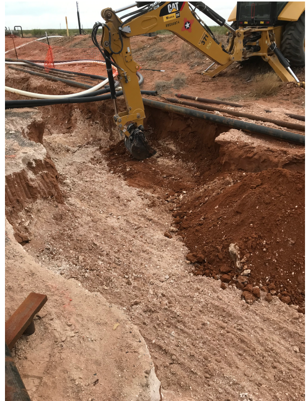
Photo of Excavation
