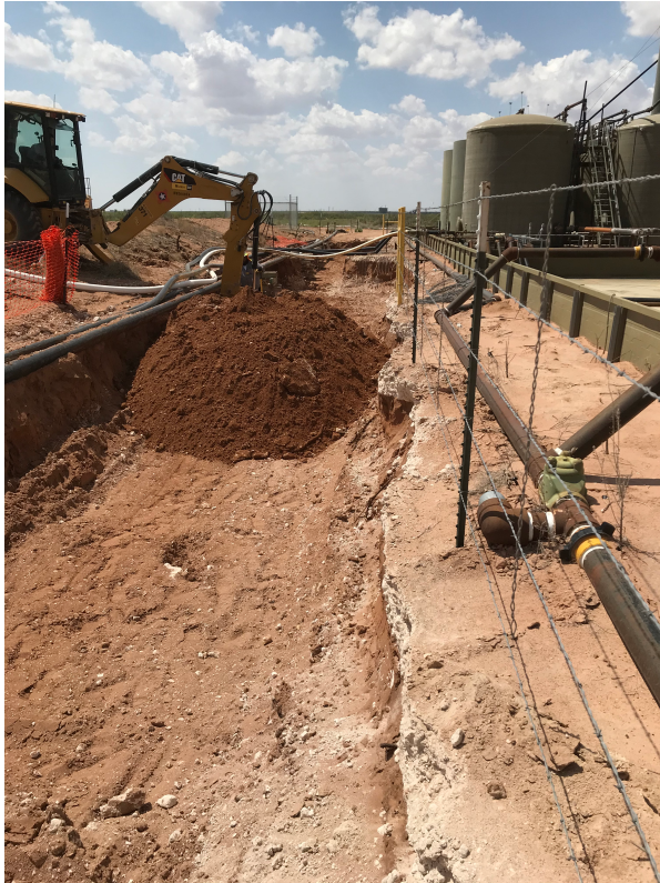
Photo of Excavation
