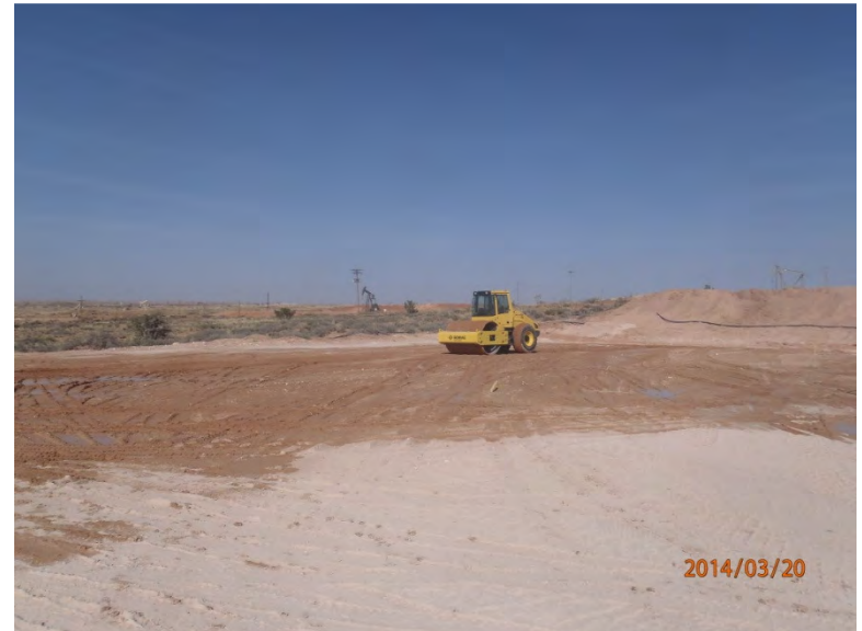
Packing backfilled area, facing northeast 3/20/14
