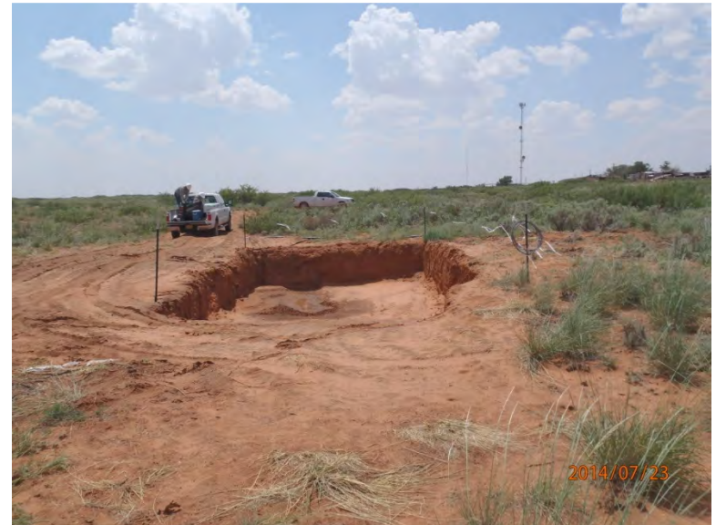
Excavation to 4 ft bgs completed, facing west 7/23/14
