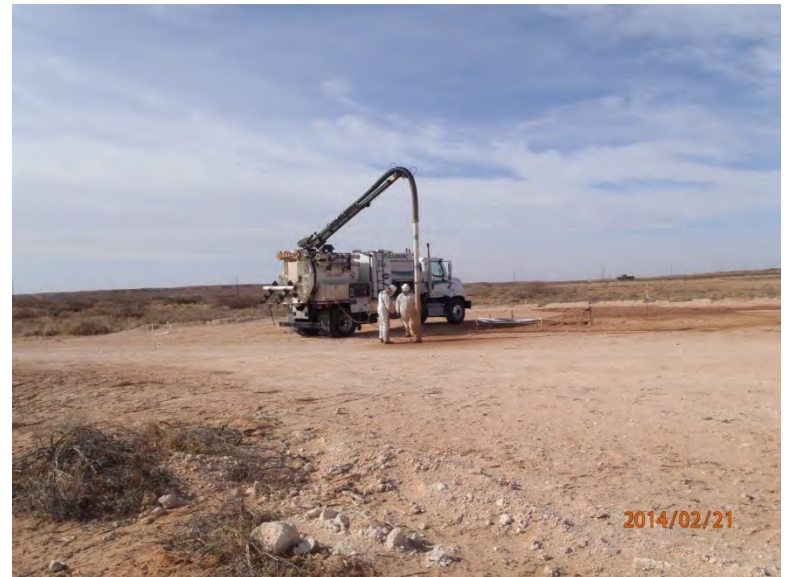
Line spot using a hydrovac, facing southwest 2/21/14
