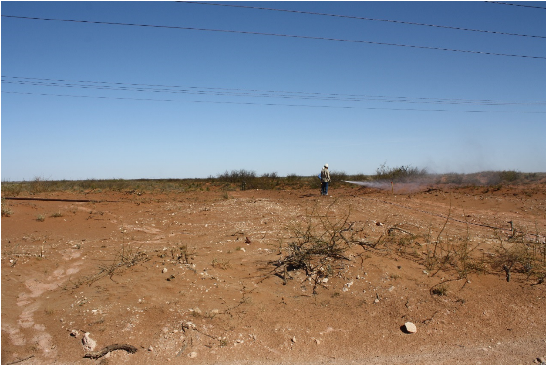
Photograph of the application of soap and Micro-Blaze® to the affected area at the PLU #411 Tank Battery Flare Release Site.
