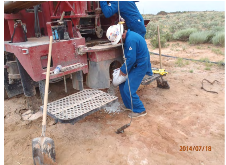
Plugging SB-1 in total with bentonite, facing west 7/18/14
