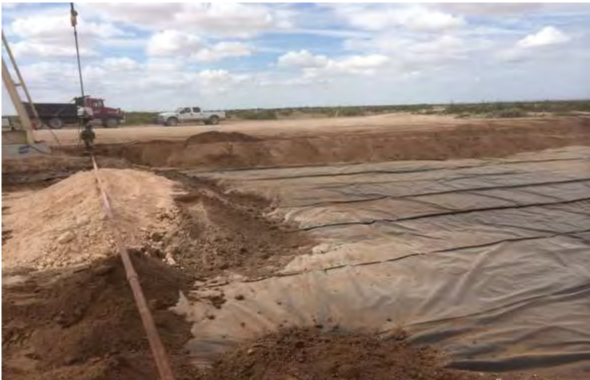
Bass 3 Federal #4 – Liner Installation (Looking South-Southwest)
