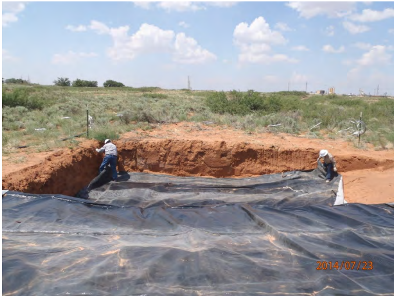
Installing liner, facing north
