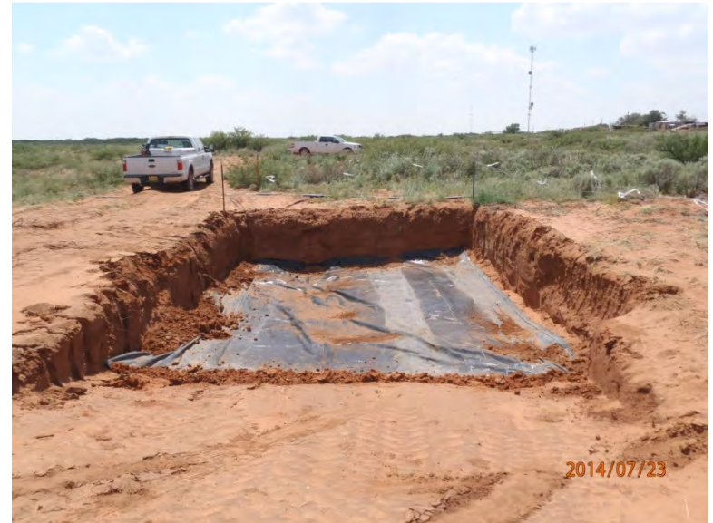
Liner installation completed, facing west
