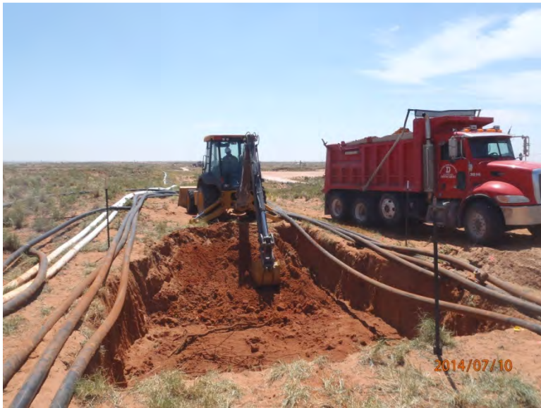
Continue to excavate to 4 ft bgs by backhoe, facing east 7/10/14
