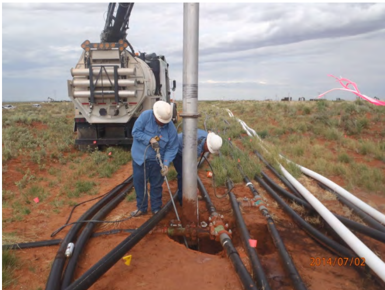
Line spotting with hydrovac, facing west
