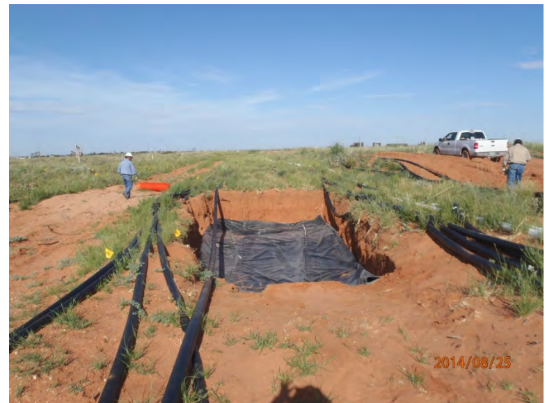
Liner installed, facing west 8/25/14
