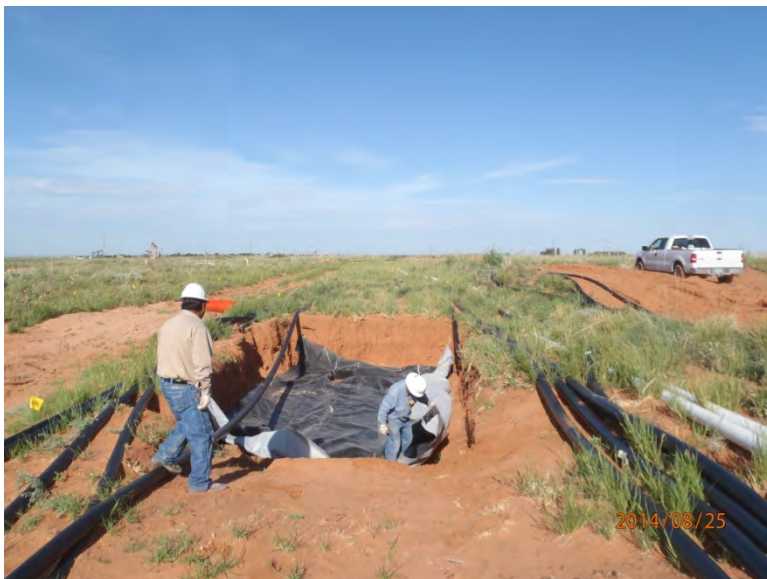
Installing liner, facing west 8/25/14
