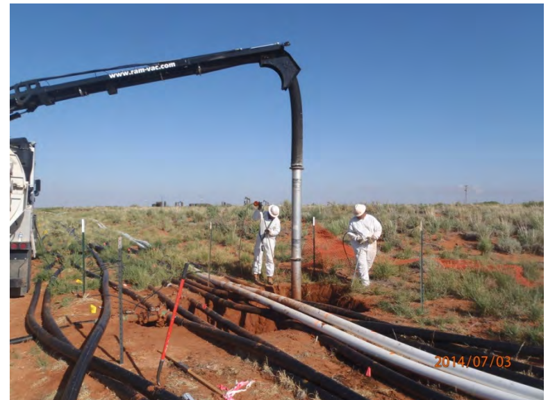
Excavating by hydrovac to 4 ft bgs, facing west
