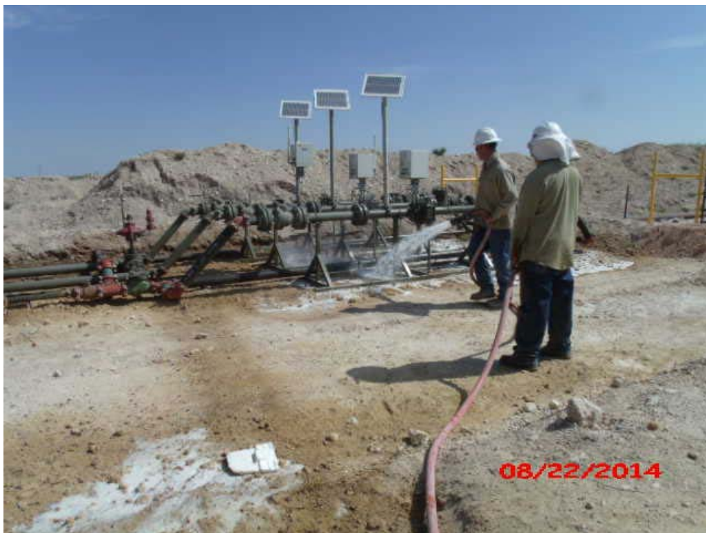
Photograph #13 – Application of Micro-Blaze
